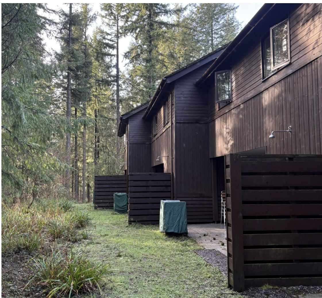
Figure 4: Rear of Existing Lodges, Patio/BBQ Areas.
