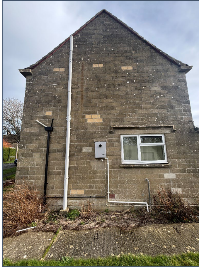
Photo of west gable; Proposed extension extends from this elevation.
