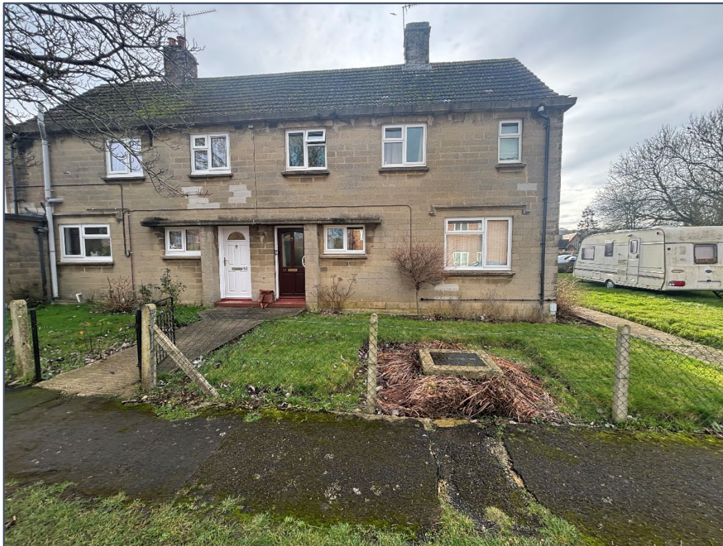
Photo of front (principal) elevation. Proposed extension is to the gable to the right of the photo.
