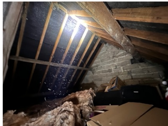
Photograph 13: Internal view of the roof space.
