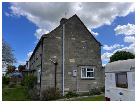
Photograph 2: West elevation of the building.
