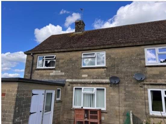
Photograph 3: South elevation of the building.
