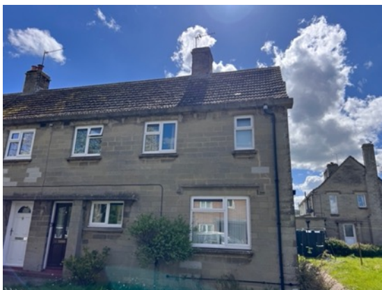
Photograph 1: North elevation of the building.
