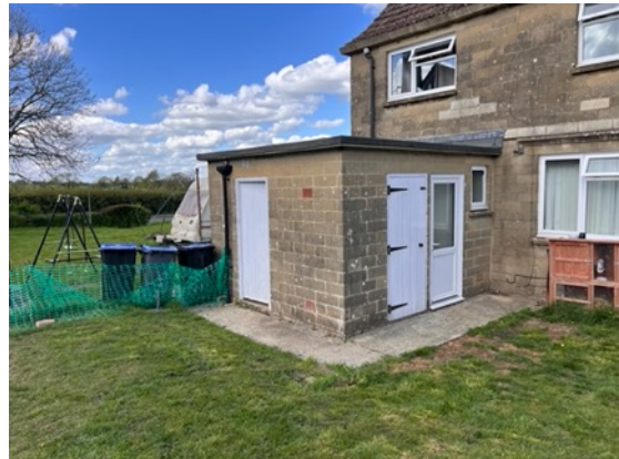
Photograph 4: Flat roof single storey section.
