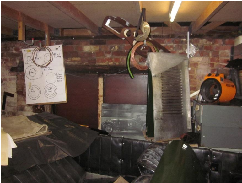
Historic west wall
