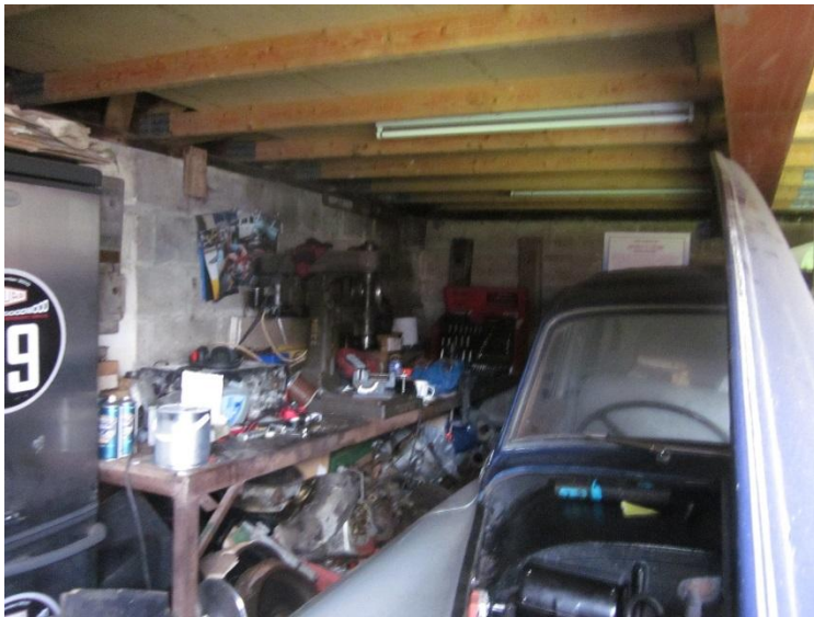
'Modern' blockwork walls and trussed rafters
