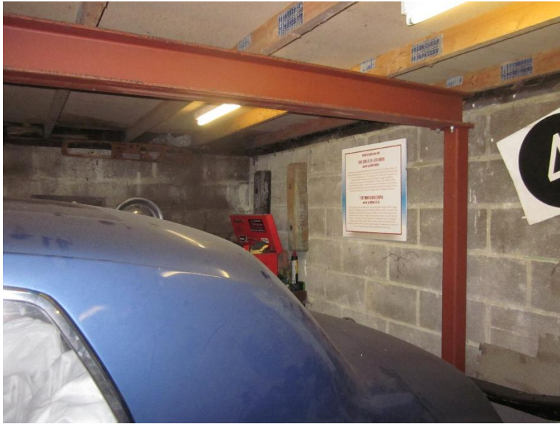
Steel frame re-inforcing/ supporting south wall / roof
