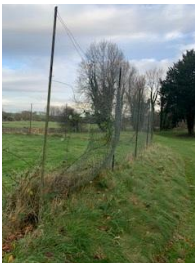
Figure 5 - Detail of poor state of previous fencing
