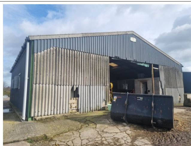
Photograph 3. The front south western elevation.
