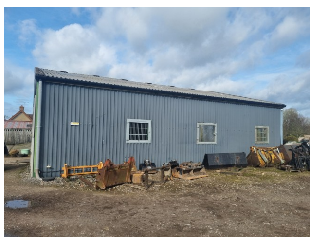
Photograph 2. Steel corrugated panels.
