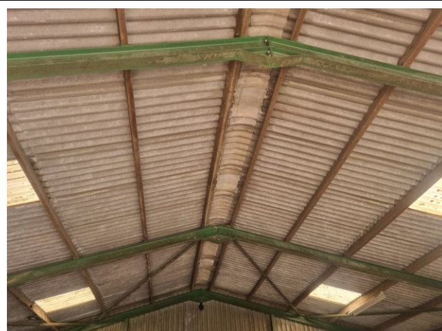
Photograph 9. The building had no internal roof void.
