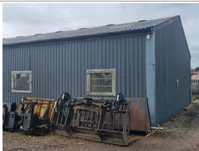
Photograph 6. Windows on the south east elevation.
