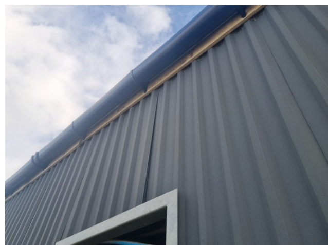
Photograph 5. Wooden fascia supporting the guttering.
