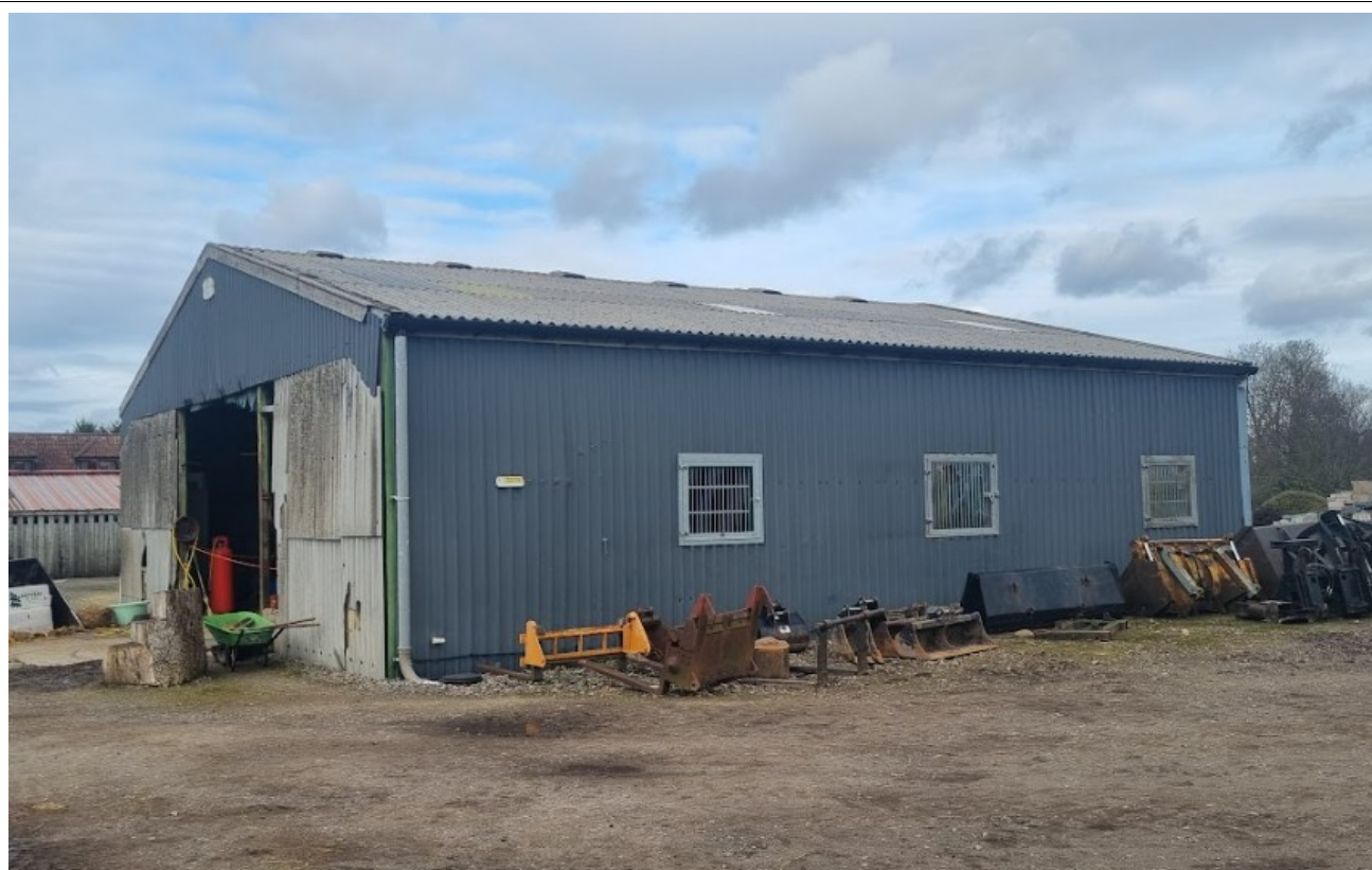
Photograph 1. The agricultural building subject to survey, viewed looking north.
