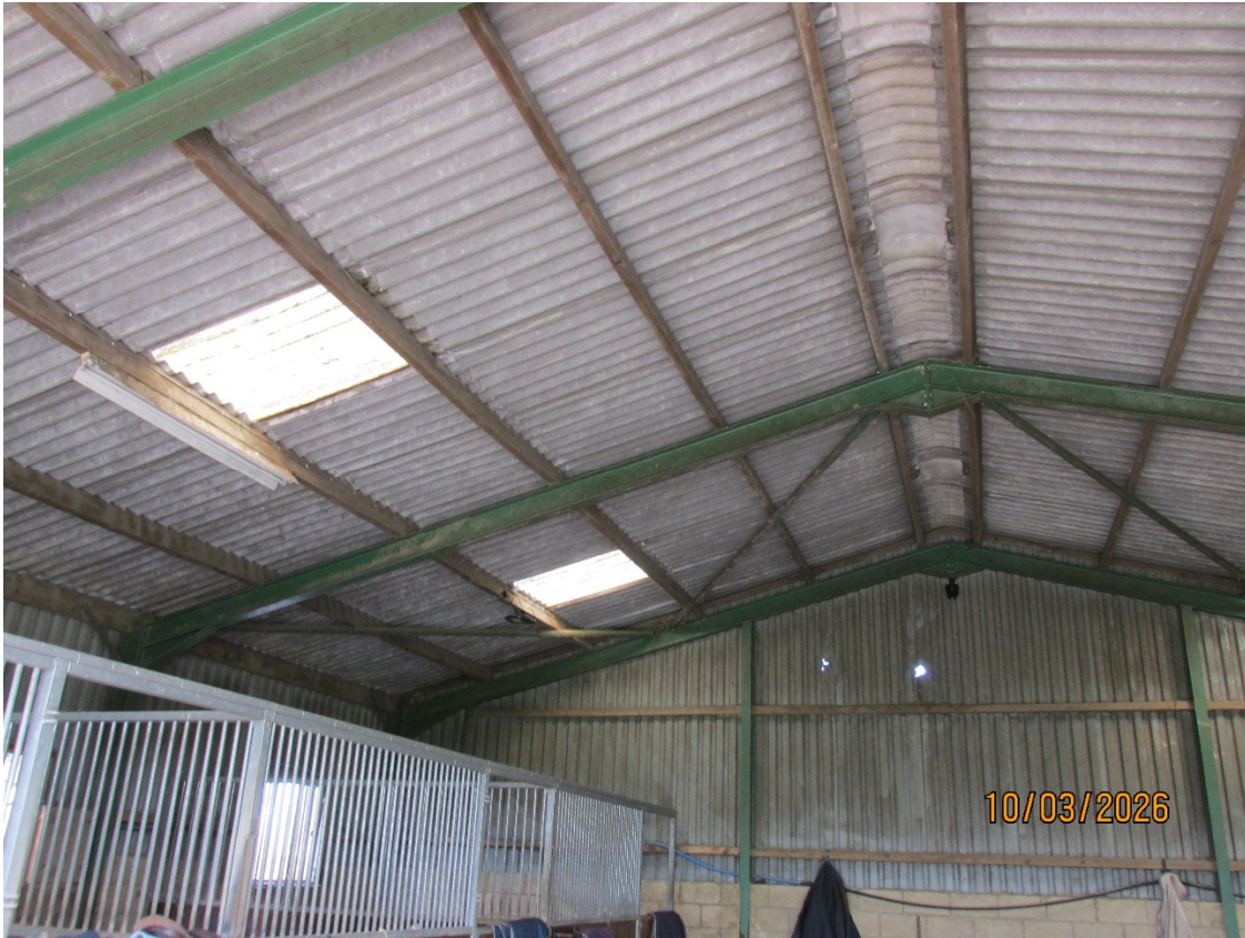
Internal view showing structural steel portal frame, roof & wall cladding
