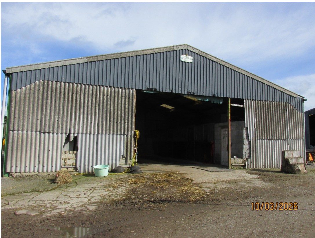
External south west elevation
