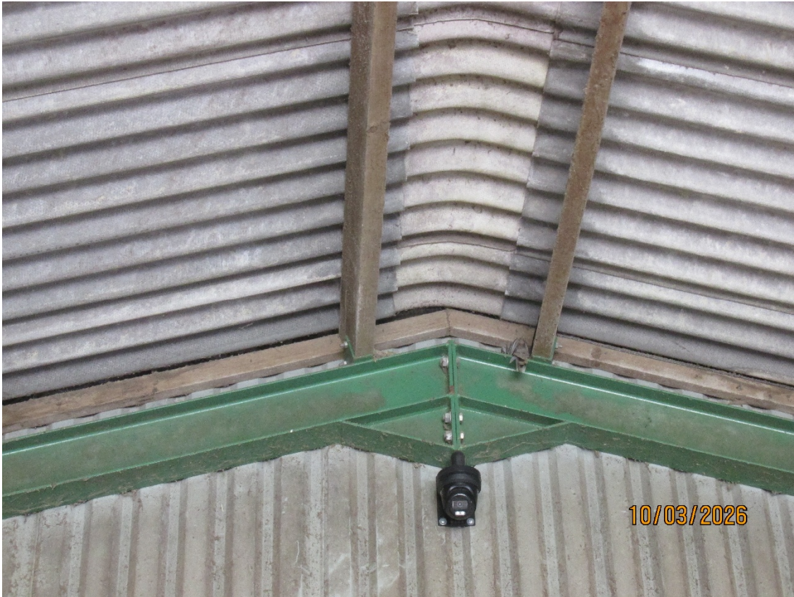
View of Haunch Connection at Ridge
