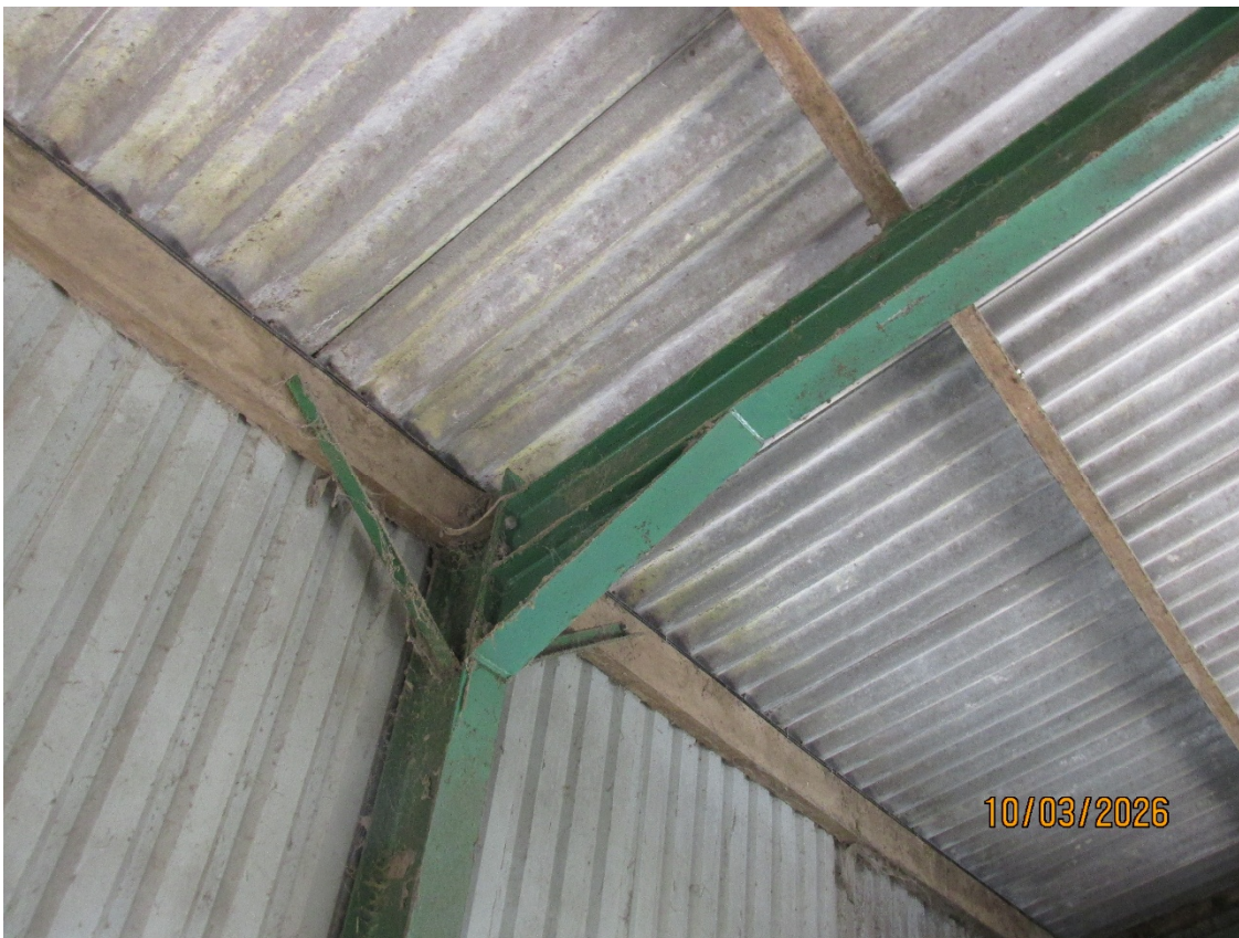
View of Haunch Connection between portal frame post & principal rafter
