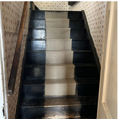
GF007 Staircase wall
