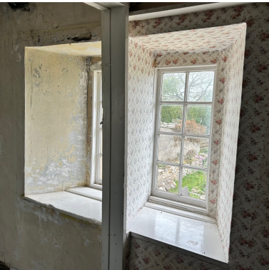
FF009 – Window with partition
