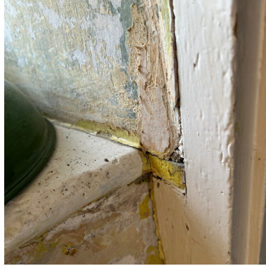
FF009 – Window cill remain intact.
