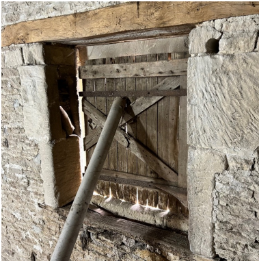
IMG008 – Opening in barn. On mezzanine
