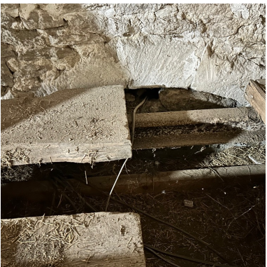
GF – View from mezzanine – stone archway
