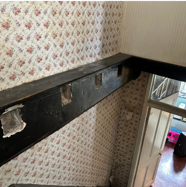
FF005 – Showing beams cut for opening
