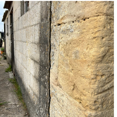
GF011 – Stables cement abutment to 1740'S barn
