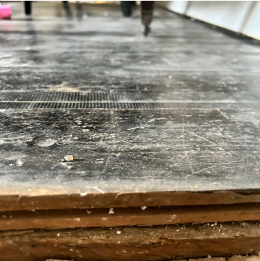
FF02 – Showing edge on view of floor
