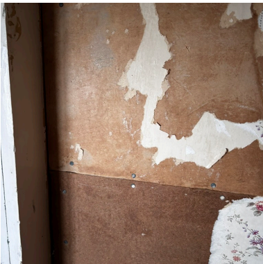
IMG015 – Hardboard partition
