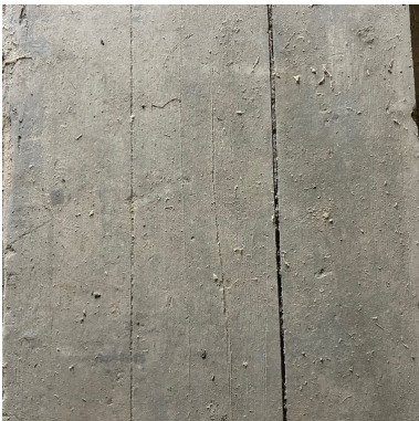
IMG012 – Mezzanine boards
