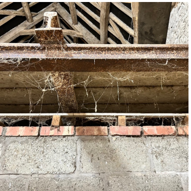
GF – Concrete blockwork and railway line mezzanine.
