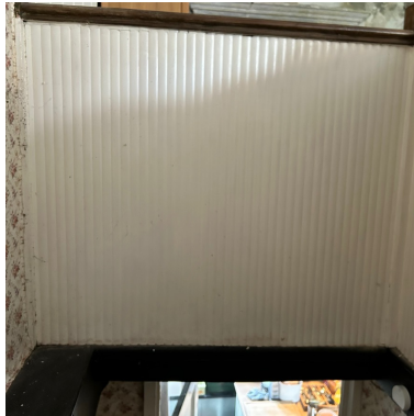
FF005 – Mid century stair balustrade
