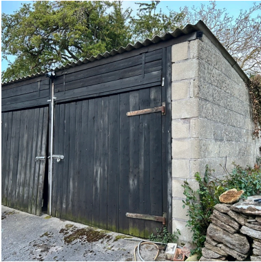
IMG002 – Existing shed
