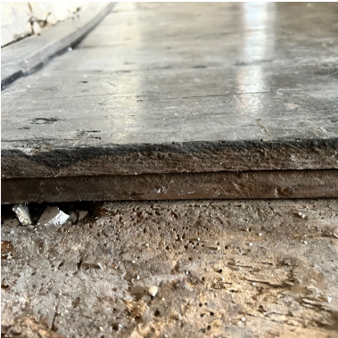
FF004 – Floor section showing newer floor laid on 16 th century boards
