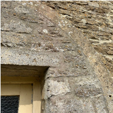
IMG006 – Stone archway with concrete / stone infill
