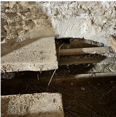
IMG010 – Archway from mezzanine
