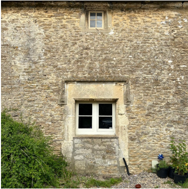
IMG001 – Front doorway infill
