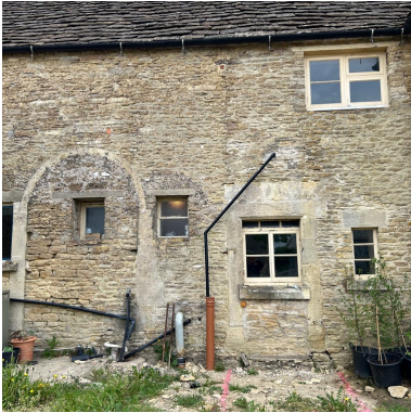
IMG004 – rear elevation / 20 th century opening and infill
