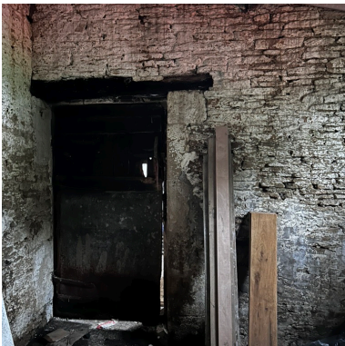
IMG014 – Side to door to Barn concrete stable
