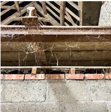
IMG009 – Mezzanine – concrete blockwork
