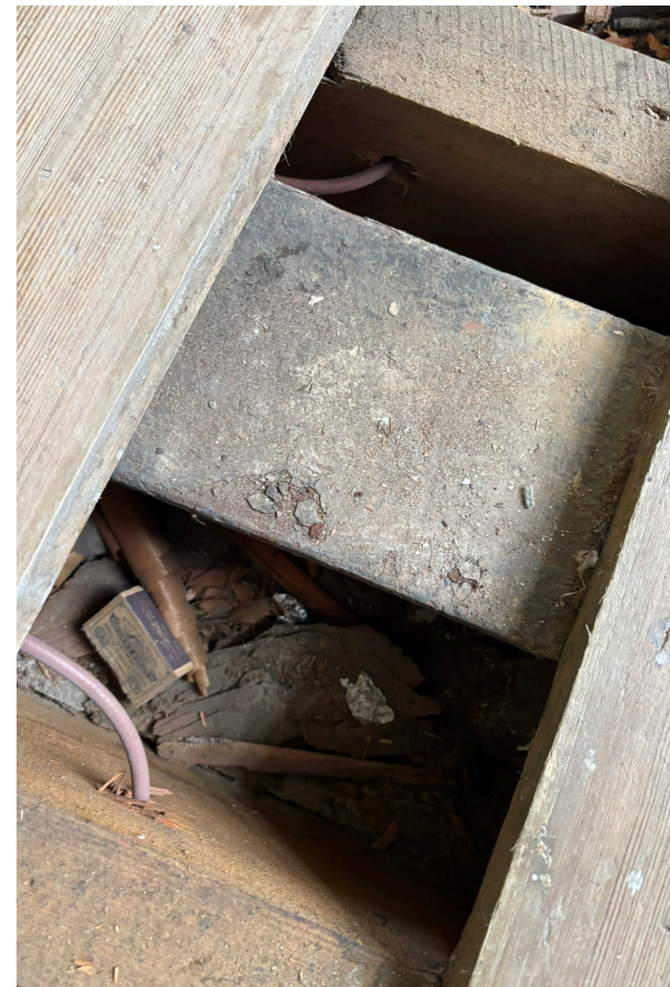
Steel beam (First Floor)
