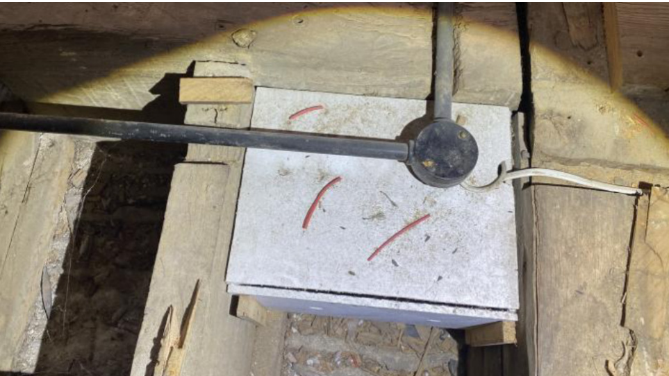
Lining panels containing asbestos used for boxing
