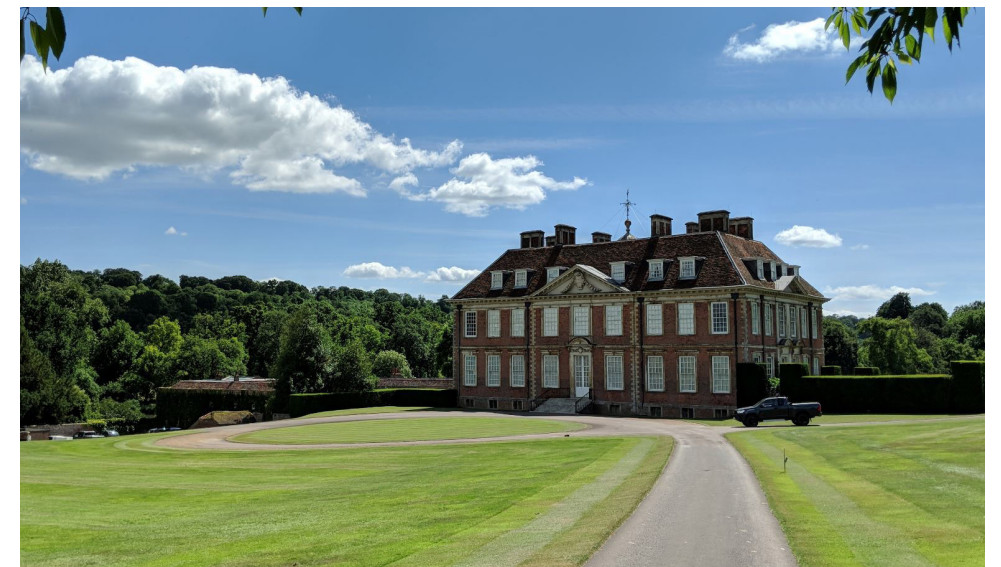
Current view of the north elevation of Ramsbury Manor, 2019
