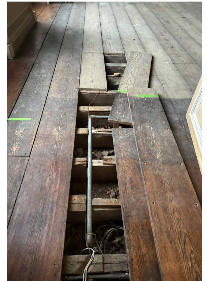
Furrings to level out floor (Ground Floor)
