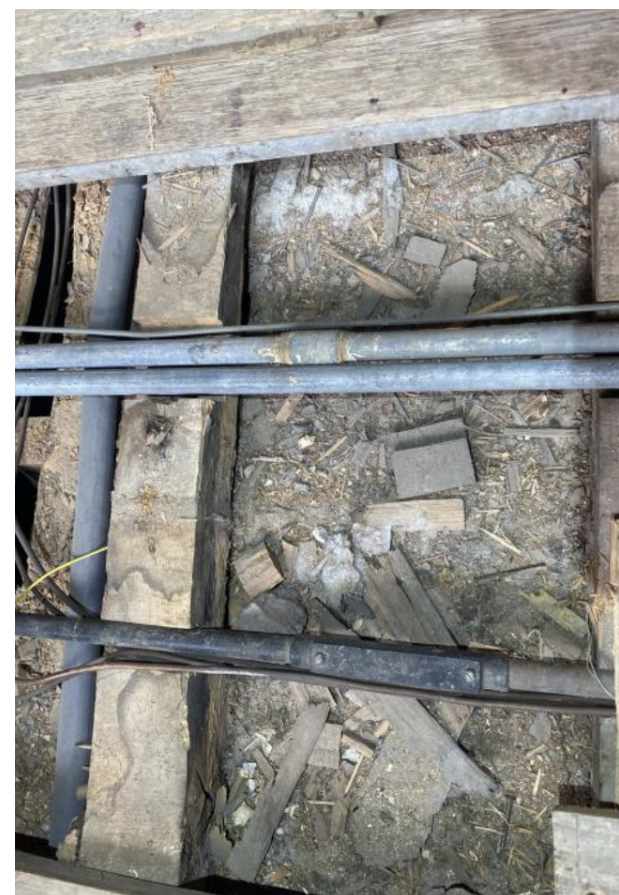
Concealed dropped ceiling void below the ceiling void (First Floor)
