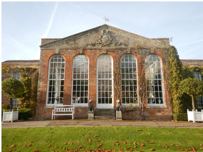
3. Orangery-part of Courtyard Buildings (curtilage listed)
