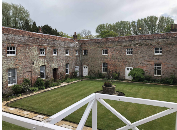
2. Courtyard Buildings (curtilage listed)
