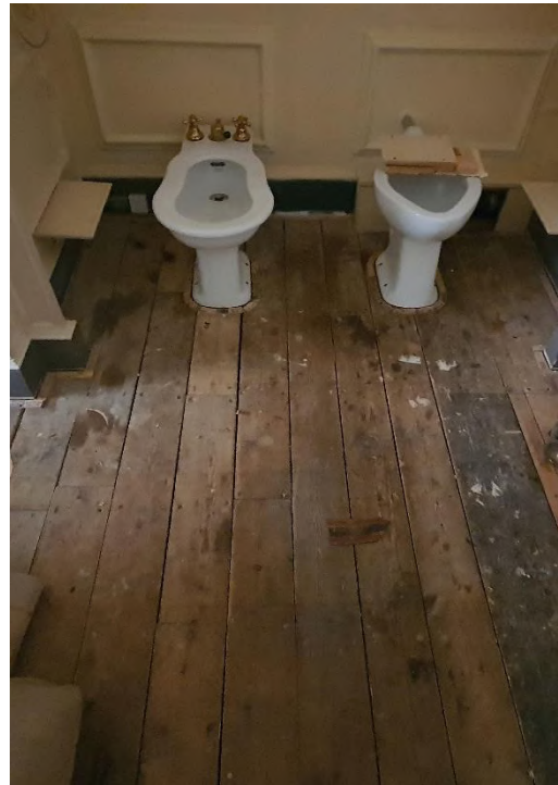
Figure 69: Timber boards, post vinyl removal- Mrs. Hyams Bathroom FR10
