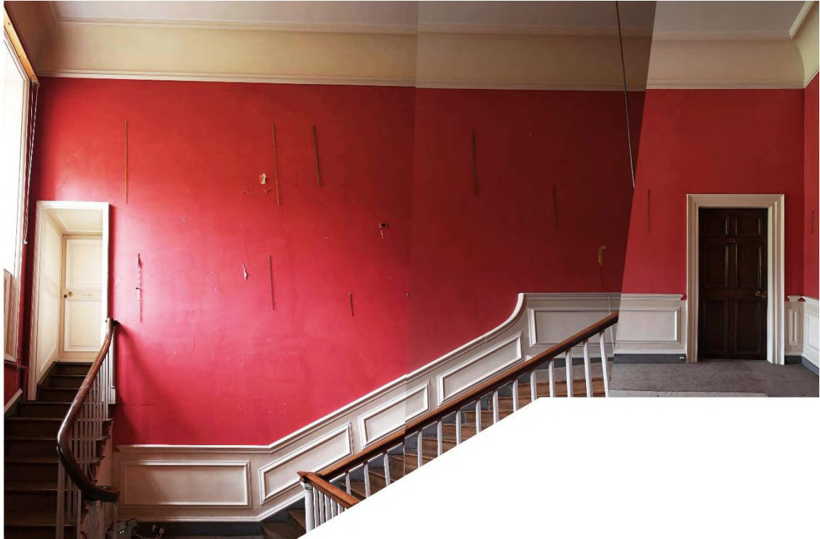
Figure 62: NE internal facade - First Floor - North Hall ST02
