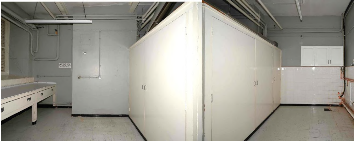
Figure 47: NE internal facade - Laundry Room LGR13
