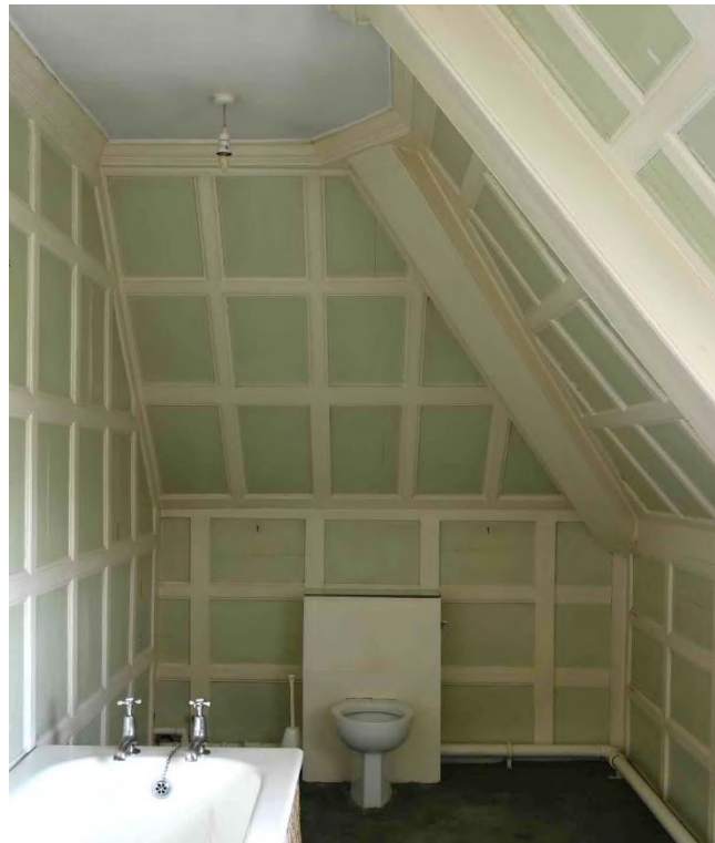
Figure 37: NE internal facade - Bathroom SR07
