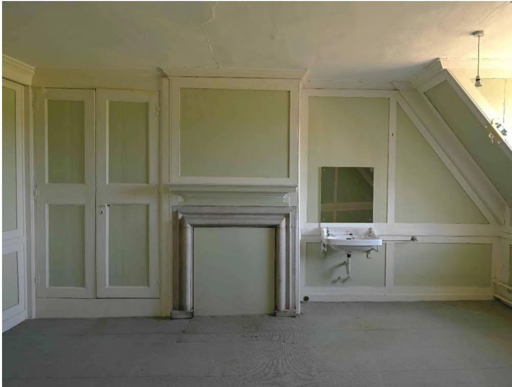
Figure 60: SE internal facade - Storeroom SR11
