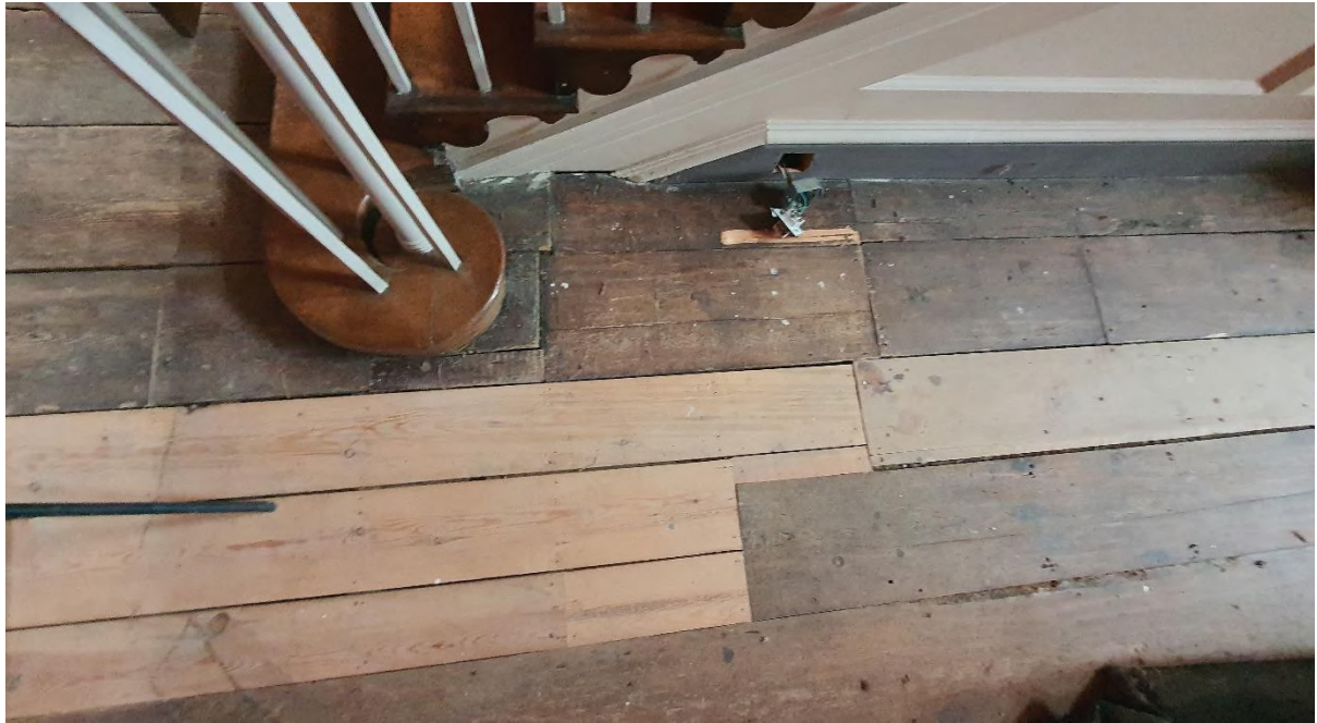
Figure 64: Floorboards - Ground Floor - North Hall ST02
