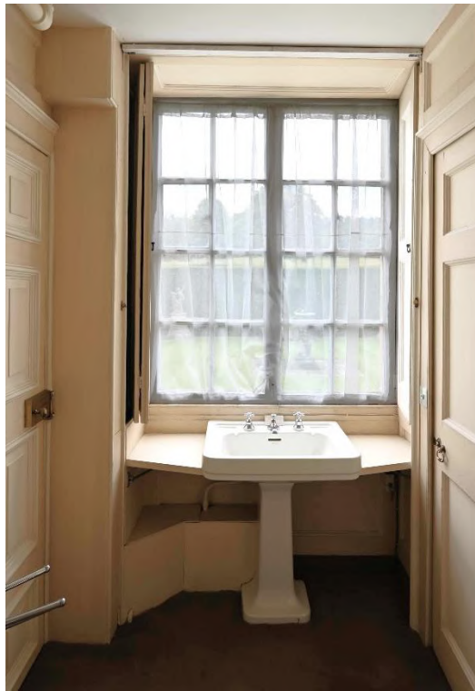
Figure 54: NW internal facade - North Hall Toilet GR09
