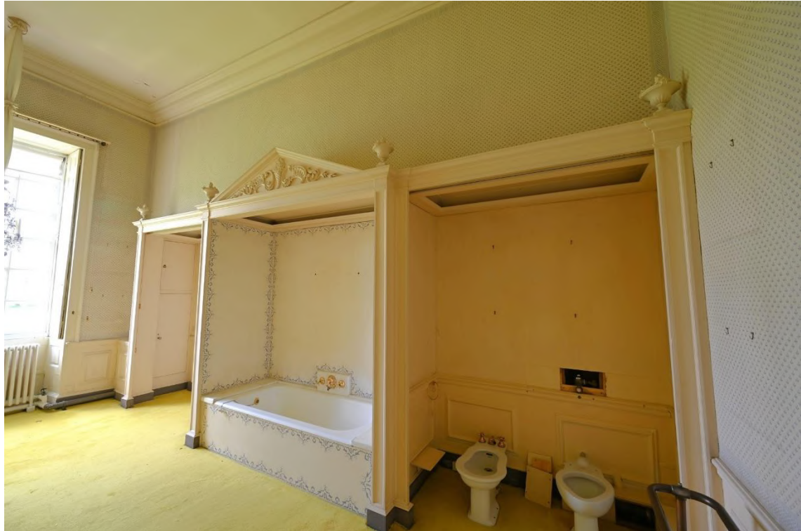
Figure 66: NW internal facade - Mrs. Hyams Bathroom FR10
