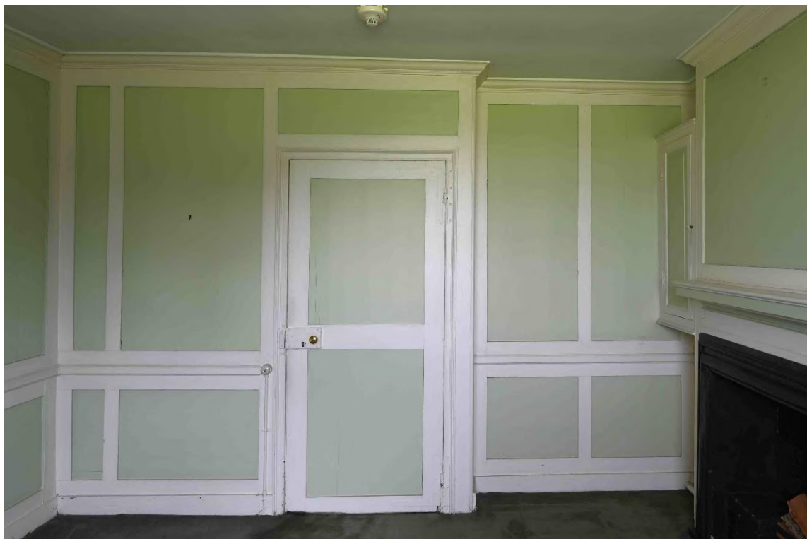
Figure 23: SW internal facade - Bedroom SR05
