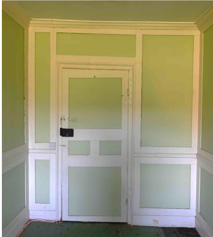
Figure 89: SE internal facade - Staff Bathroom SR17
