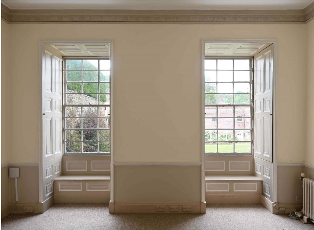
Figure 7: SE internal facade - Staff Room LGR05
