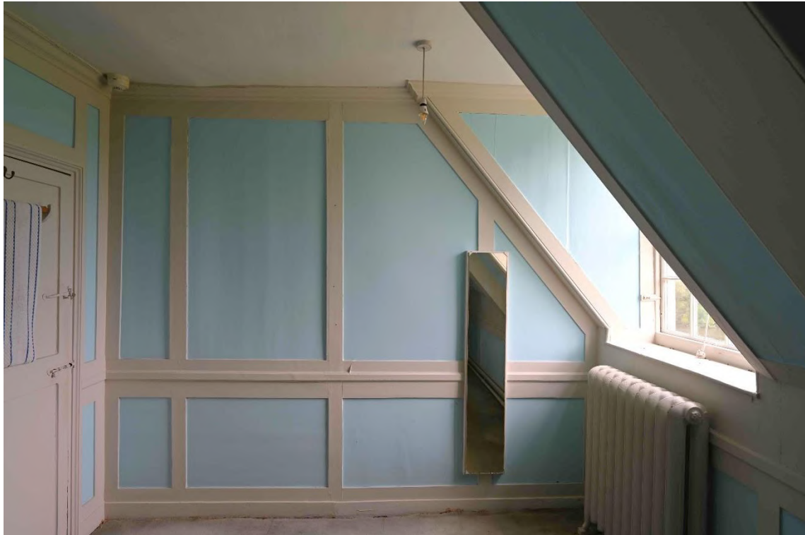
Figure 75: SE internal facade - Staff Bathroom SR14
