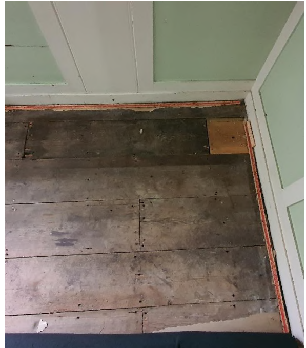
Figure 73: Timber floorboards exposed post removal of carpet - Sewing Room SR13
