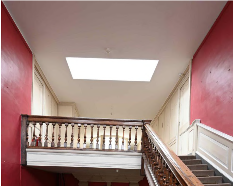
Figure 58: NW internal facade - Second Floor - Back Stairs ST01
