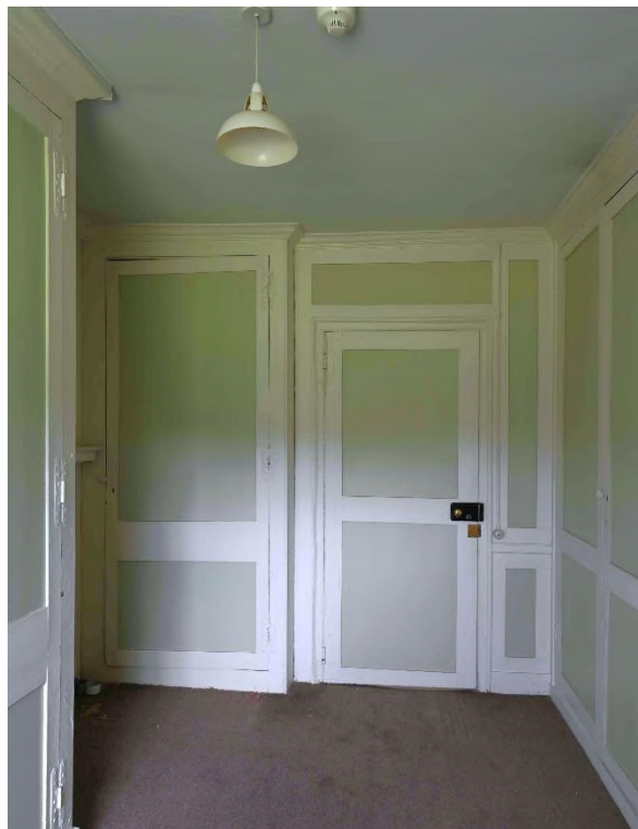
Figure 51: NE internal facade - Linen Room SR09
