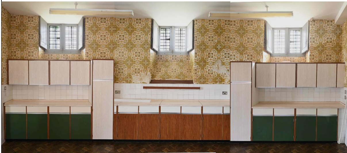
Figure 16: SW internal facade - Main Kitchen LGR07
