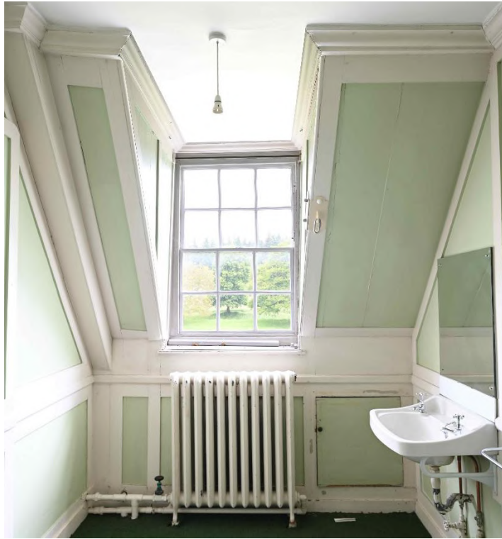
Figure 86: NW internal facade - Staff Bathroom SR16
