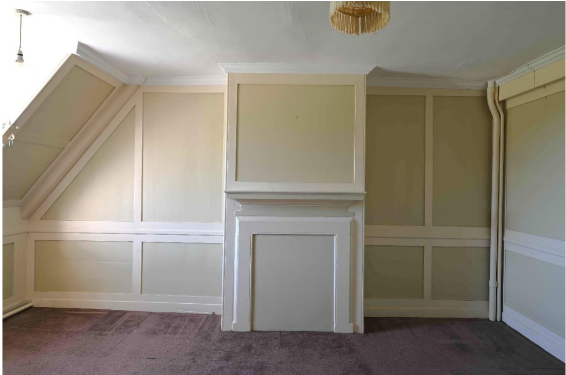
Figure 17: SE internal facade - Bedroom SR04
