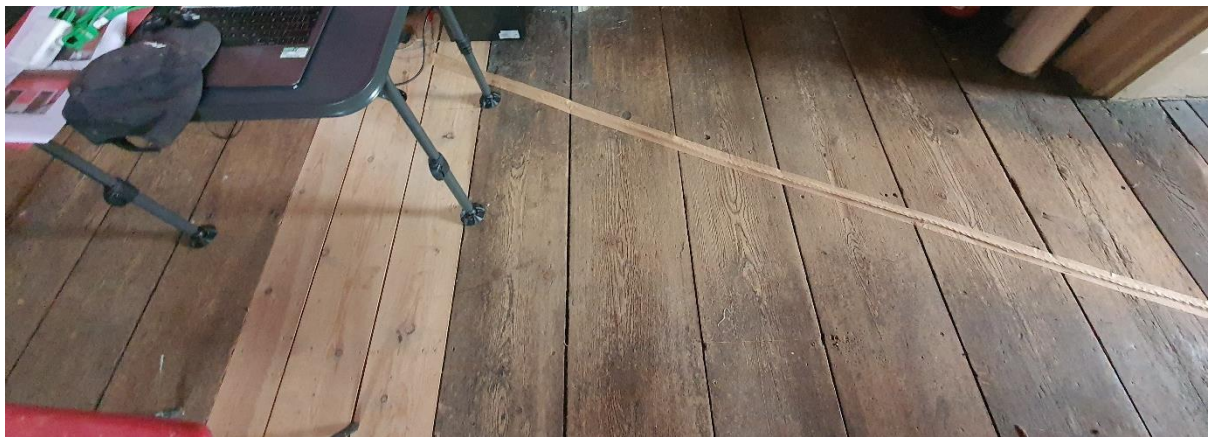
Figure 65: Floorboards - Ground Floor - North Hall ST02
