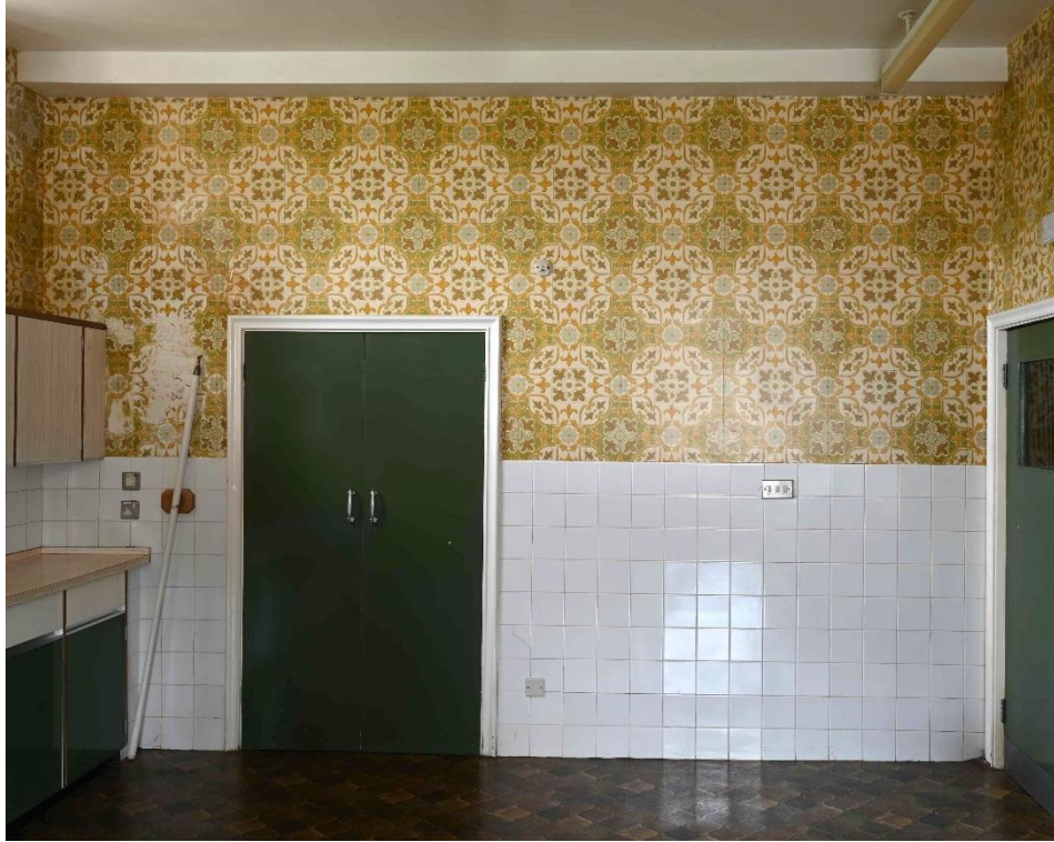
Figure 17: NW internal facade - Main Kitchen LGR07
