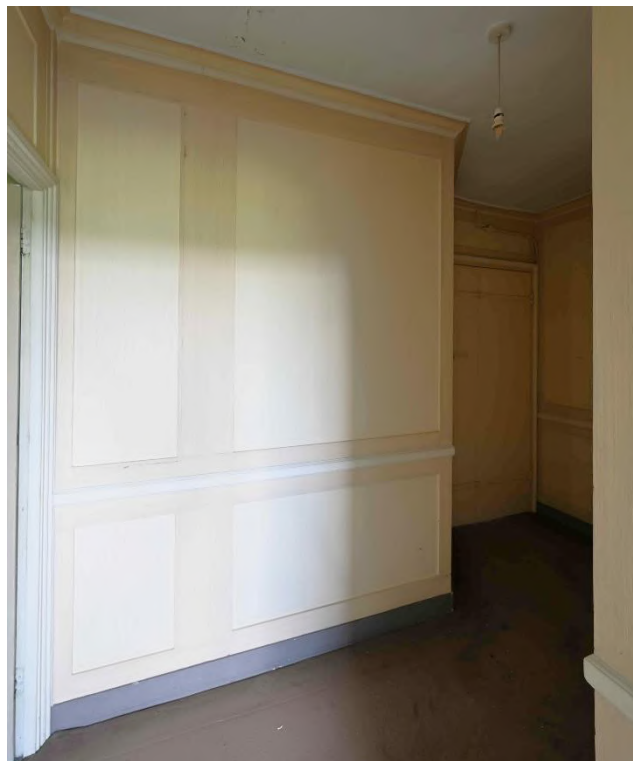
Figure 104: NE internal facade - Hallway SR20
