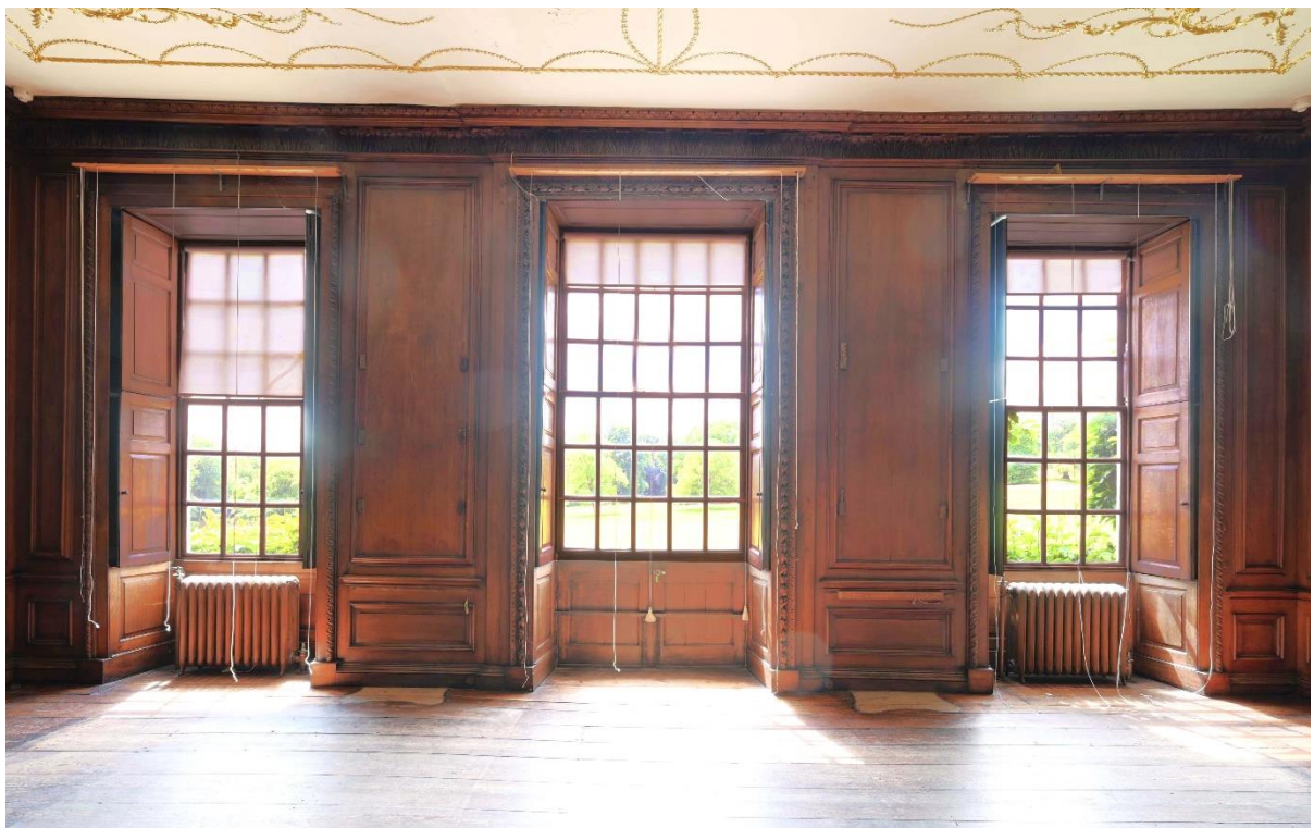
Figure 35: NE internal facade - Salon GR06
