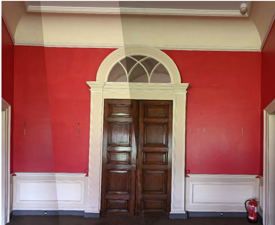
Figure 56: SE internal facade - First Floor - North Hall ST02
