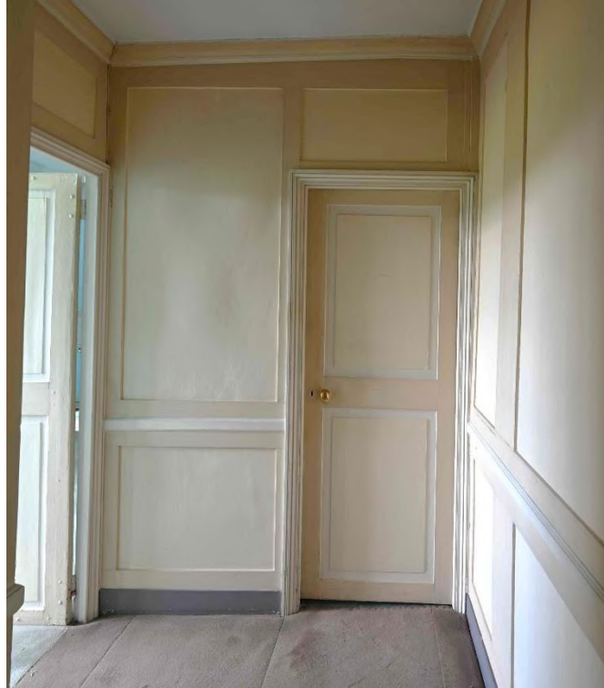
Figure 103: NW internal facade - Hallway SR20
