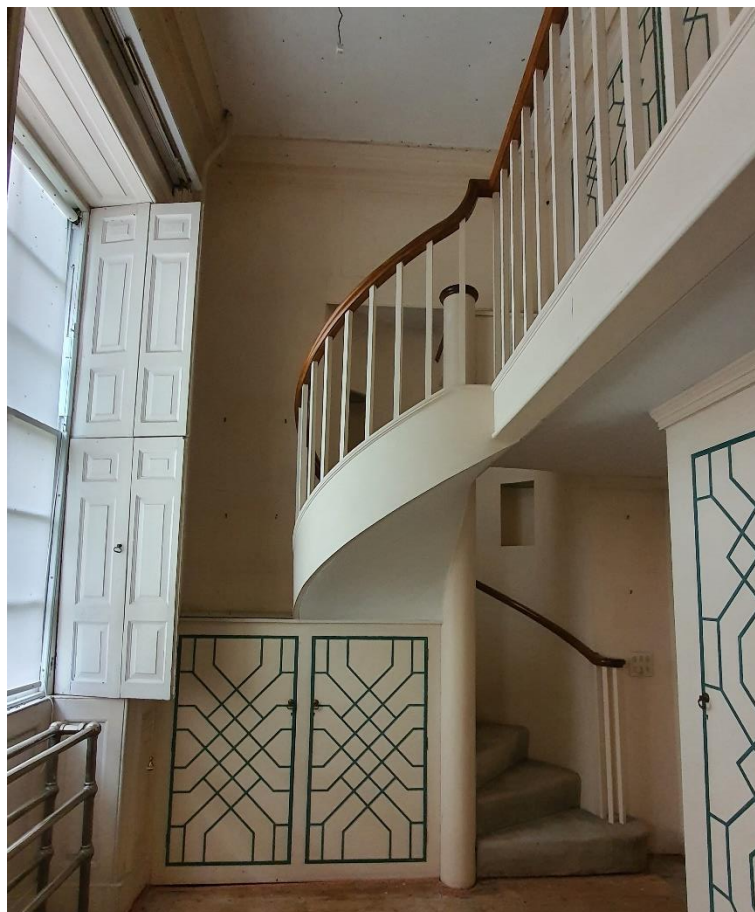
Figure 44: SW internal facade - Mrs. Hyams Dressing Room FR08
