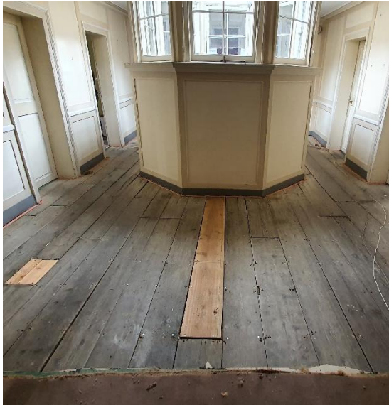
Figure 57: Timber floor exposed after removal of carpet – Central Landing SR10
