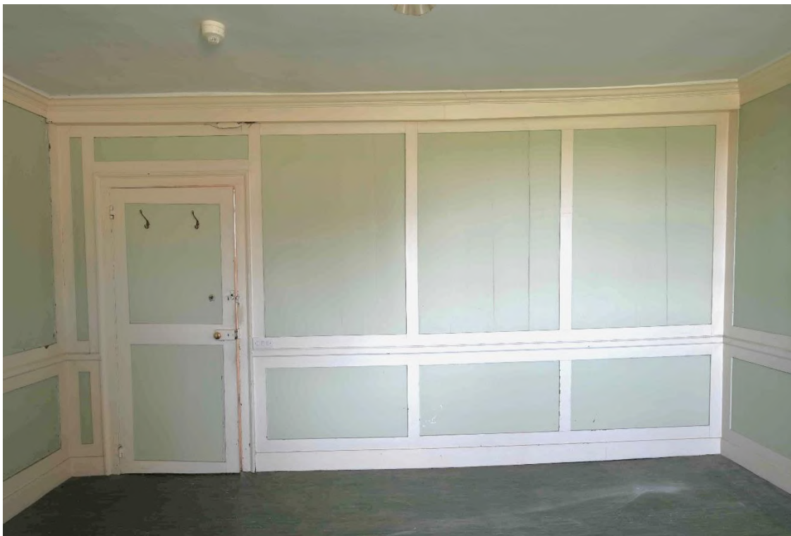
Figure 12: SW internal facade - Storeroom SR03
