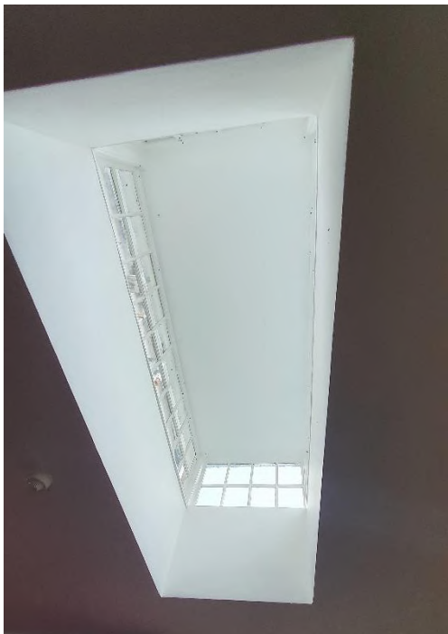
Figure 59: Skylight - Central Landing SR10
