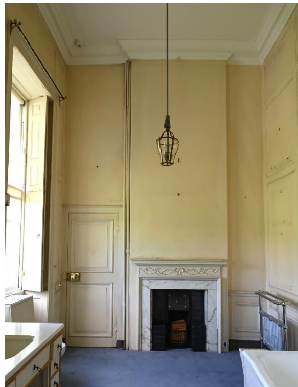
Figure 88: NE internal facade - Mr. Hyams Bathroom FR14
