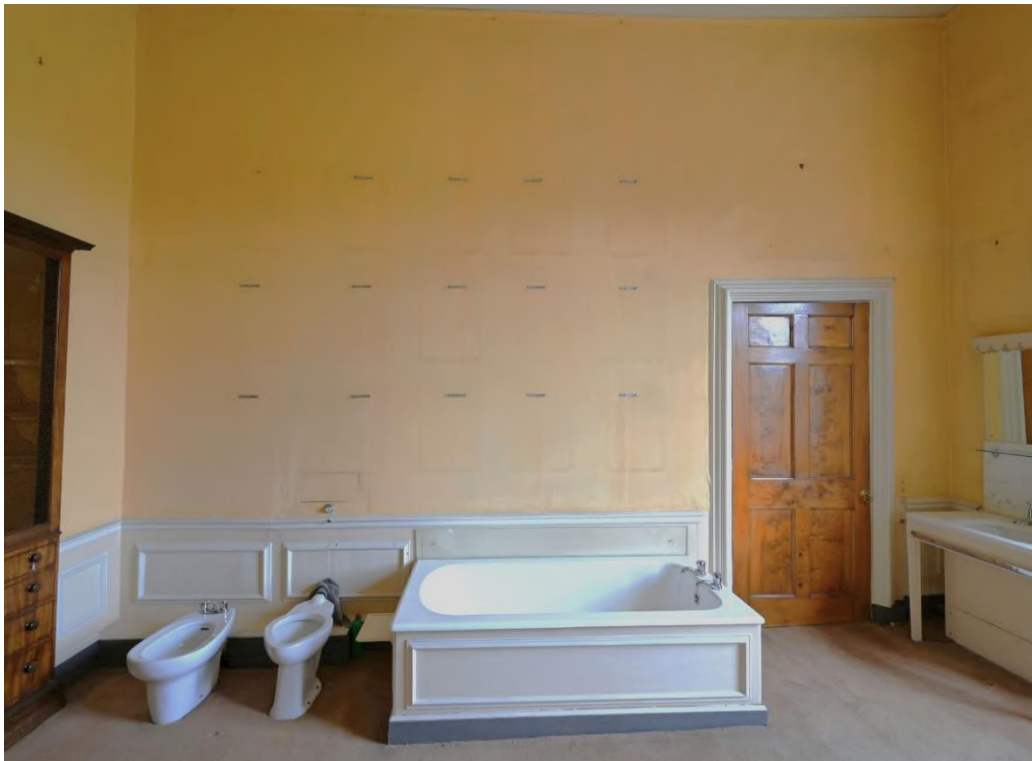
Figure 22: NW internal facade - Chinese Bathroom FR04
