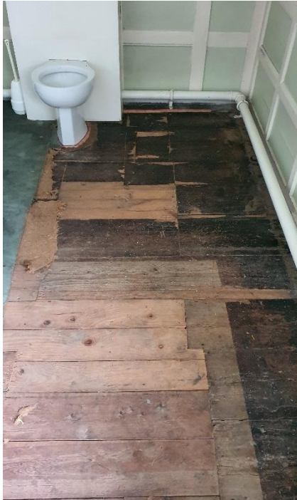
Figure 38: Exposed timber floor post vinyl removal - Bathroom SR07
