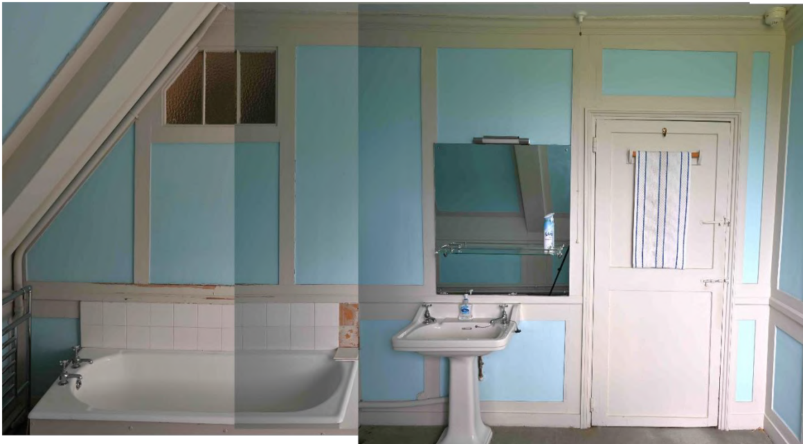
Figure 78: NE internal facade – Staff Bathroom SR14
