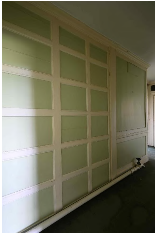
Figure 96: SW internal facade - Corridor SR18
