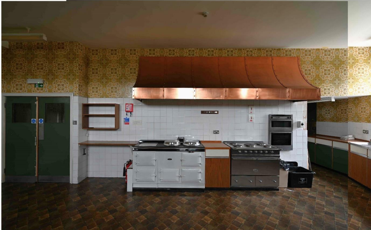
Figure 18: NE internal facade - Main Kitchen LGR07
