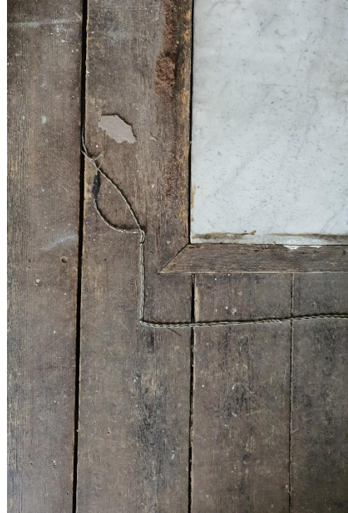
Figure 6: Floorboard threshold with stone hearth - Library GR01
