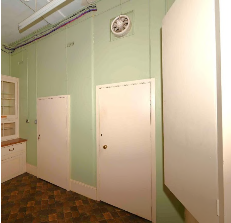
Figure 34: SE internal facade - Projection Room LGR11
