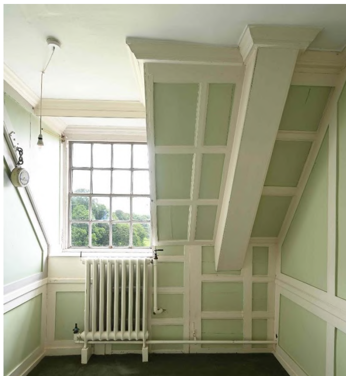
Figure 31: NE internal facade - Dressing Room SR06
