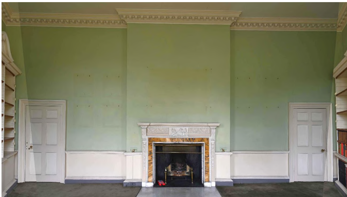
Figure 2: SW internal facade - Library GR01
