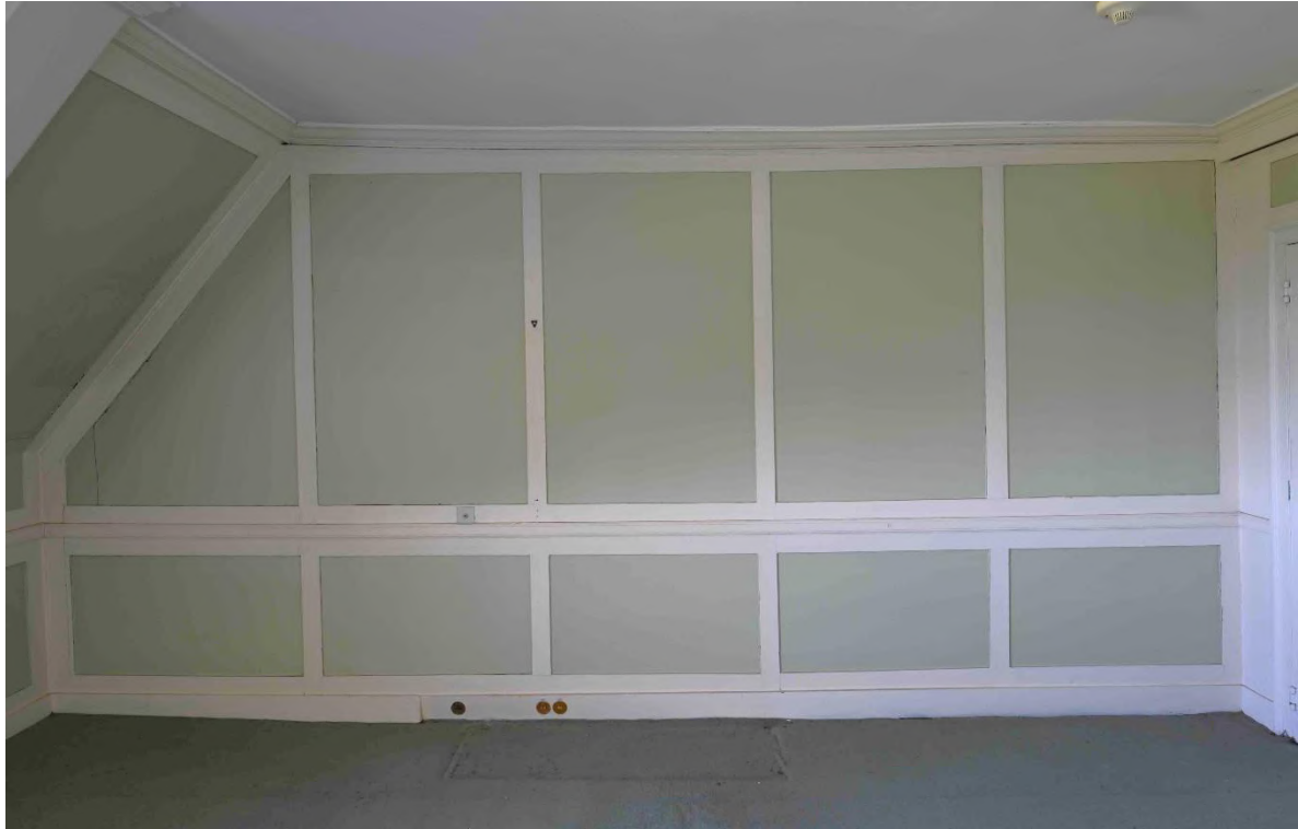
Figure 62: NW internal facade - Storeroom SR11
