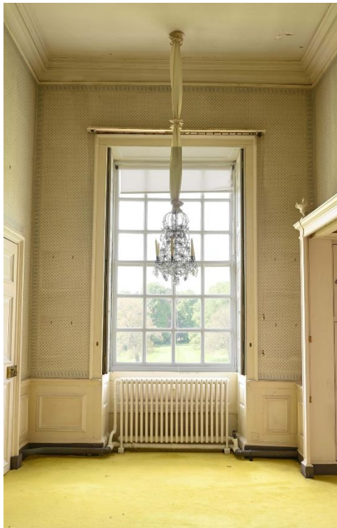
Figure 65: SW internal facade - Mrs. Hyams Bathroom FR10
