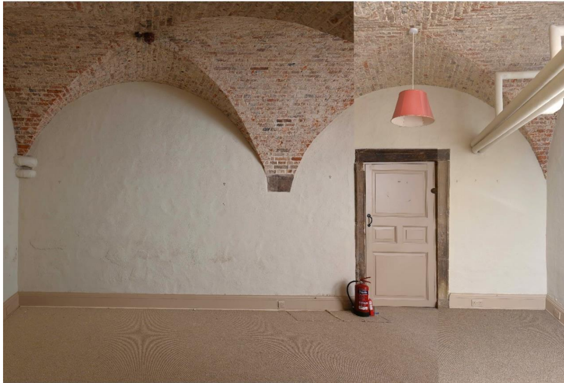
Figure 3: NW internal facade - Games room LGR02
