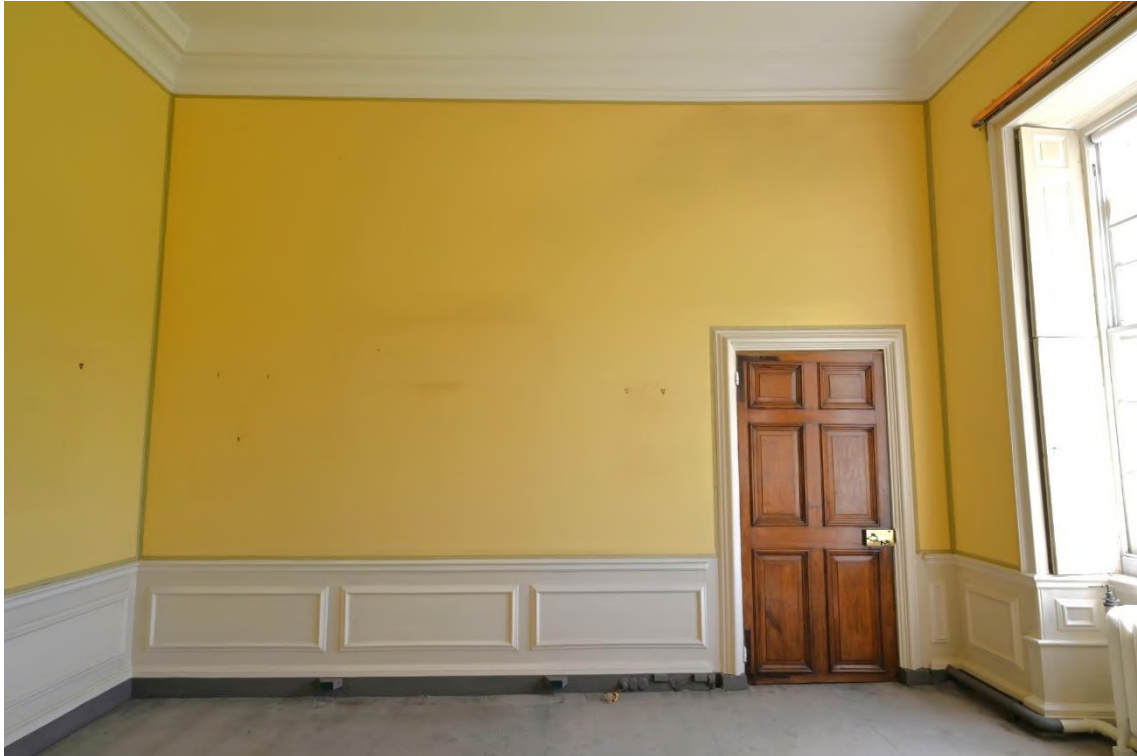
Figure 51: SE internal facade - Yellow Bedroom FR09
