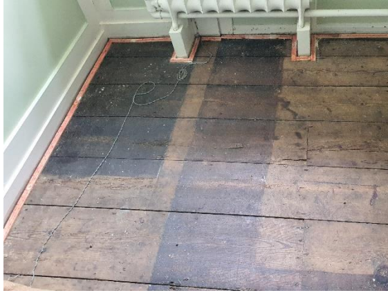
Figure 32: Exposed timber floor post carpet removal - Dressing Room SR06
