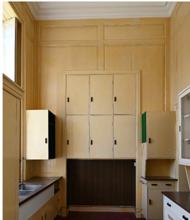
Figure 21: SW internal facade - Butler's Pantry GR04
