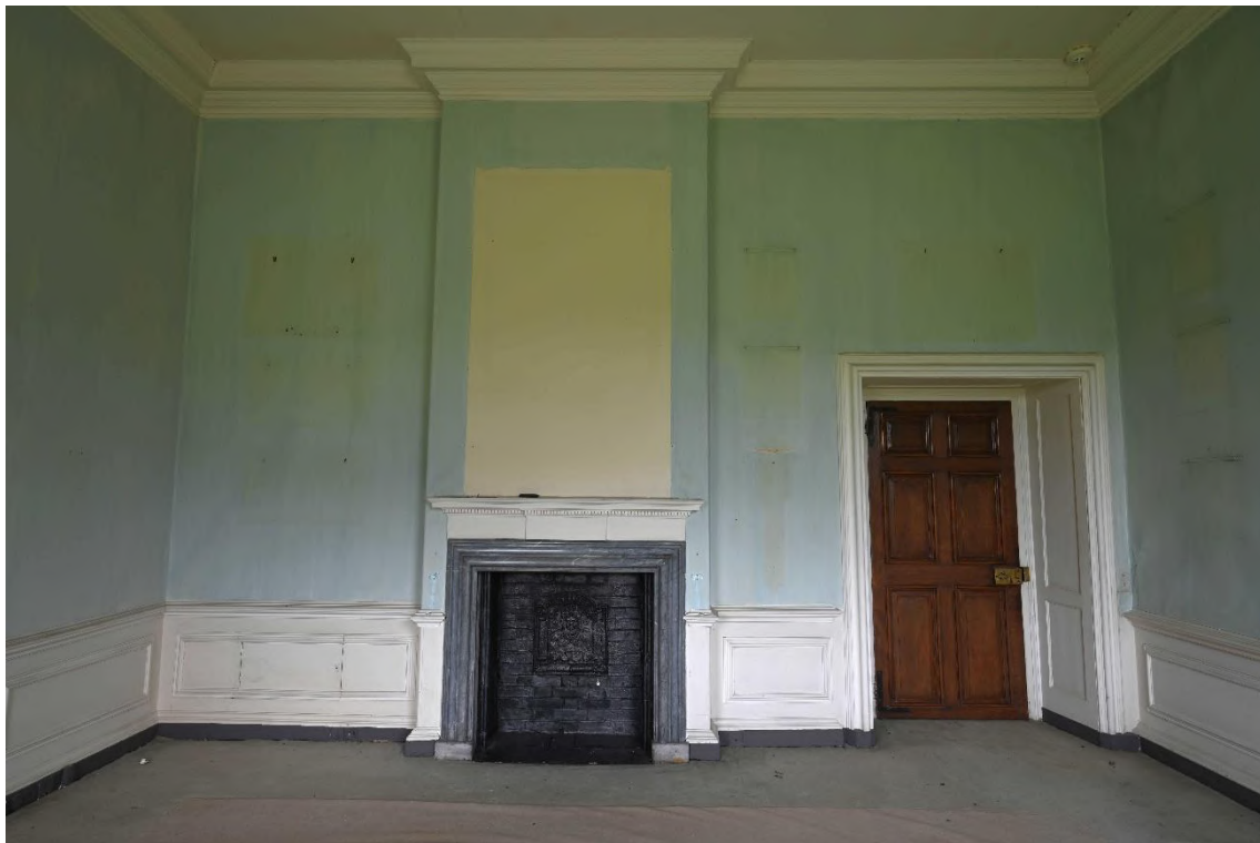
Figure 81: NE internal facade - Mr. Hyams Bedroom FR13
