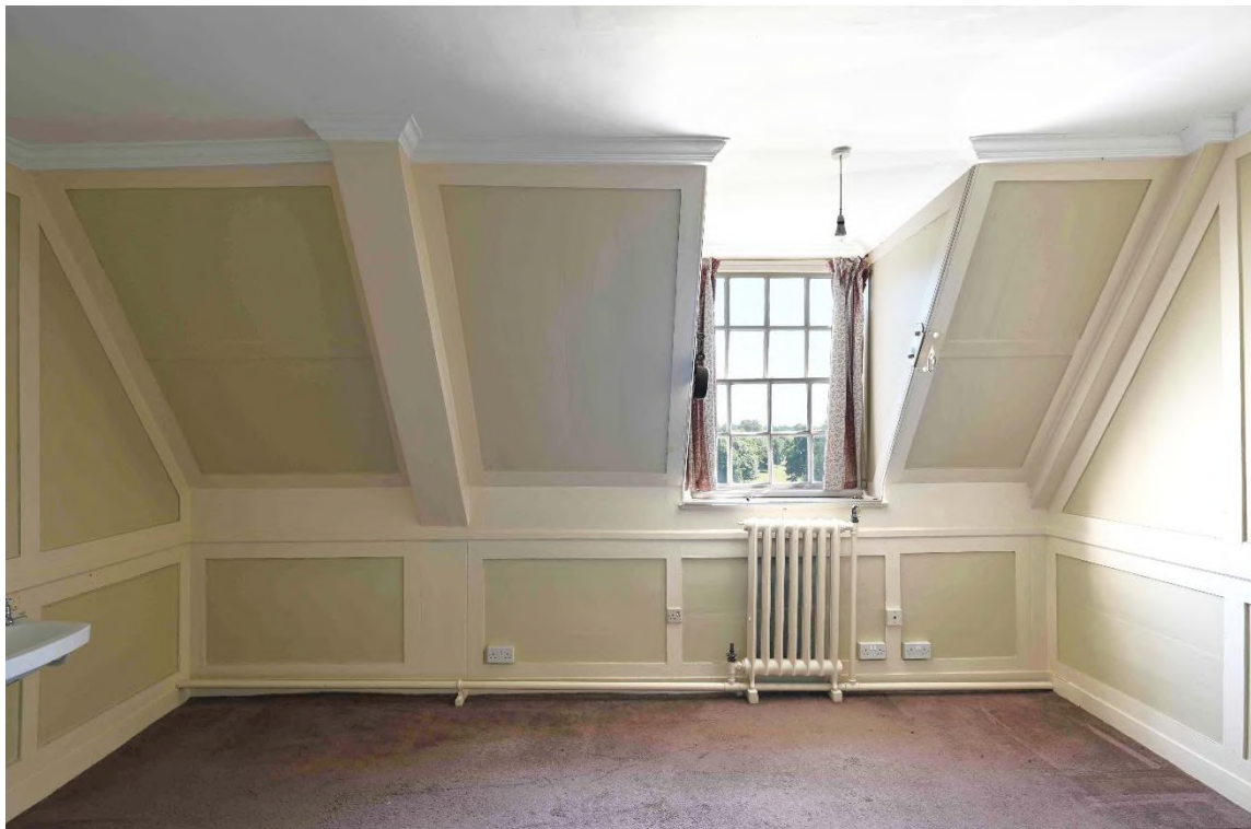
Figure 20: NE internal facade - Bedroom SR04
