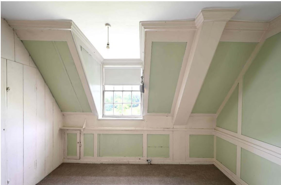
Figure 69: SW internal facade - Sewing Room SR13
