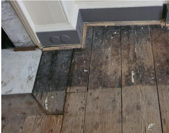
Figure 68: Areas of adhesive from the vinyl that was removed - Mrs. Hyams Bathroom FR10
