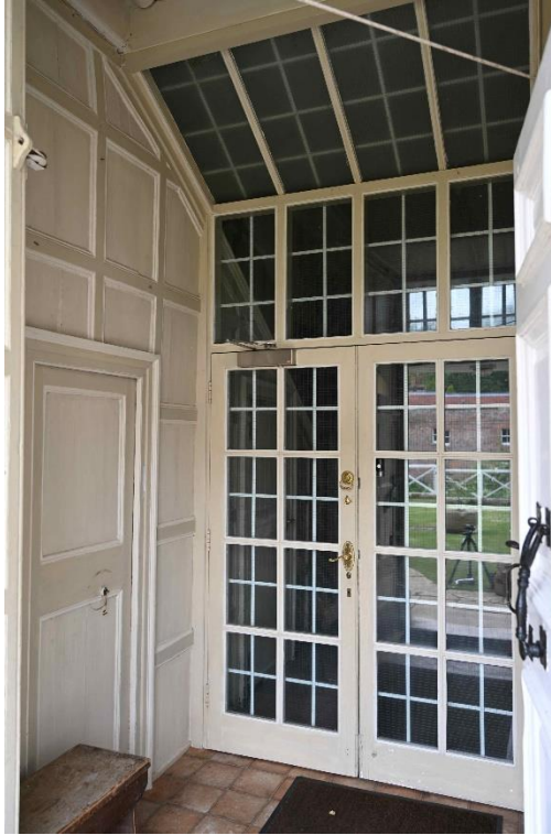
Figure 13: NW internal facade - Lobby LGR06
