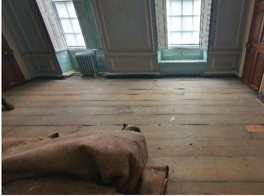
Figure 12: Timber floor, post carpet removal - Blue Bedroom FR02
