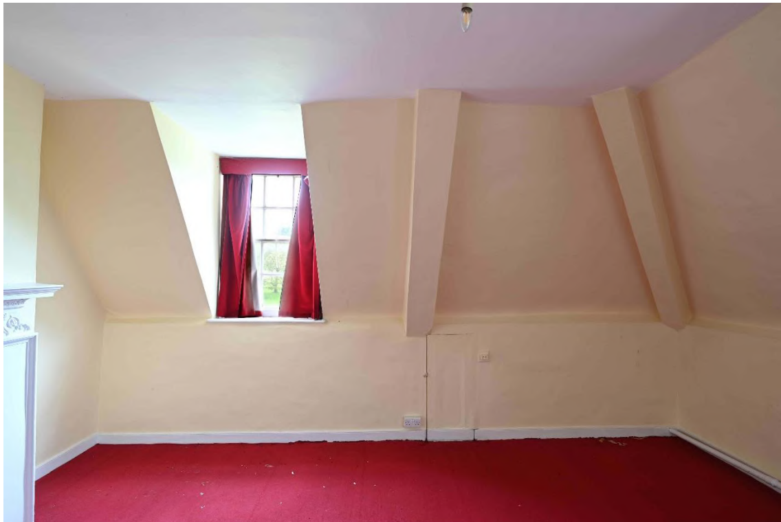
Figure 2: NW internal facade - Staff Bedroom SR01
