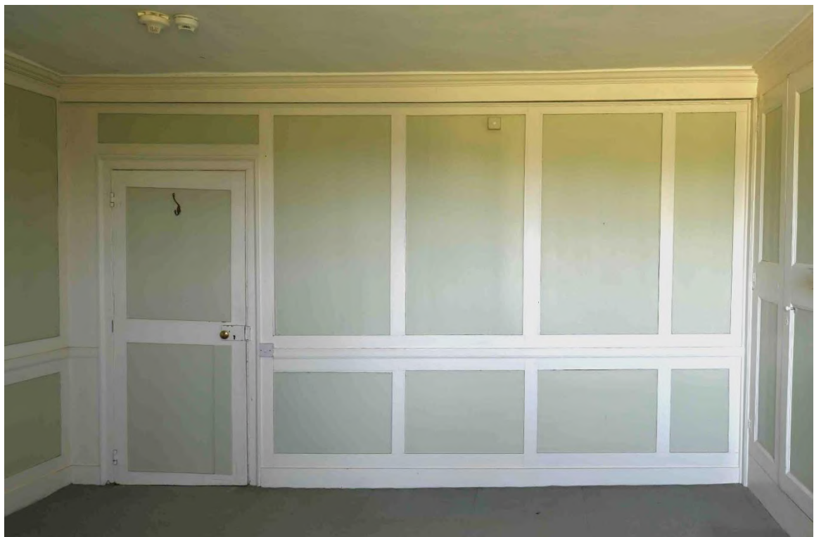
Figure 63: NE internal facade - Storeroom SR11
