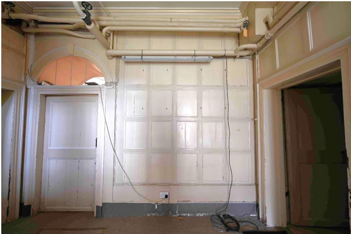
Figure 61: NW internal facade - Lower Ground Floor - Back Stairs ST01
