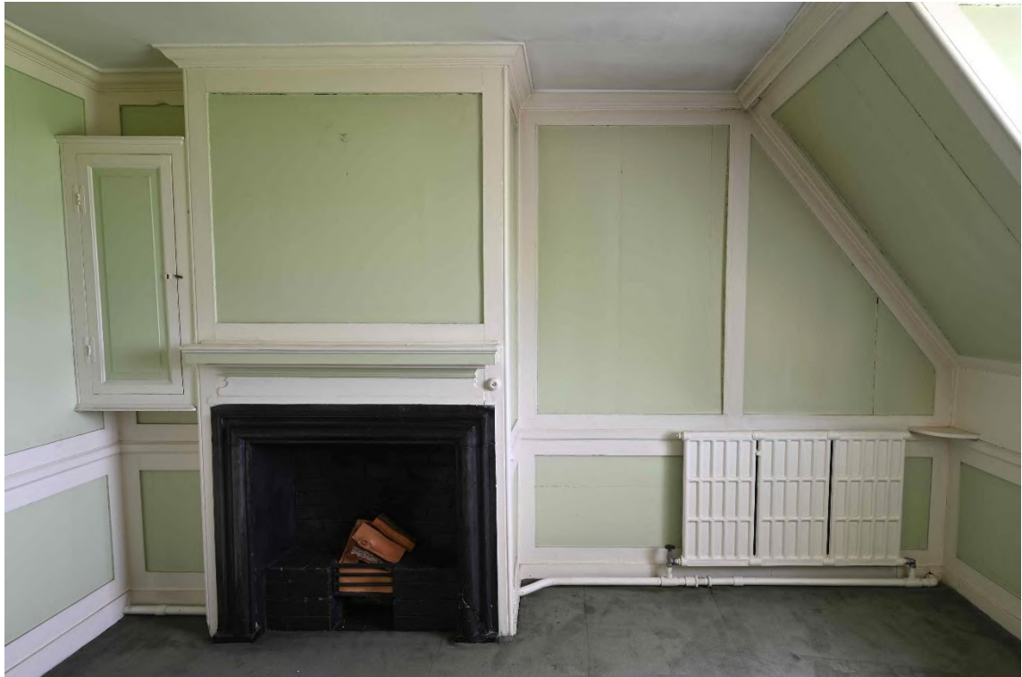
Figure 24: NW internal facade - Bedroom SR05
