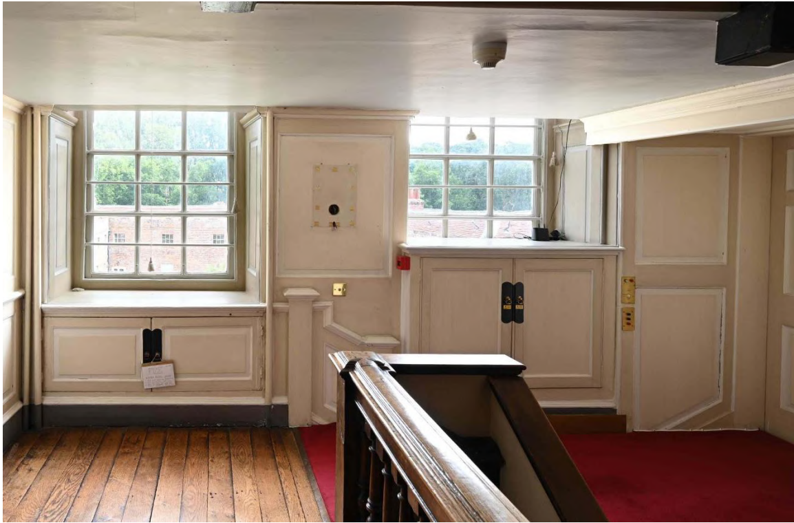
Figure 52: SE internal facade - Ground Floor - Back Stairs ST01
