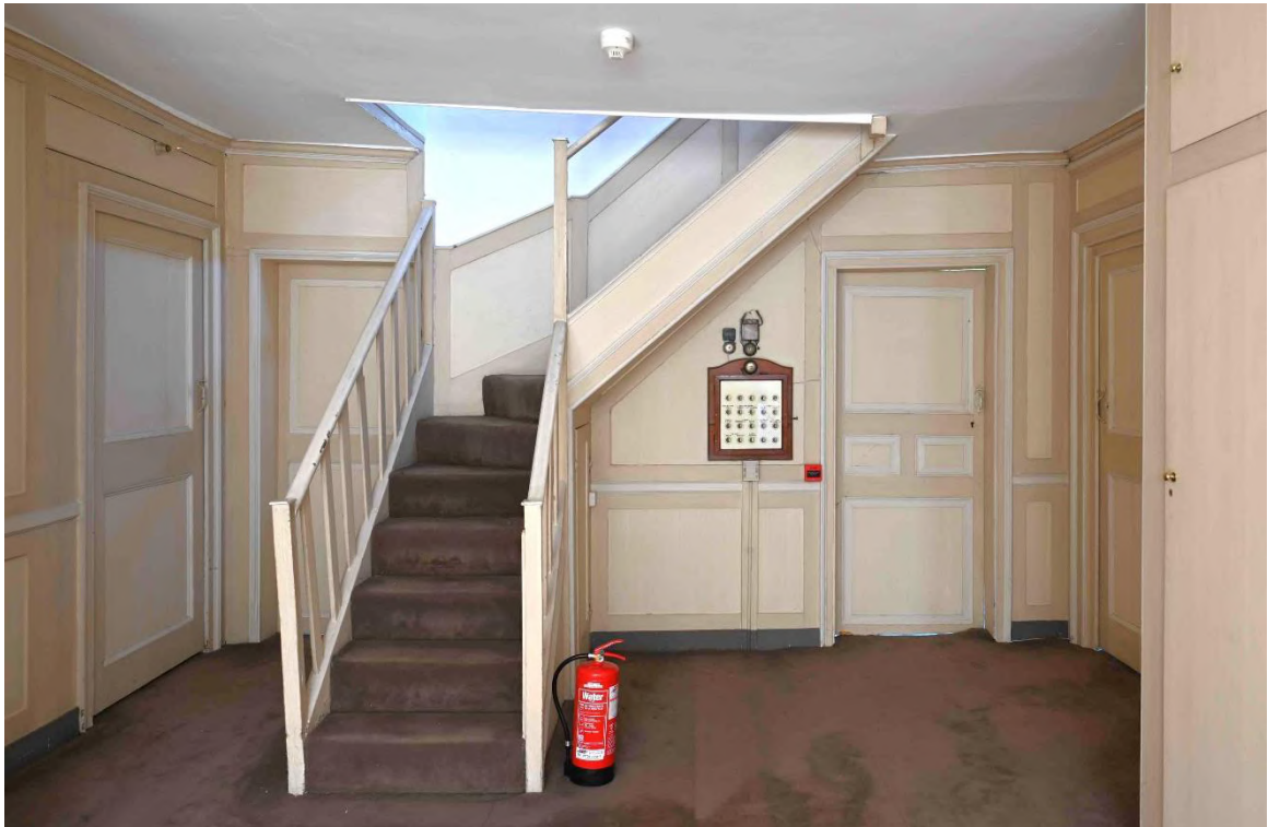
Figure 110: NW internal facade - Stairs to roof ST03
