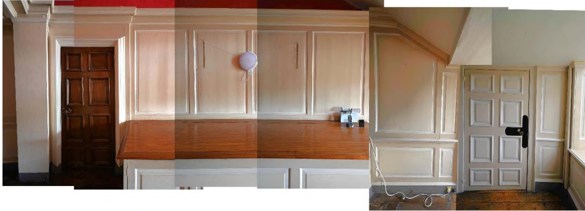
Figure 64: NE internal facade - Ground Floor - Back Stairs ST01
