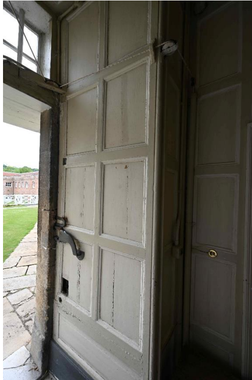
Figure 11: SE internal facade - Lobby LGR06
