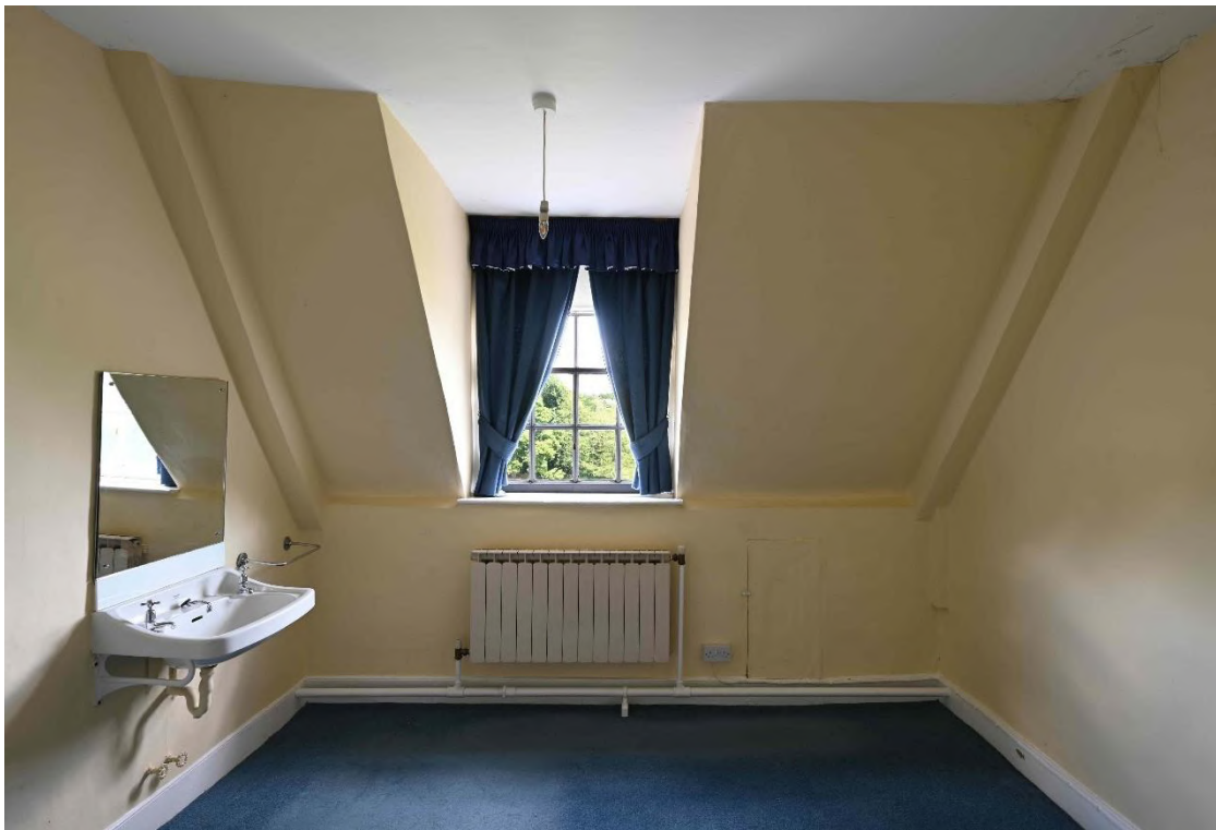
Figure 9: NE internal facade - Staff Sitting Room SR02
