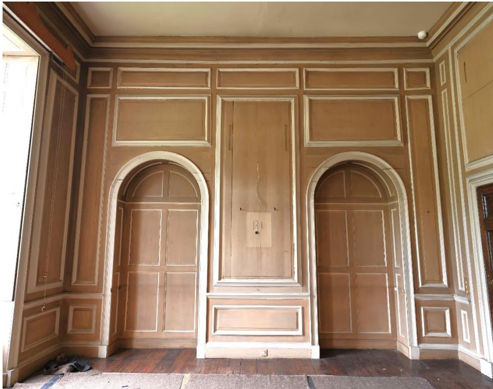
Figure 14: SE internal facade - Large Dining Room GR03
