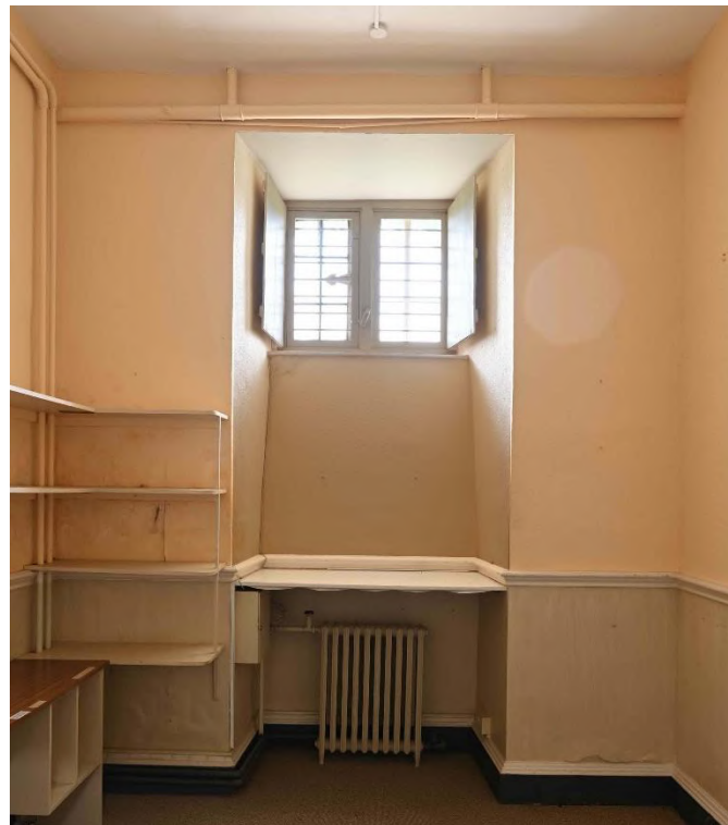
Figure 26: SW internal facade - Office LGR09
