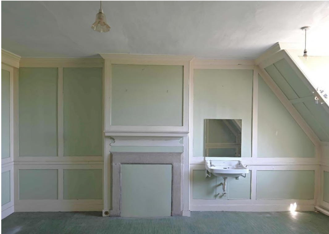
Figure 13: NW internal facade - Storeroom SR03
