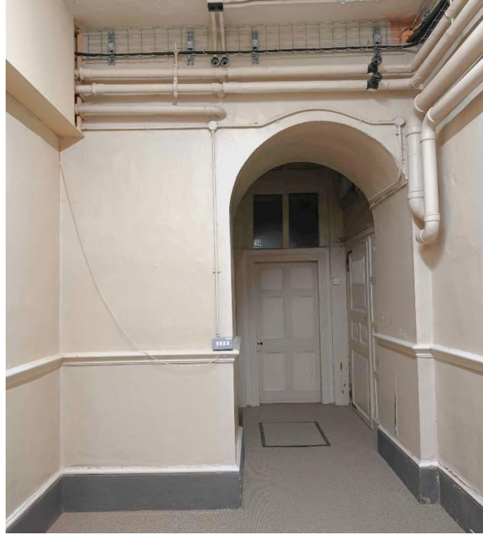
Figure 31: NW internal facade - LGR10
