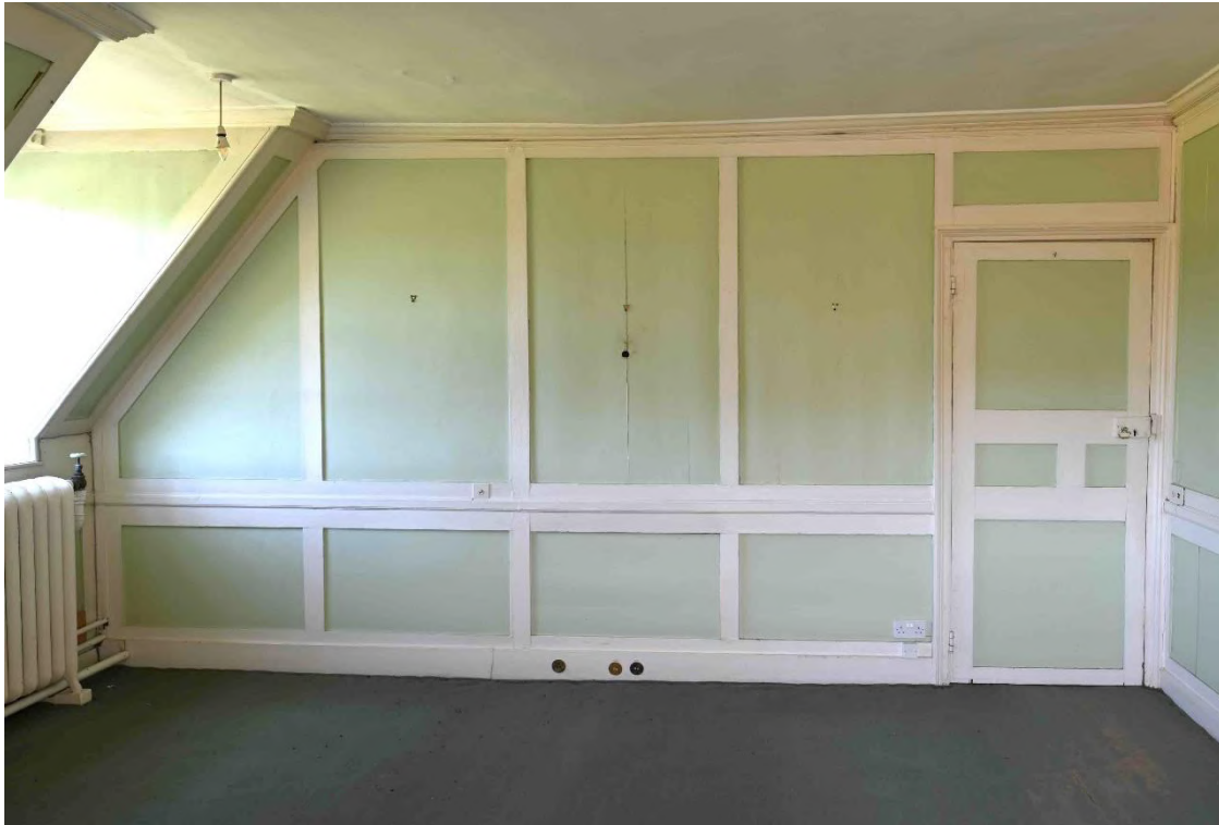
Figure 42: NW internal facade - Green Bedroom SR08
