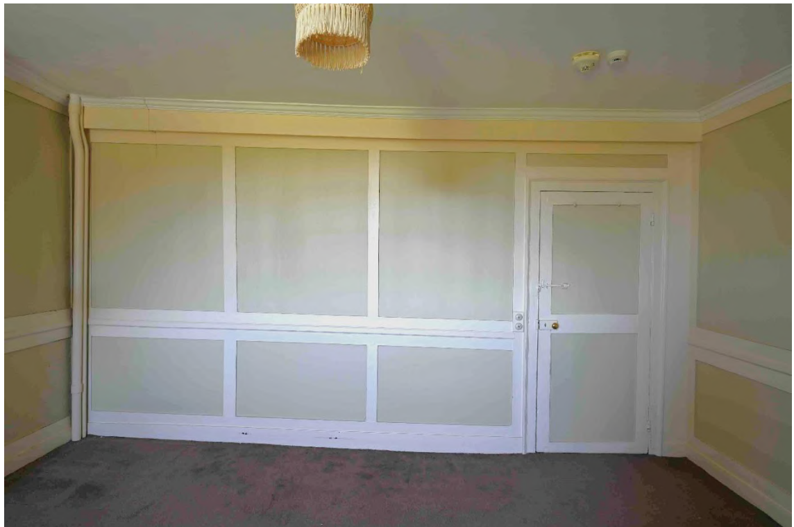
Figure 18: SW internal facade - Bedroom SR04
