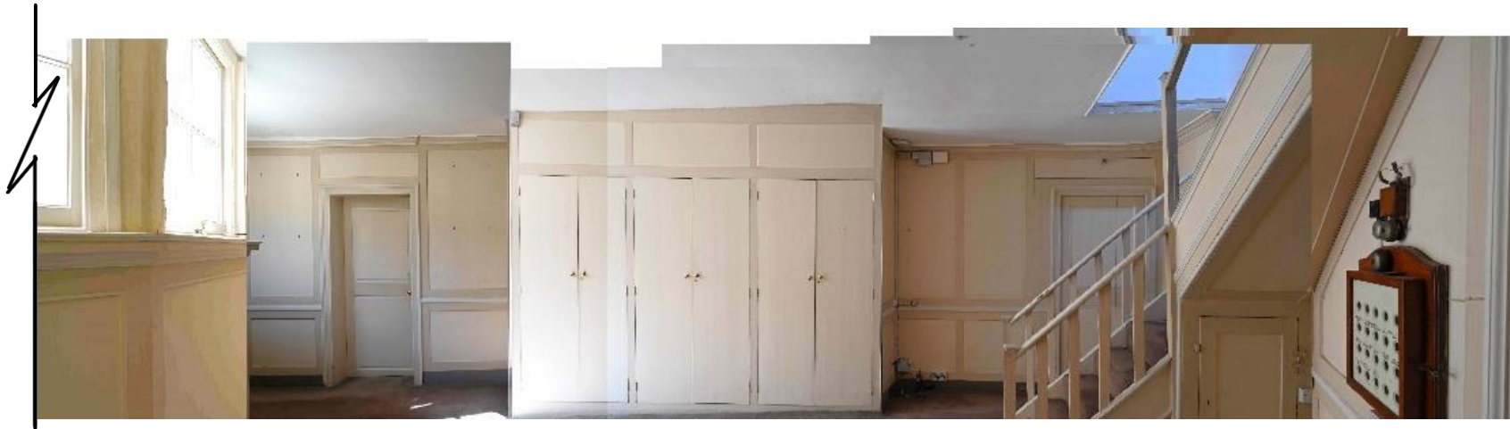
Figure 54: SW internal facade - Central Landing SR10
