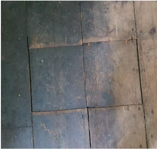
Figure 26: Exposed timber floor post carpet removal - Bedroom SR05
