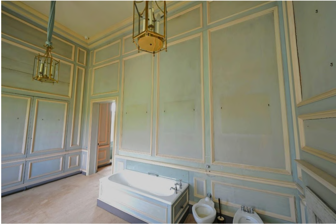
Figure 1: SE internal facade - Blue Bathroom FR01
