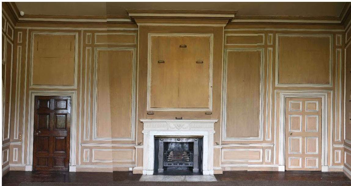
Figure 15: SW internal facade - Large Dining Room GR03
