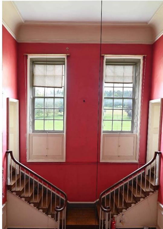
Figure 60: NW internal facade - First Floor - North Hall ST02
