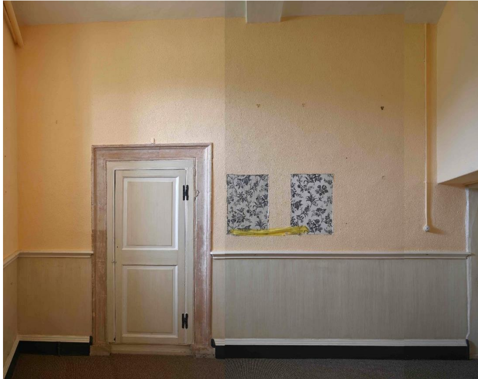
Figure 27: NW internal facade - Office LGR09
