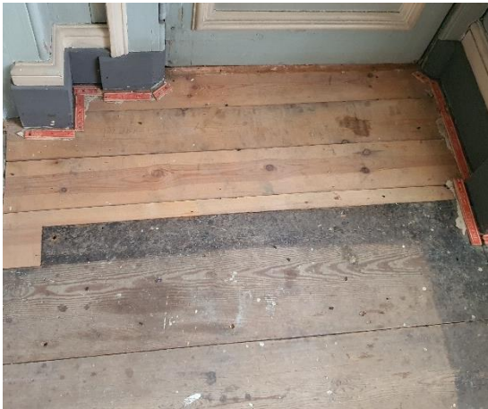
Figure 7: Timber floor, post carpet removal - Blue Bathroom FR01
