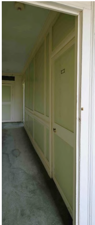
Figure 98: NE internal facade - Corridor SR18
