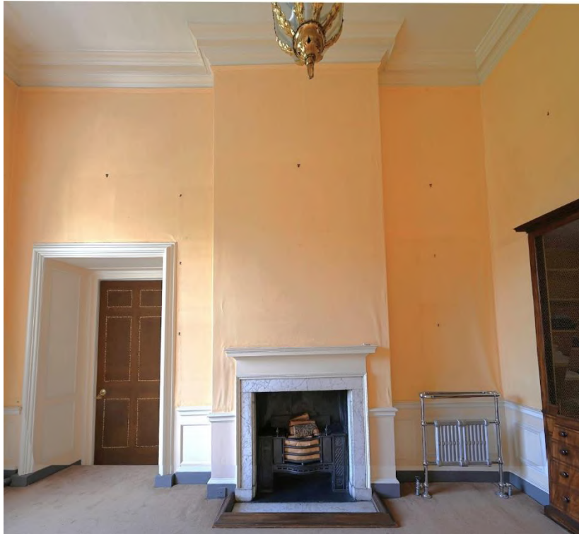
Figure 20: SE internal facade - Chinese Bathroom FR04
