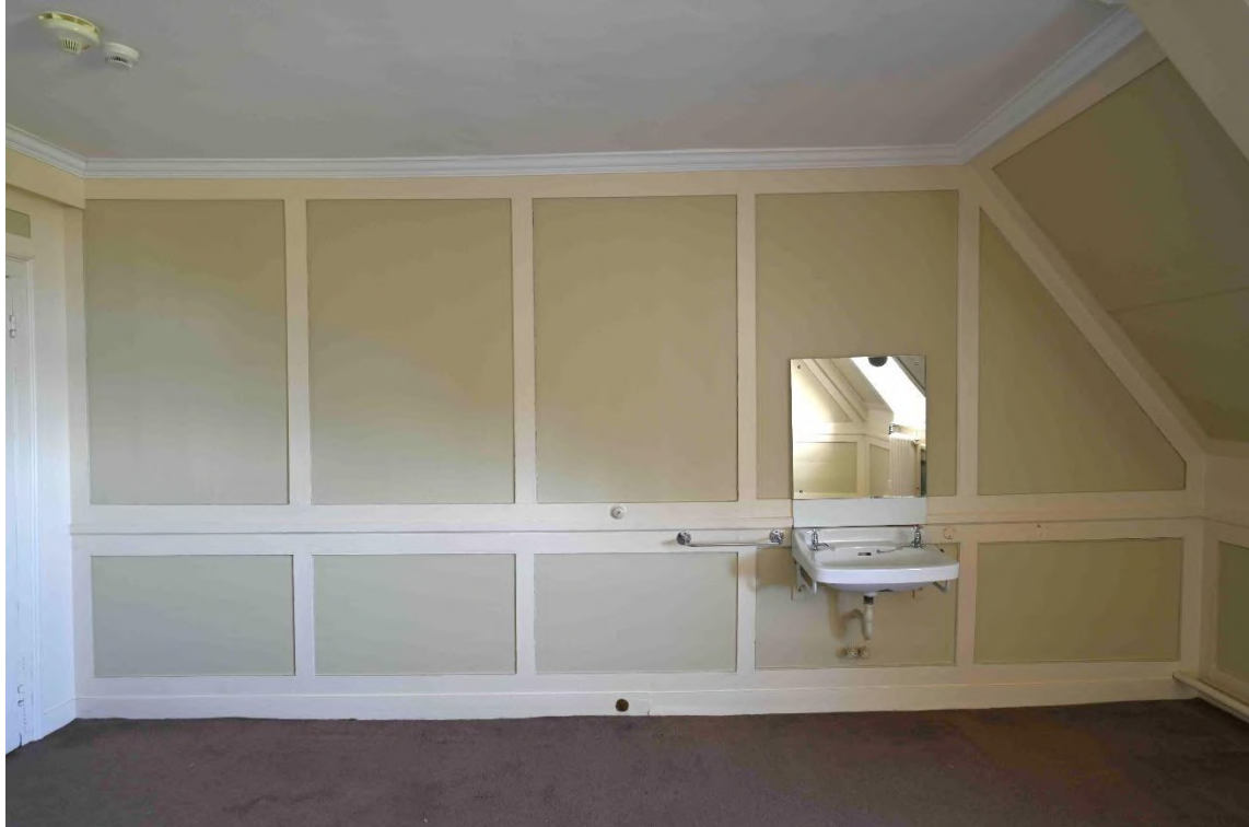
Figure 19: NW internal facade - Bedroom SR04
