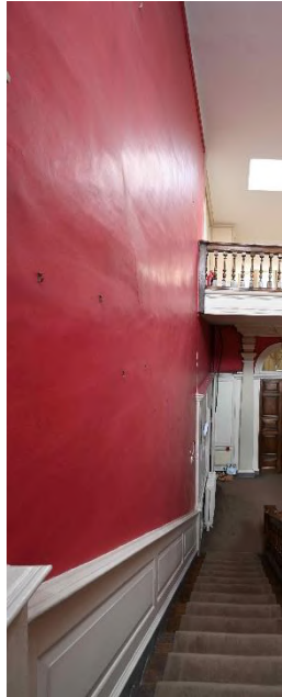
Figure 54: SW internal facade - Second Floor - Back Stairs ST01
