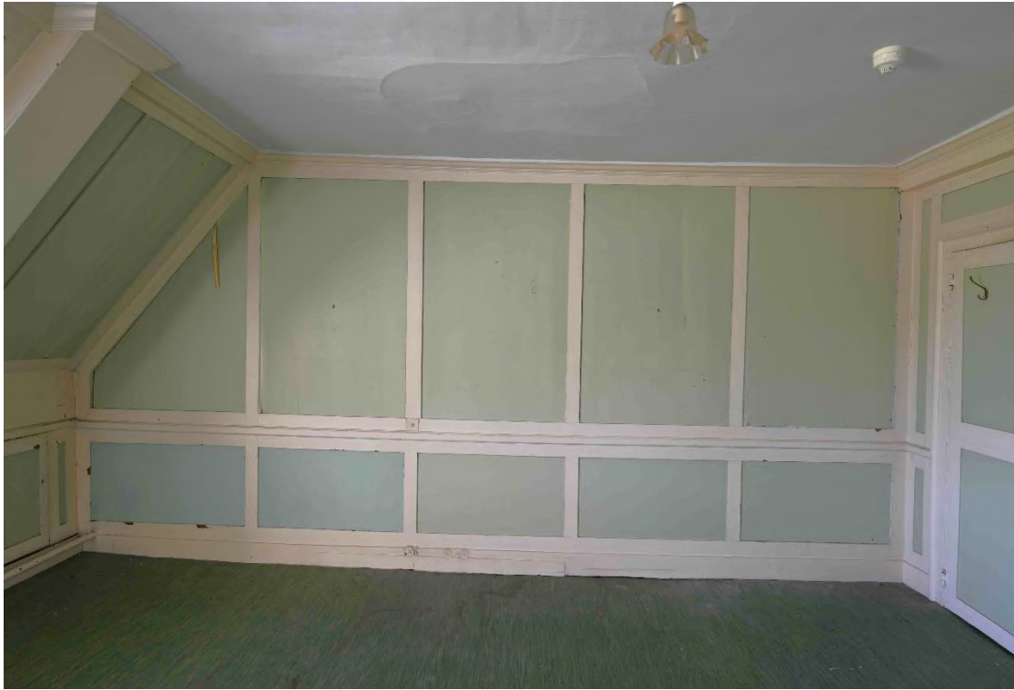
Figure 11: SE internal facade - Storeroom SR03
