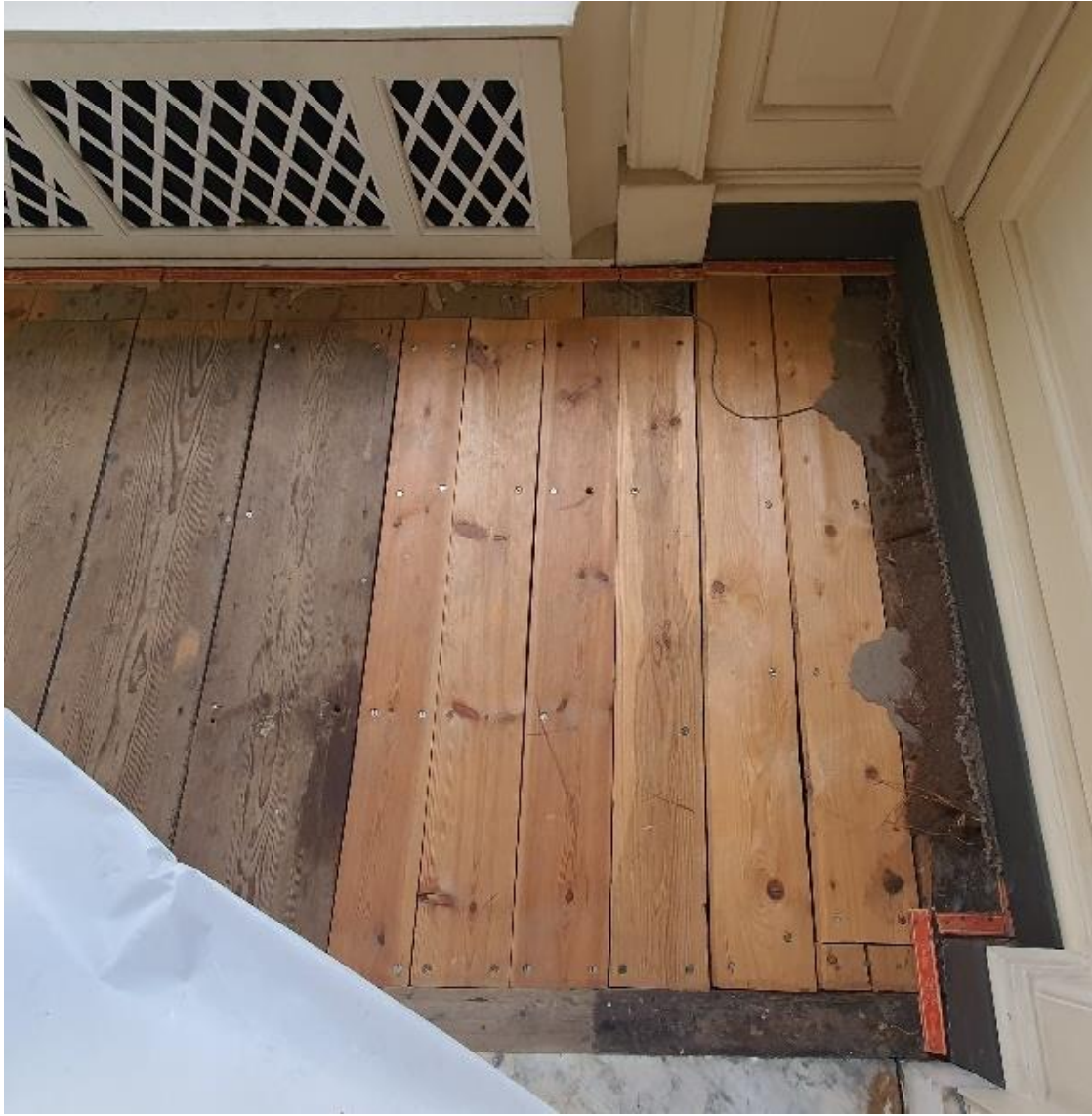
Figure 46: Floorboards - Chinese Sitting Room GR07
