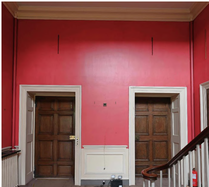
Figure 57: SE internal facade - Ground Floor - North Hall ST02
