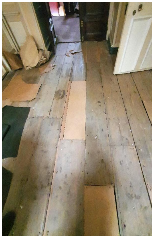
Figure 63: Timber boards and visible old repairs, post carpet removal - Corridor FR11
