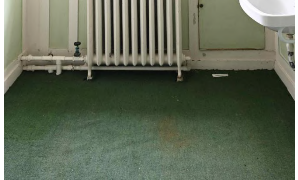
Figure 16: Radiator and floor - Storeroom SR03
