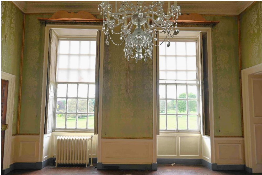
Figure 26: SW internal facade - Small Dining Room GR05
