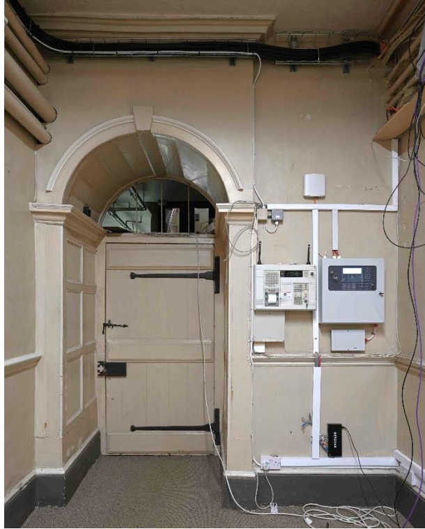
Figure 29: SE internal facade - LGR10
