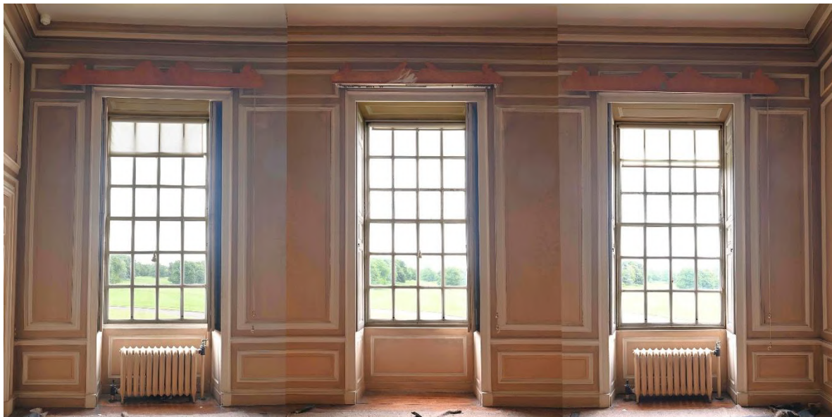
Figure 17: NE internal facade - Large Dining Room GR03
