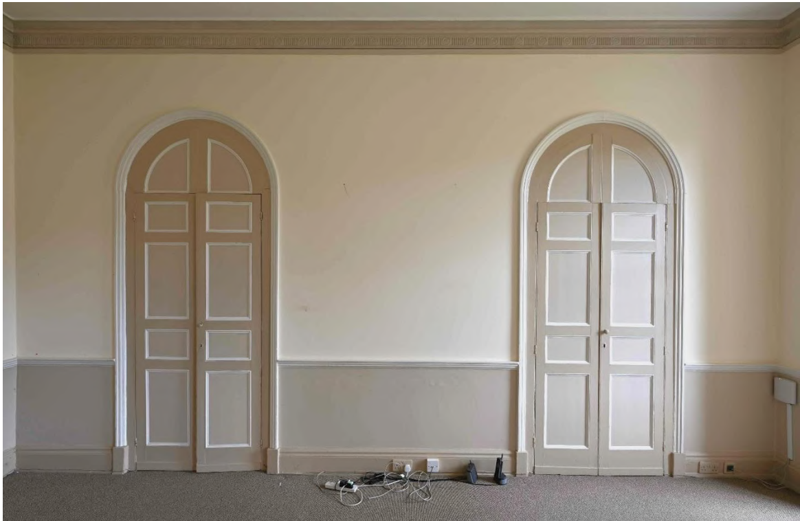
Figure 10: NE internal facade - Staff Room LGR05
