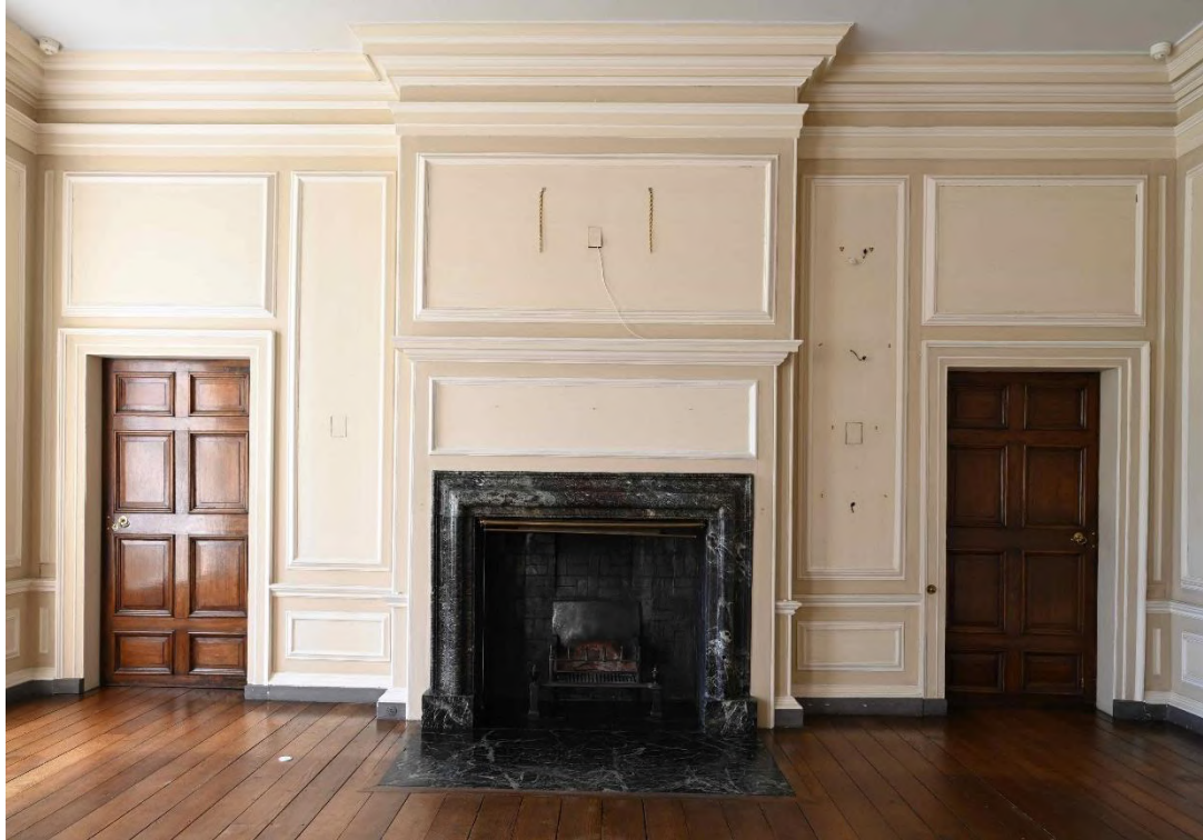
Figure 10: NW internal facade - Hall GR02
