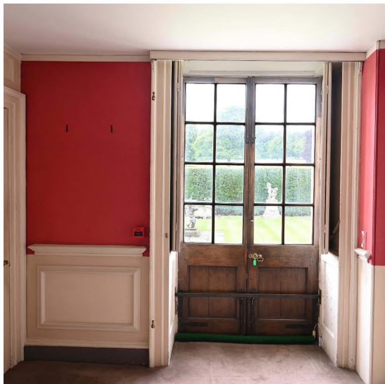
Figure 61: NW internal facade - Ground Floor - North Hall ST02
