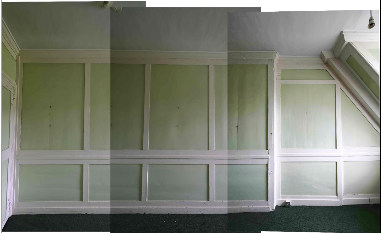
Figure 85: SW internal facade - Staff Bathroom SR16
