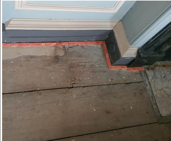
Figure 13: Timber floor, post carpet removal - Blue Bedroom FR02
