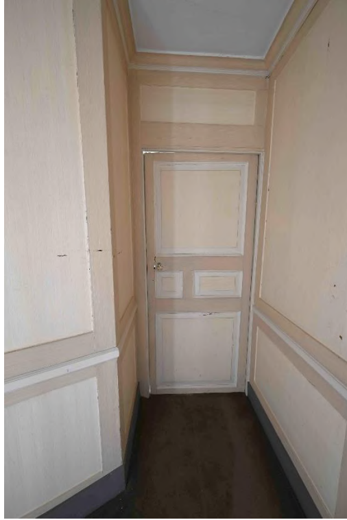
Figure 107: SE internal facade - Hallway SR22
