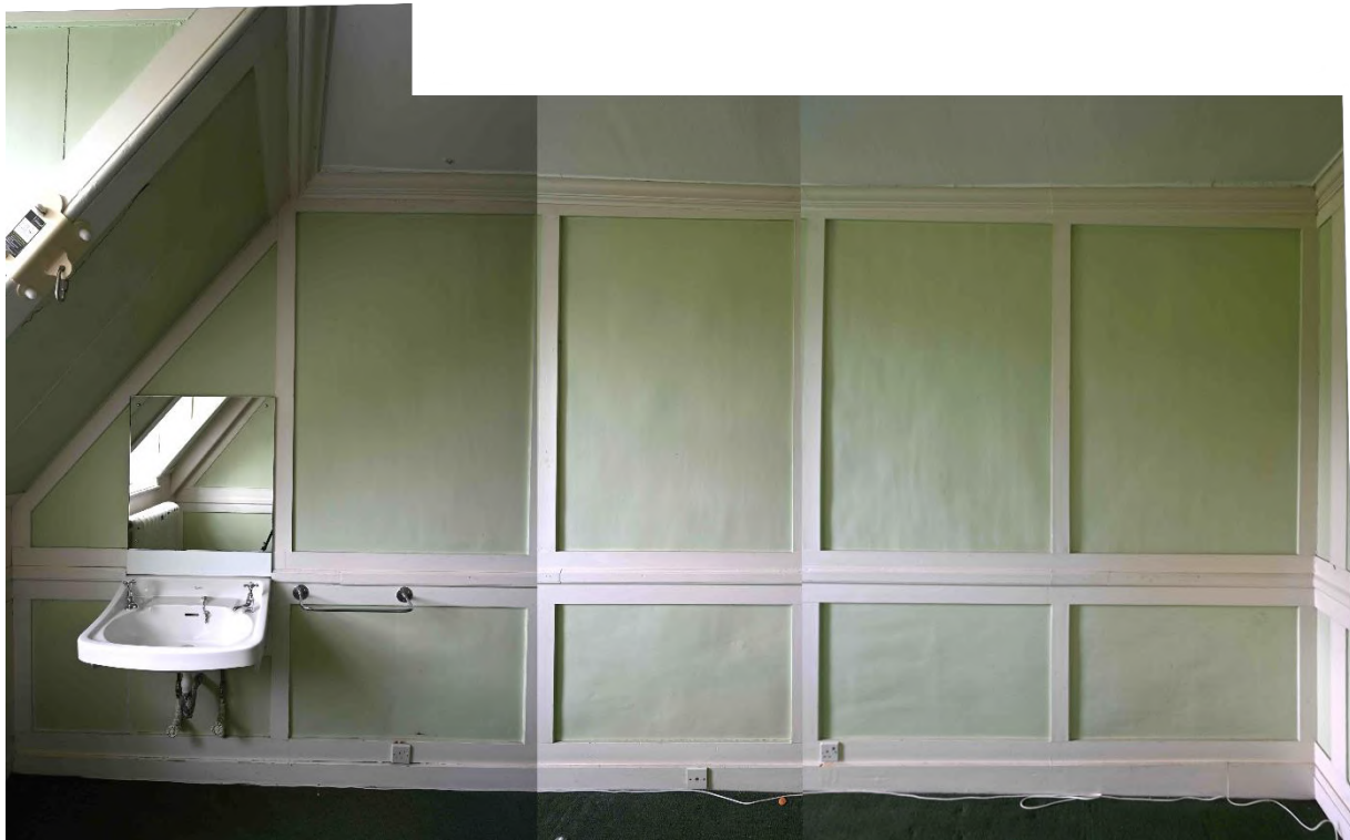
Figure 87: NE internal facade - Staff Bathroom SR16
