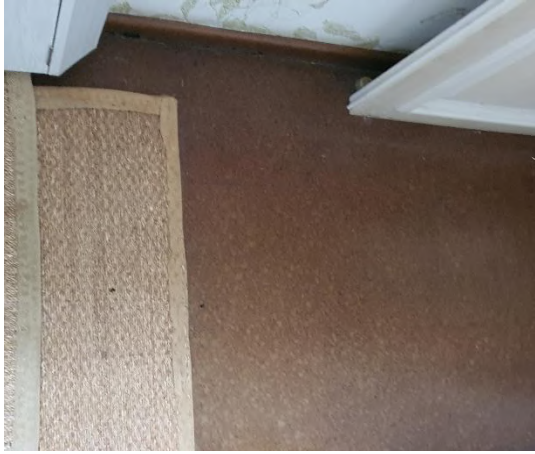
Figure 42: Existing vinyl floor - Model Kitchen FR07
