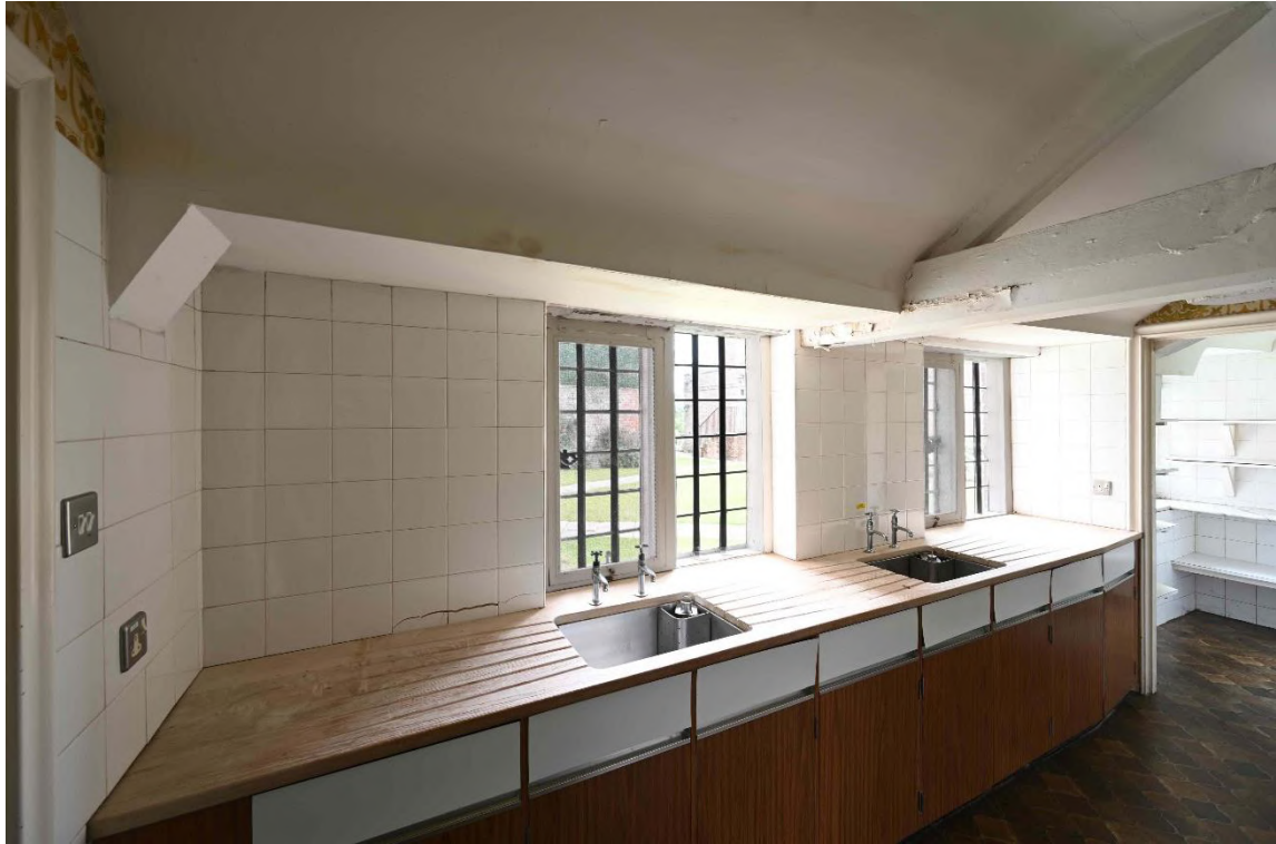
Figure 24: NE internal facade - Scullery LGR08
