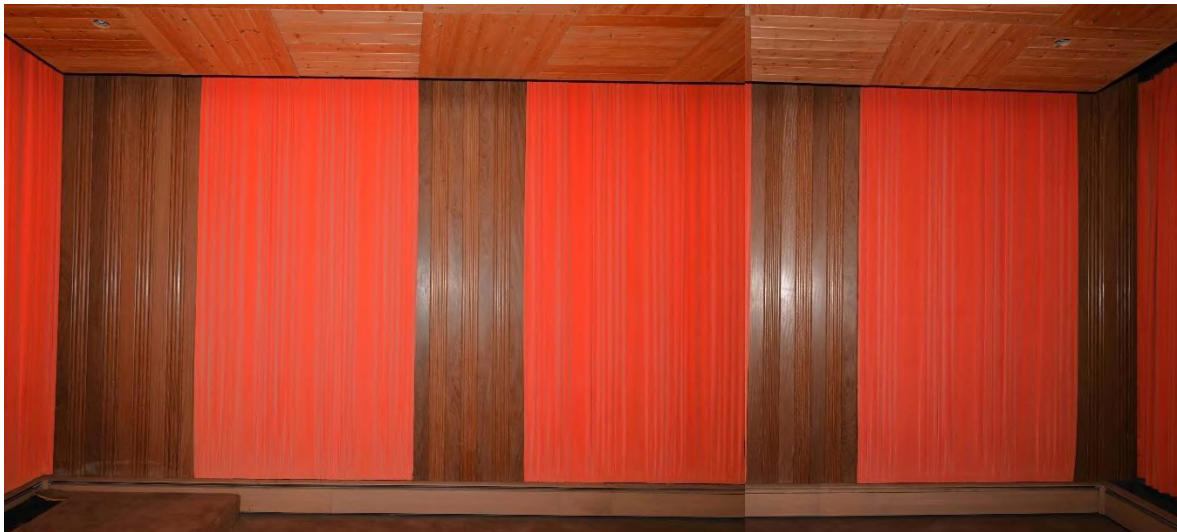
Figure 41: SW internal facade - Cinema LGR12
