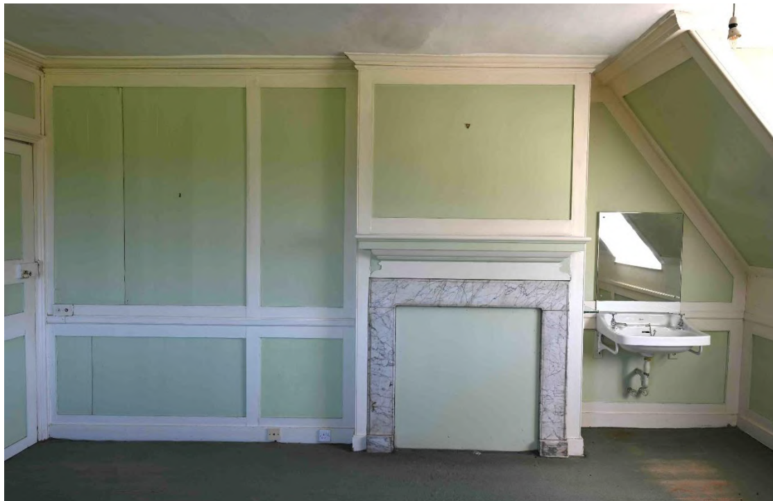
Figure 43: NE internal facade - Green Bedroom SR08
