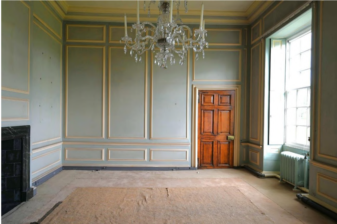
Figure 10: NW internal facade - Blue Bedroom FR02
