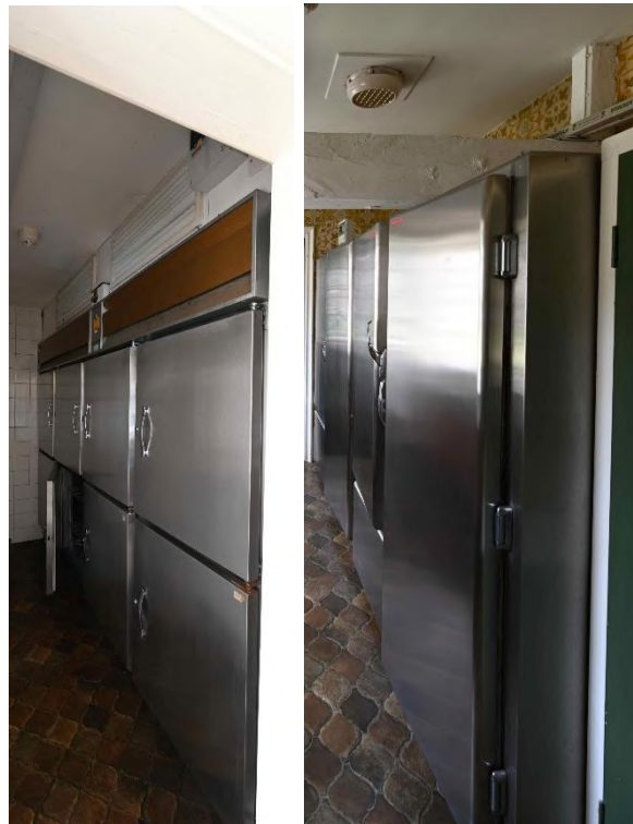
Figure 23: SW internal facade - Scullery LGR08
