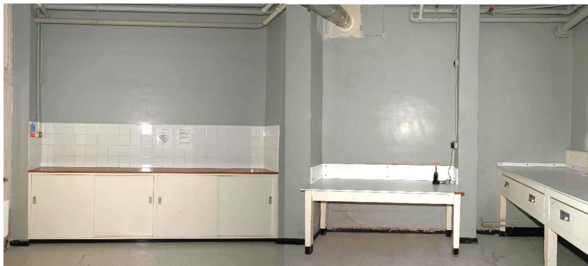
Figure 45: SW internal facade - Laundry Room LGR13
