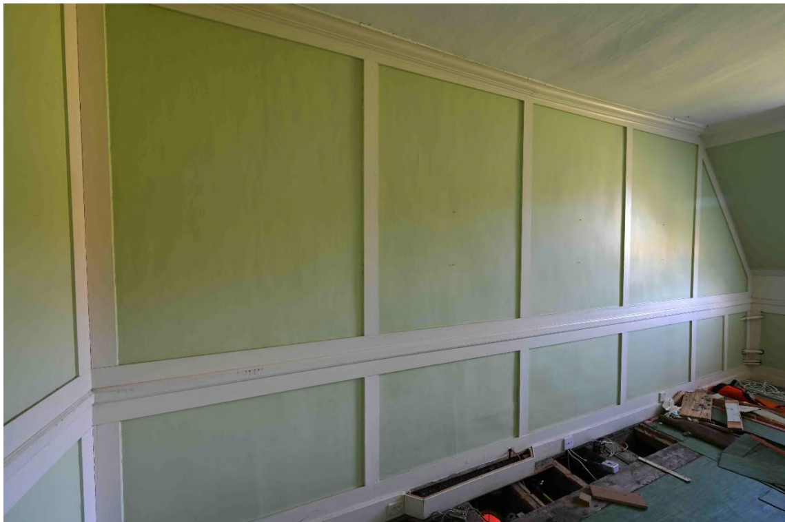
Figure 90: SW internal facade - Staff Bathroom SR17
