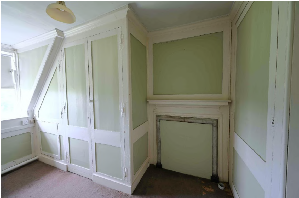
Figure 50: NW internal facade - Linen Room SR09
