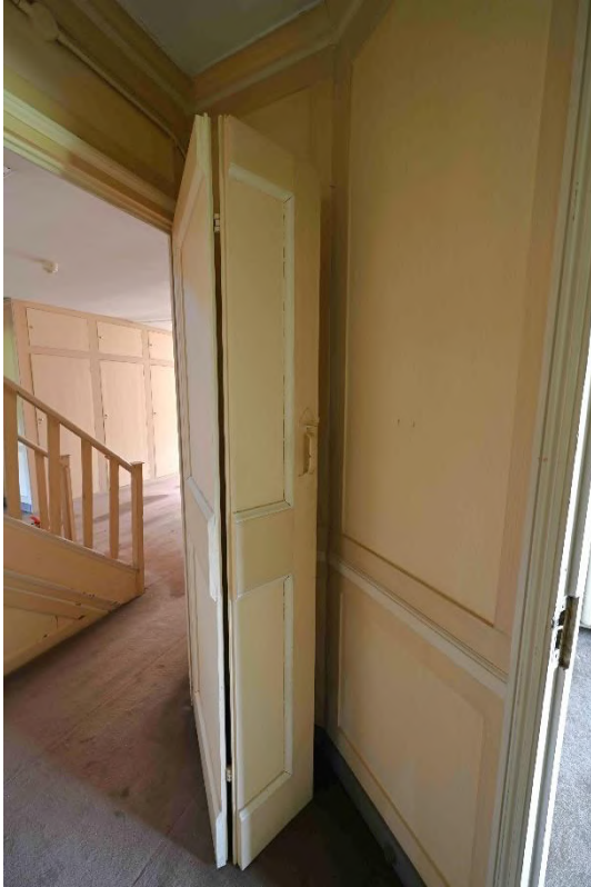
Figure 105: Entry to Hallway SR20
