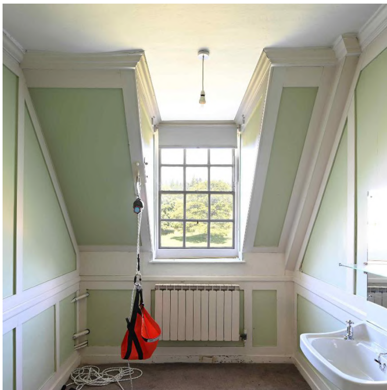
Figure 91: NW internal facade - Staff Bathroom SR17
