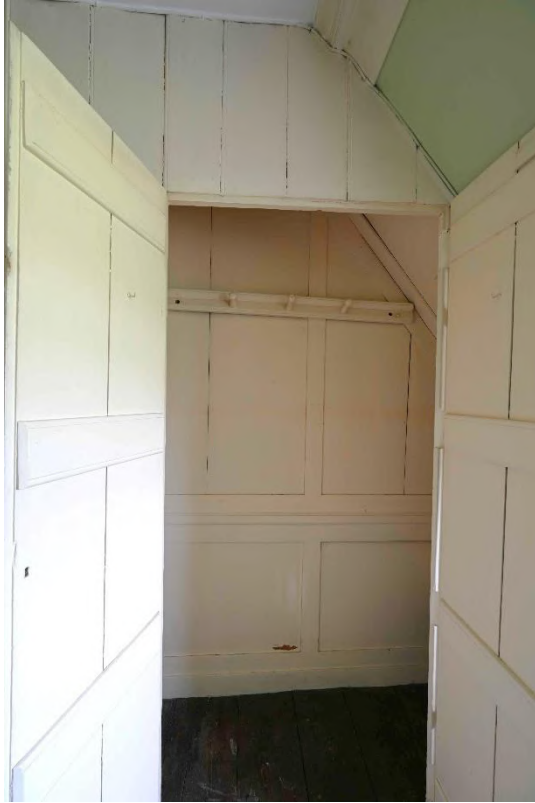
Figure 72: Inside cupboard - Sewing Room SR13
