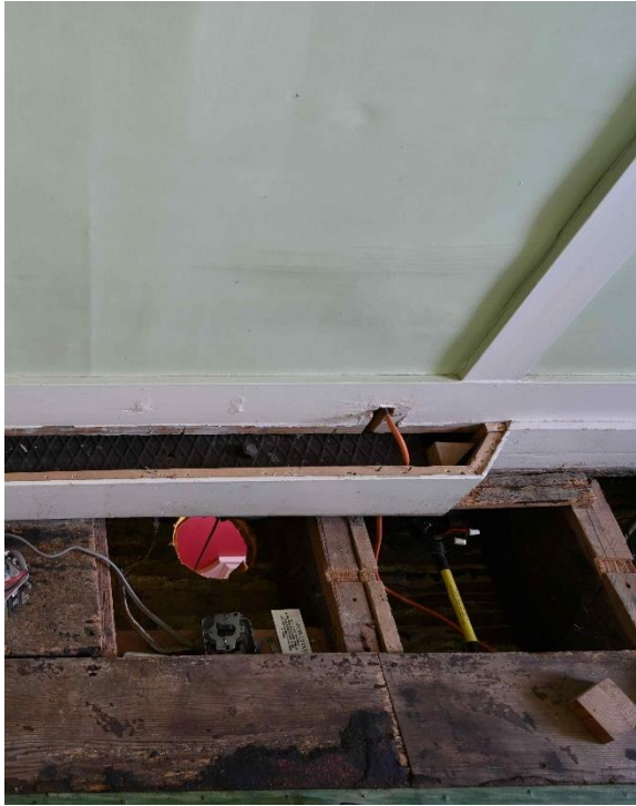
Figure 93: Floor and services inspection - Staff Bathroom SR17
