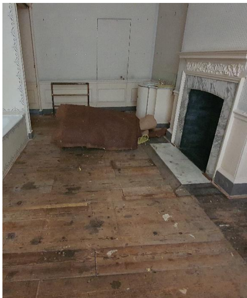
Figure 70: Timber boards, post vinyl removal - Mrs. Hyams Bathroom FR10
