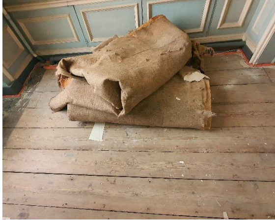
Figure 5: Timber floor, post carpet removal - Blue Bathroom FR01
