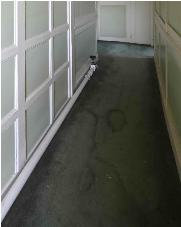
Figure 99: Existing floor finish - Corridor SR18
