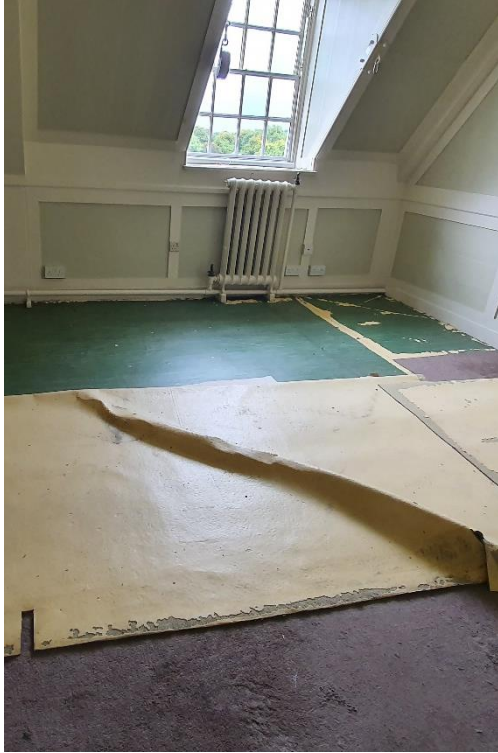
Figure 21: Vinyl floor - Bedroom SR04
