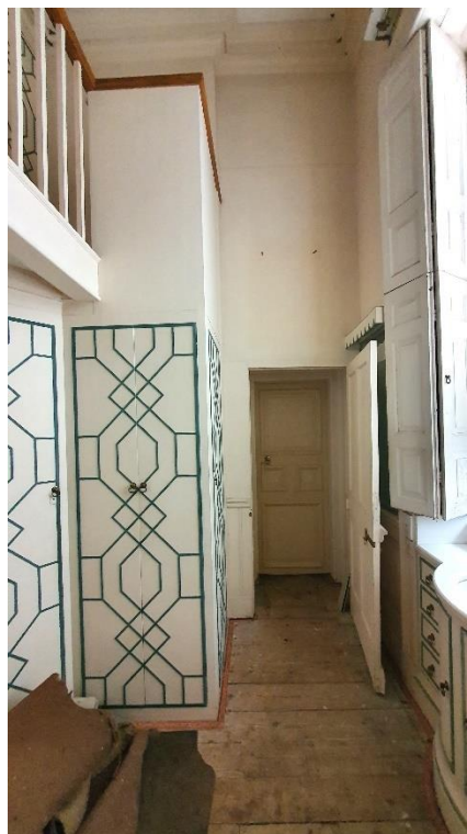
Figure 46: NE internal facade - Mrs. Hyams Dressing Room FR08
