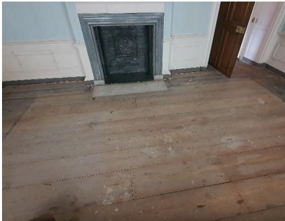
Figure 84: Timber boards, post carpet removal - Mr. Hyams Bedroom FR13
