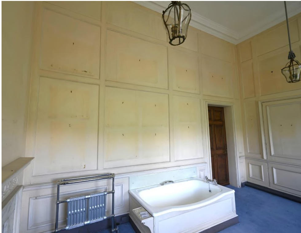
Figure 85: SE internal facade - Mr. Hyams Bathroom FR14
