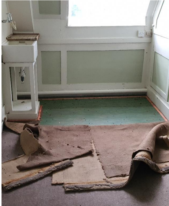
Figure 52: Vinyl under carpet - Linen Room SR09
