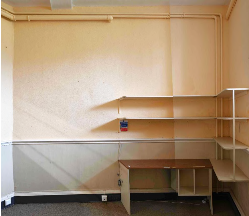
Figure 25: SE internal facade - Office LGR09
