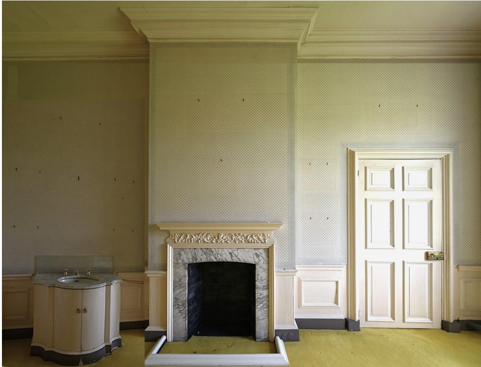
Figure 64: SE internal facade - Mrs. Hyams Bathroom FR10
