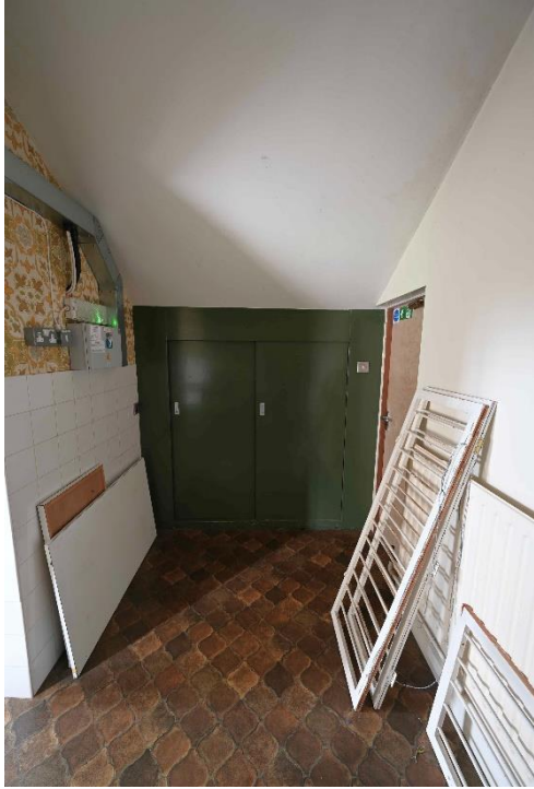
Figure 19: Cupboards in Main Kitchen LGR07
