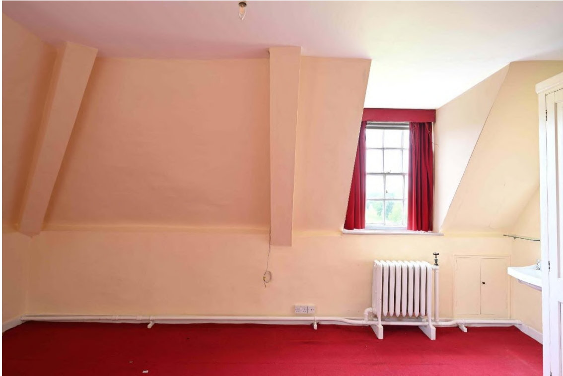
Figure 3: NE internal facade - Staff Bedroom SR01
