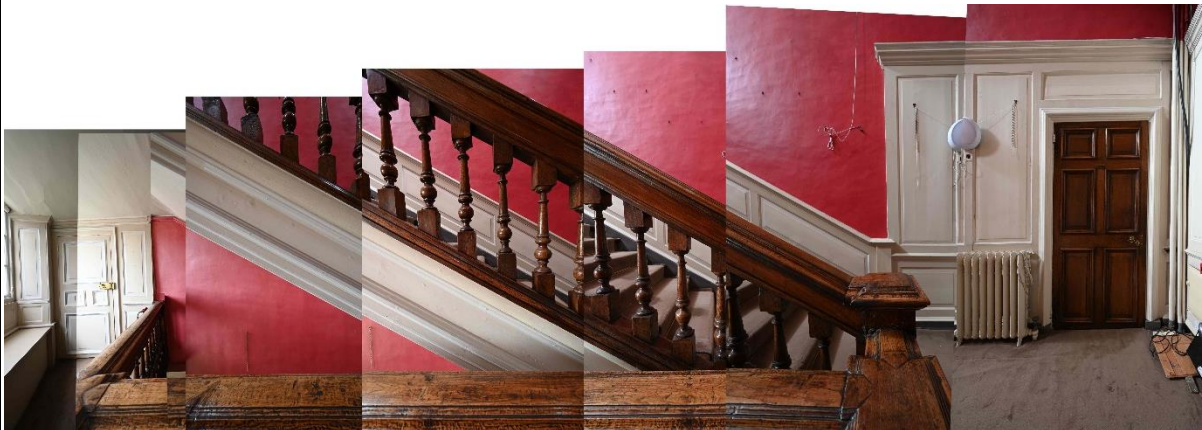
Figure 55: SW internal facade - First Floor - Back Stairs ST01
