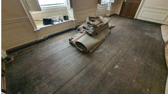
Figure 29: Timber boards, post carpet removal - Pink Bedroom FR05
