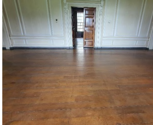
Figure 13: Overview of floorboards - Hall GR02
