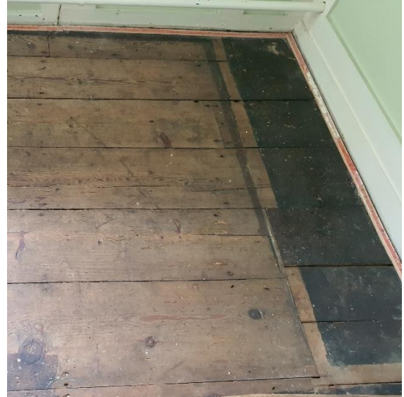
Figure 33: Exposed timber floor post carpet removal - Dressing Room SR06
