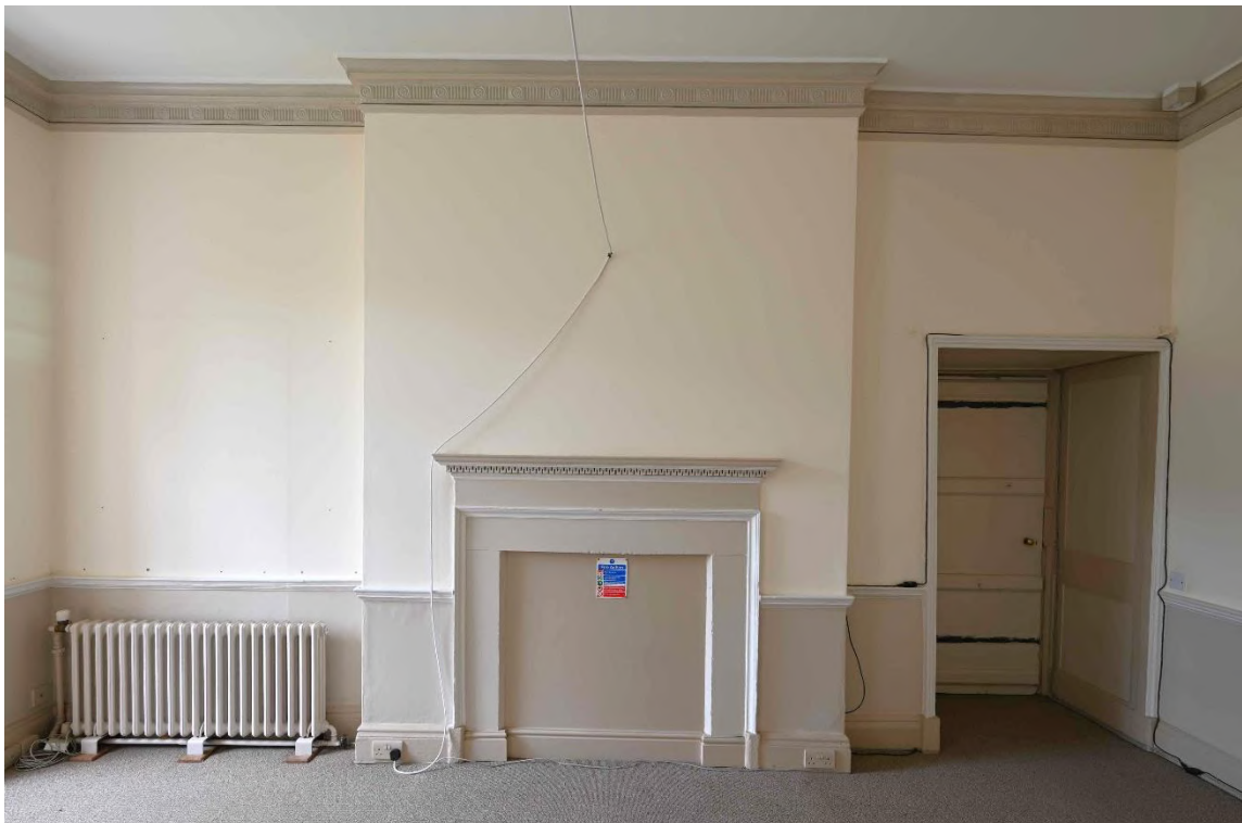
Figure 8: SW internal facade - Staff Room LGR05
