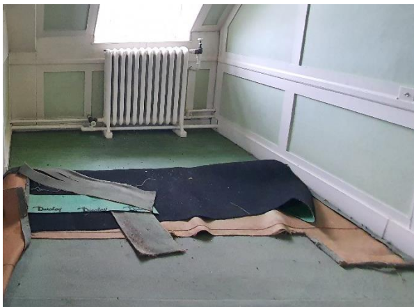
Figure 46: Removal of carpet and exposing vinyl - Green Bedroom SR08
