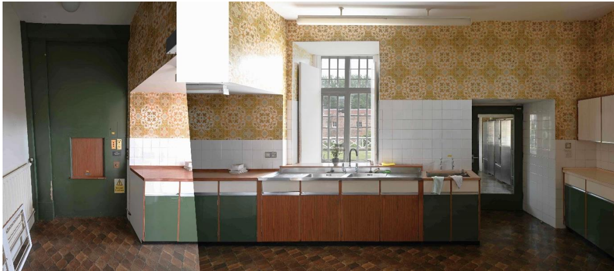
Figure 15: SE internal facade - Main Kitchen LGR07
