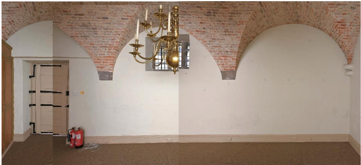
Figure 2: SW internal facade - Games room LGR02
