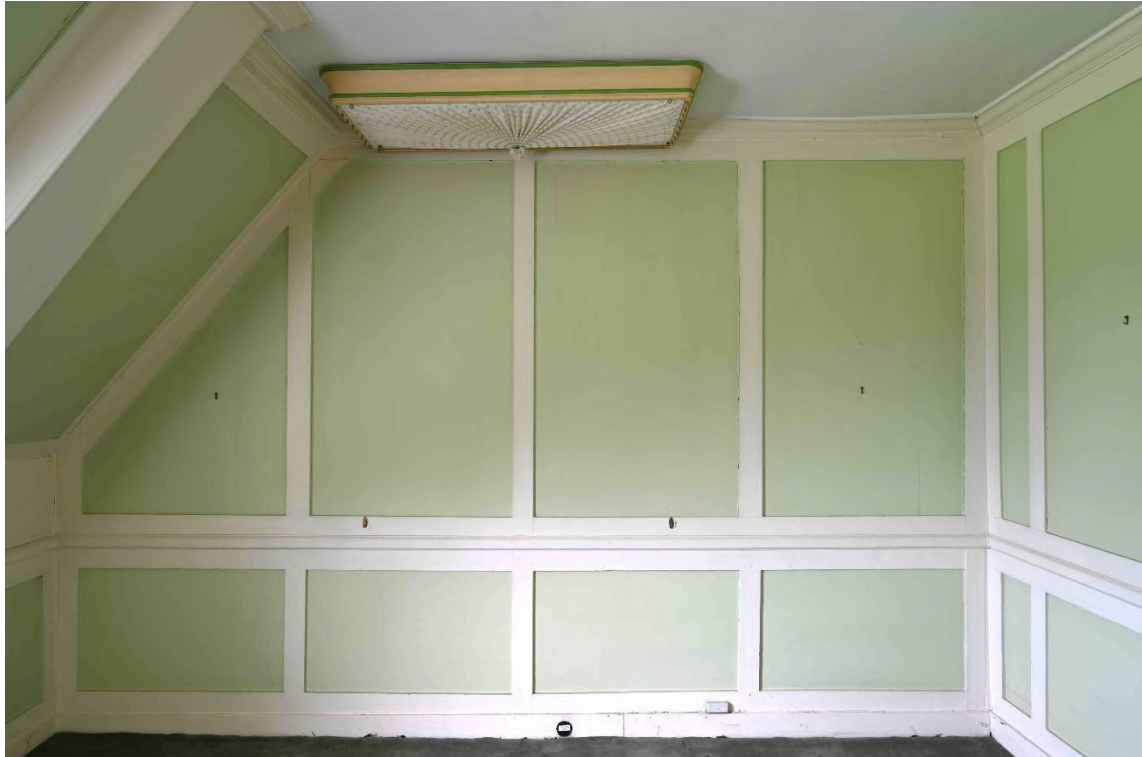
Figure 22: SE internal facade - Bedroom SR05
