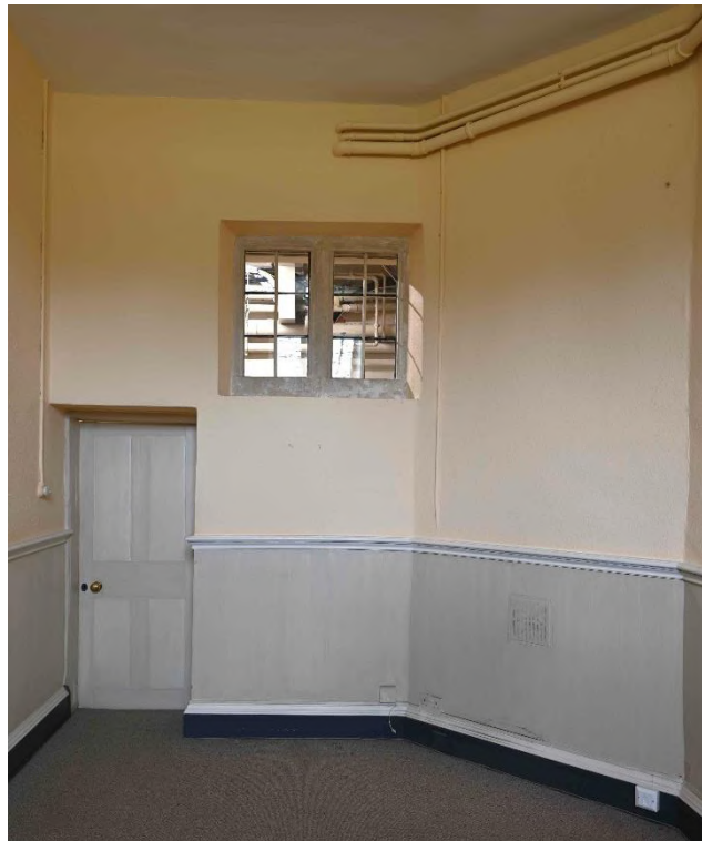
Figure 28: NE internal facade - Office LGR09
