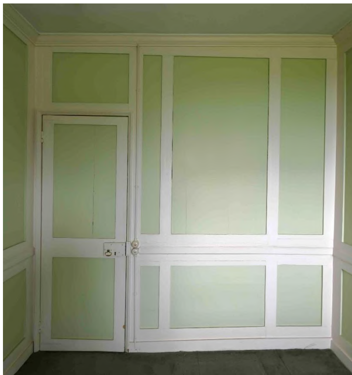
Figure 29: SW internal facade - Dressing Room SR06
