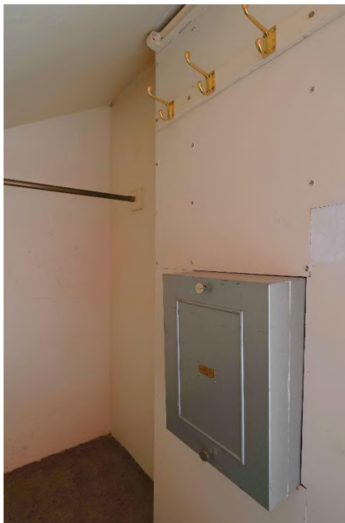
Figure 55: Cloak Cupboard – North Hall Toilet GR09
