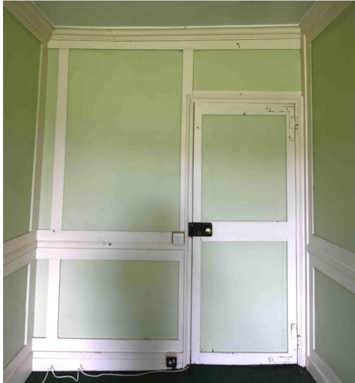
Figure 84: SE internal facade - Staff Bathroom SR16
