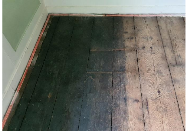
Figure 27: Exposed timber floor post carpet removal - Bedroom SR05
