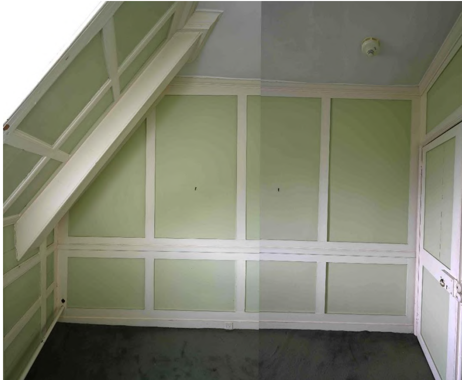
Figure 28: SE internal facade - Dressing Room SR06
