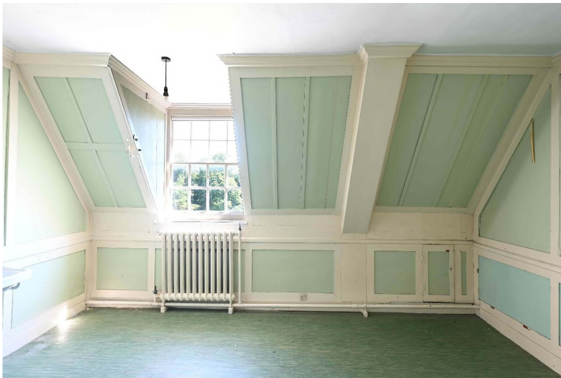
Figure 14: NE internal facade - Storeroom SR03
