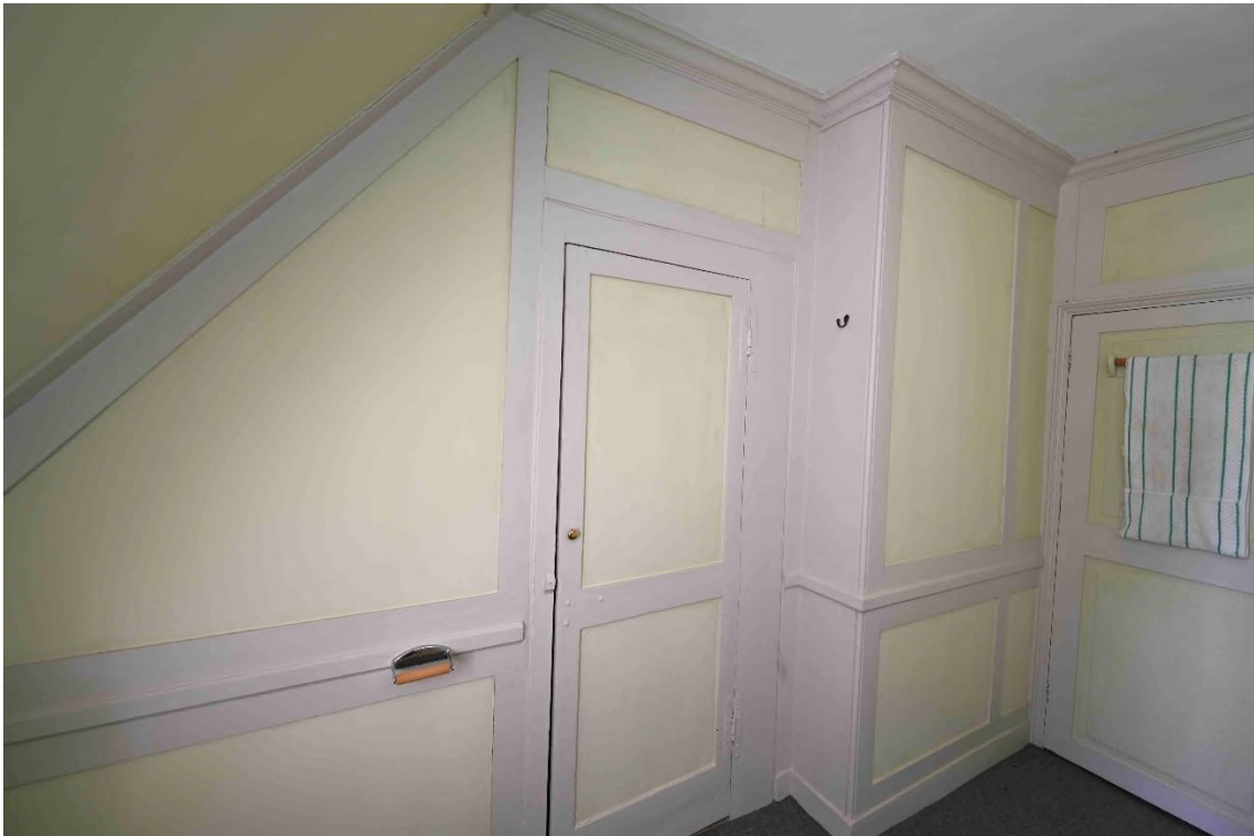
Figure 83: NE internal facade - Staff Bathroom SR15
