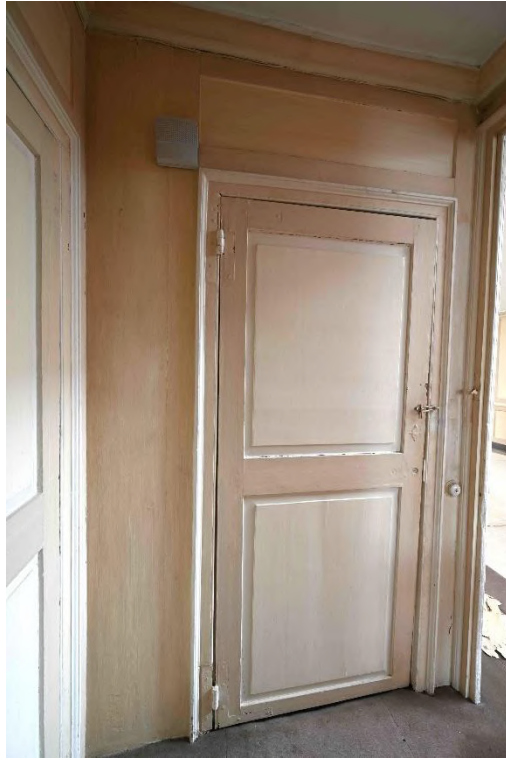
Figure 109: NW internal facade - Hallway SR22
