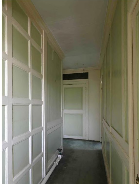
Figure 97: NW internal facade - Corridor SR18
