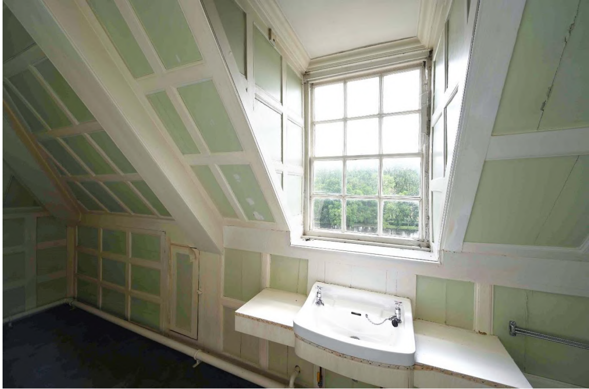
Figure 34: SE internal facade - Bathroom SR07
