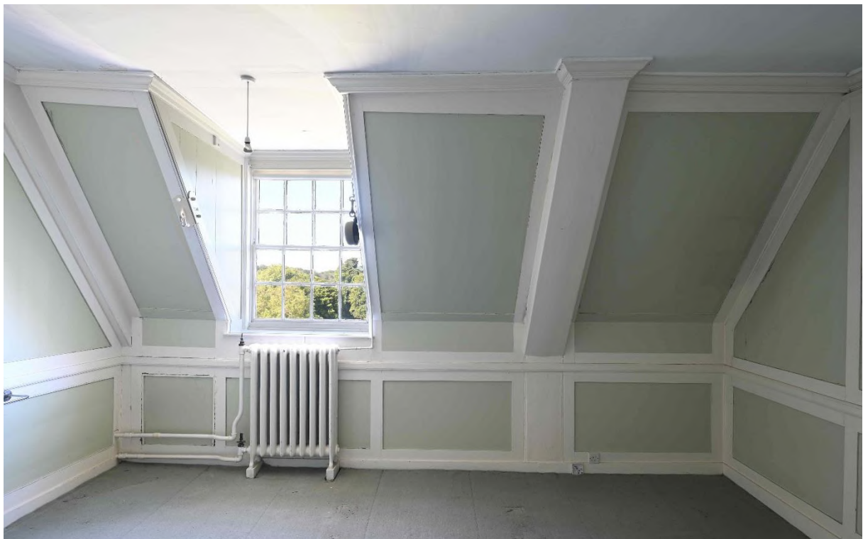
Figure 61: SW internal facade - Storeroom SR11
