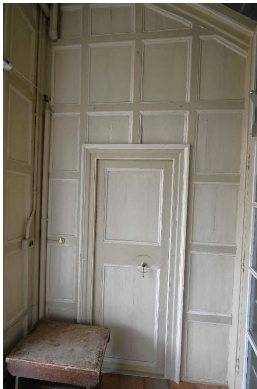
Figure 12: SW internal facade - Lobby LGR06
