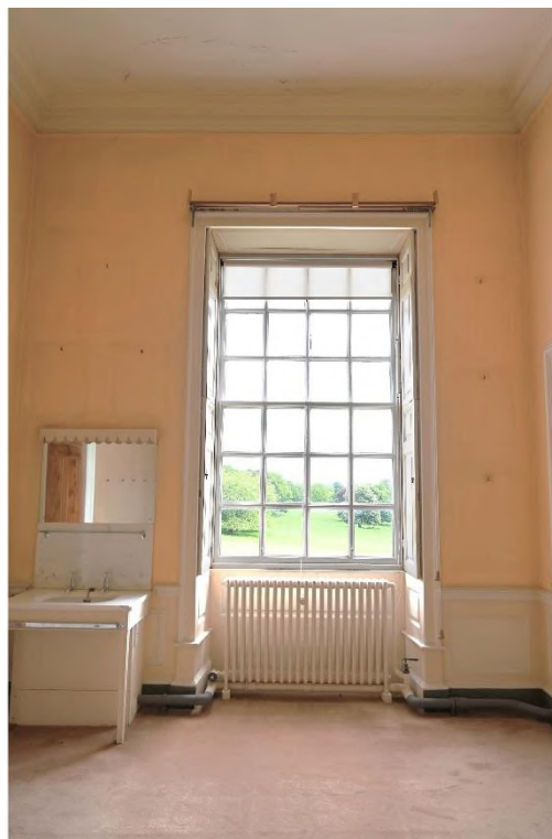
Figure 23: NE internal facade- Chinese Bathroom FR04
