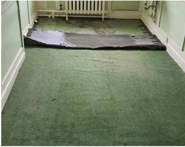
Figure 88: Floor, vinyl under carpet - Staff Bathroom SR16
