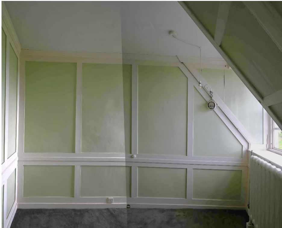
Figure 30: NW internal facade - Dressing Room SR06
