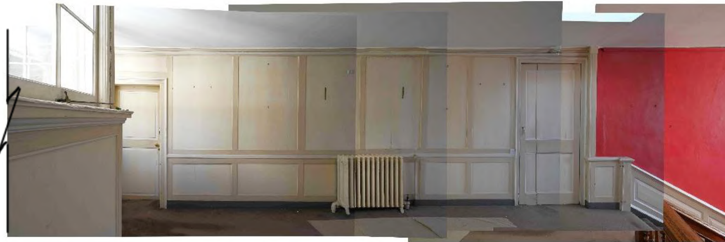
Figure 56: NE internal facade - Central Landing SR10
