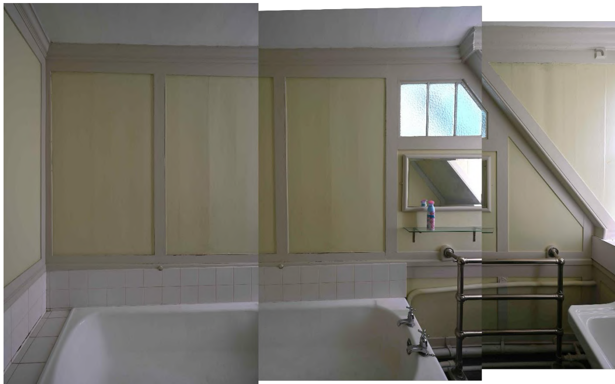
Figure 81: SW internal facade - Staff Bathroom SR15
