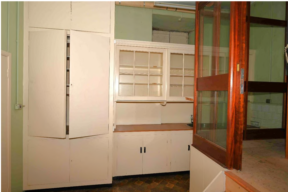
Figure 35: SW internal facade - Projection Room LGR11
