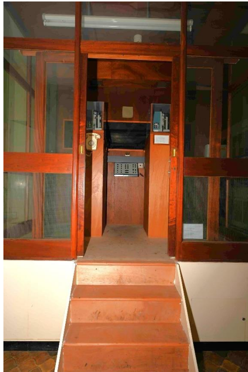
Figure 36: NW internal facade - Projection Room LGR11
