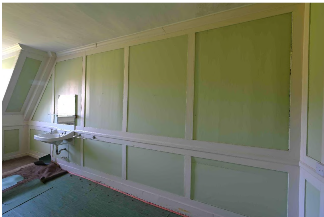
Figure 92: NE internal facade - Staff Bathroom SR17
