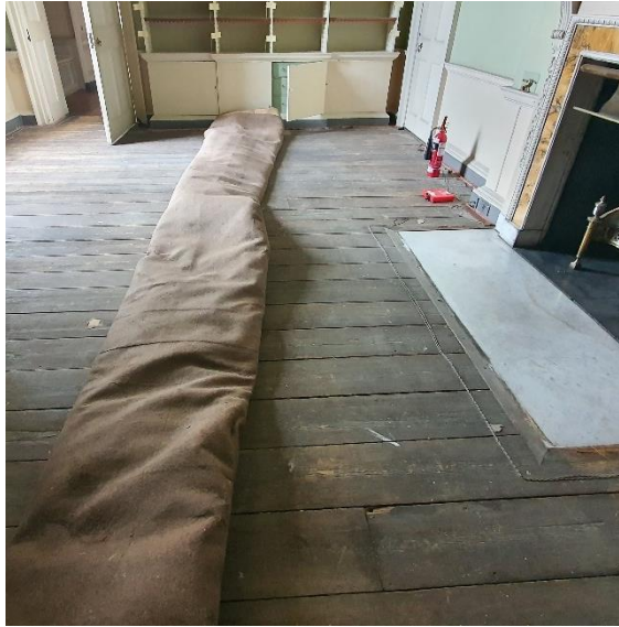
Figure 5: Overview of floorboards - Library GR01
