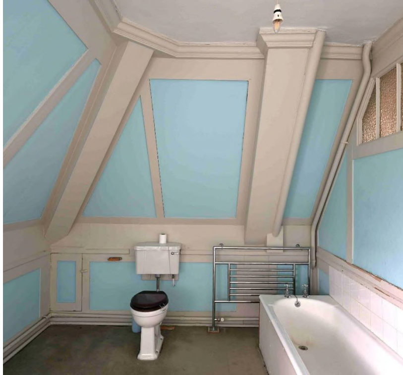
Figure 77: NW internal facade – Staff Bathroom SR14
