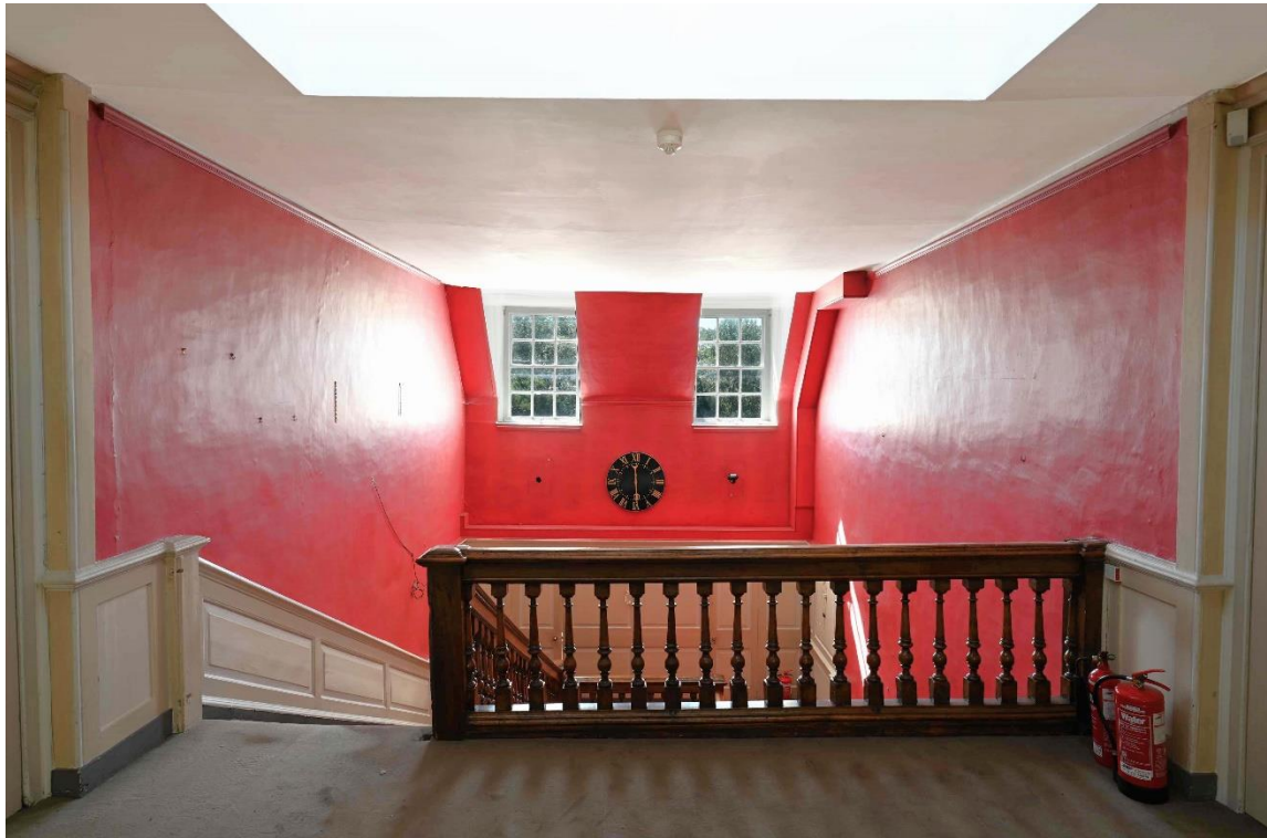
Figure 53: SE internal facade - Central Landing SR10
