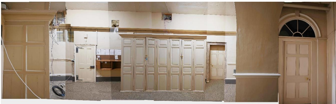
Figure 32: NE internal facade - LGR10
