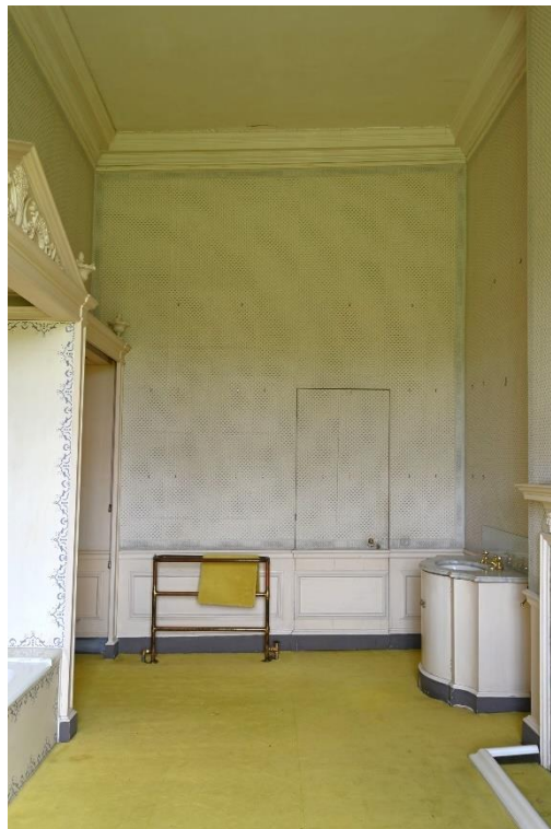
Figure 67: NE internal facade - Mrs. Hyams Bathroom FR10
