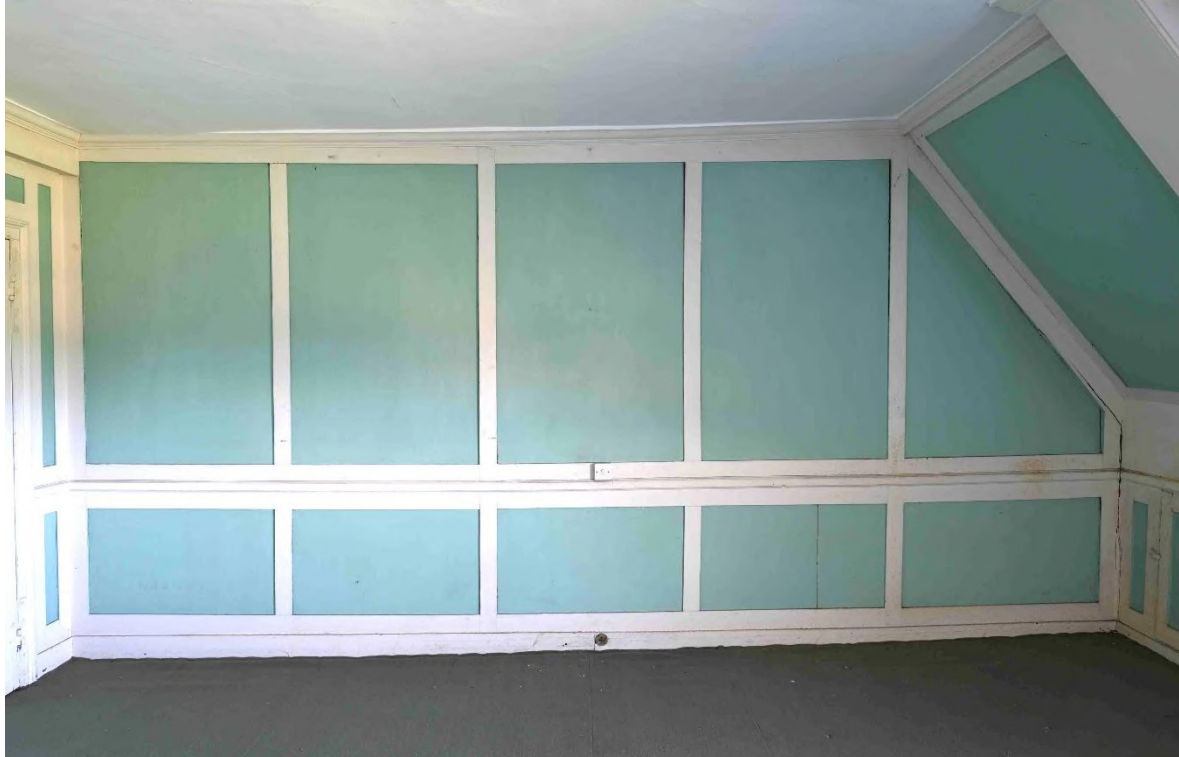
Figure 64: SE internal facade - Restoration Room SR12
