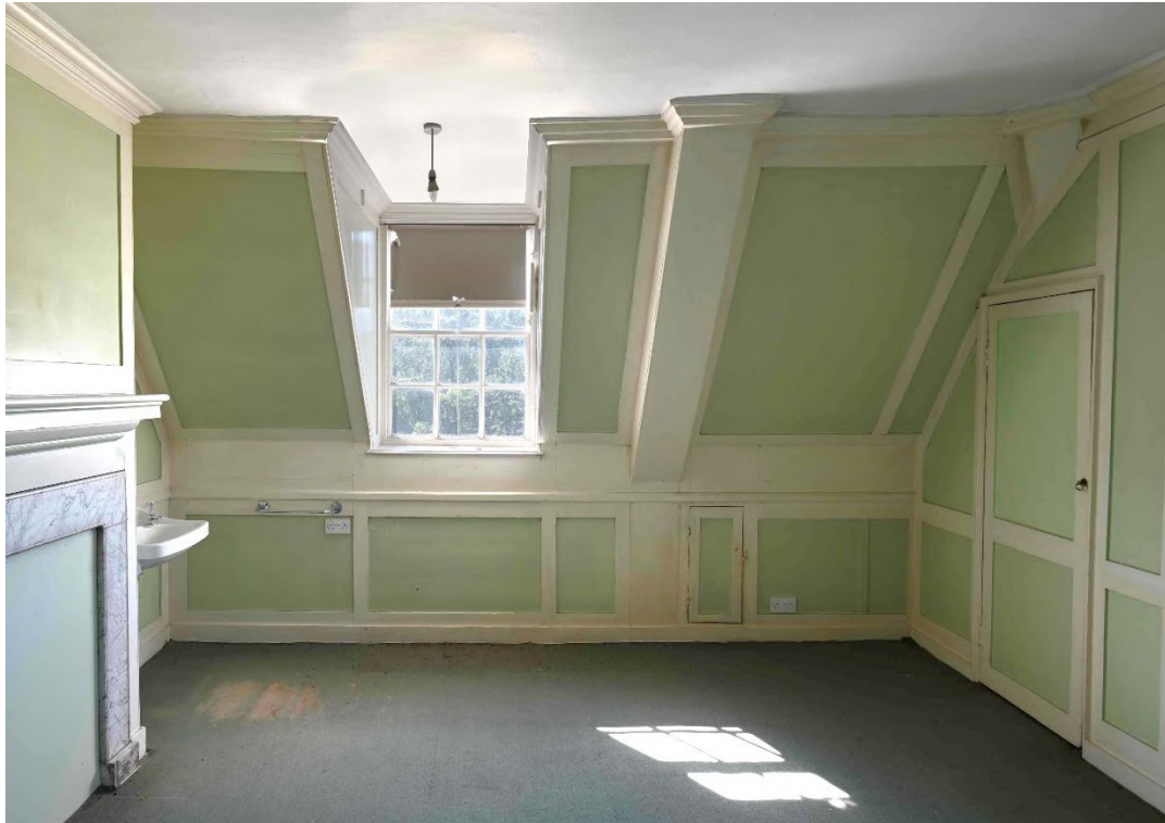
Figure 40: SE internal facade - Green Bedroom SR08
