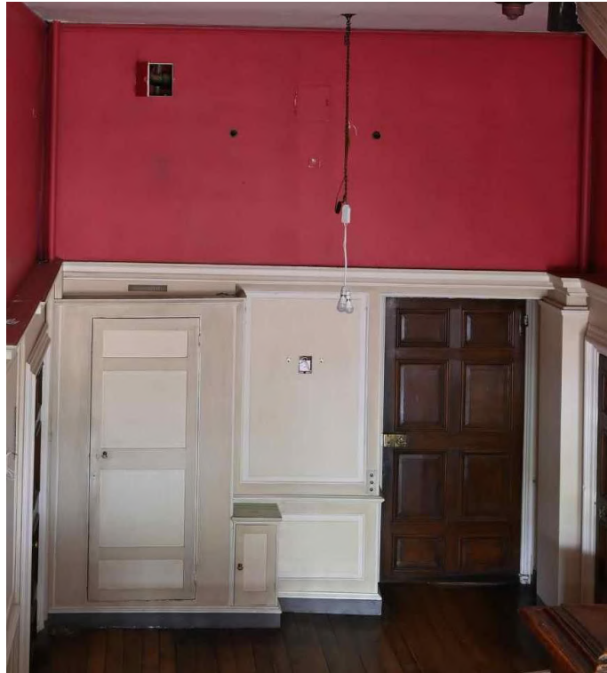
Figure 60: NW internal facade - Ground Floor - Back Stairs ST01
