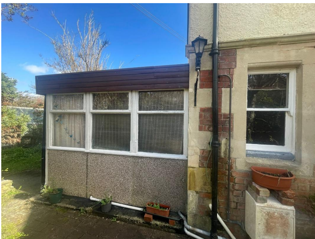
Photograph 2: Rear conservatory western elevation
