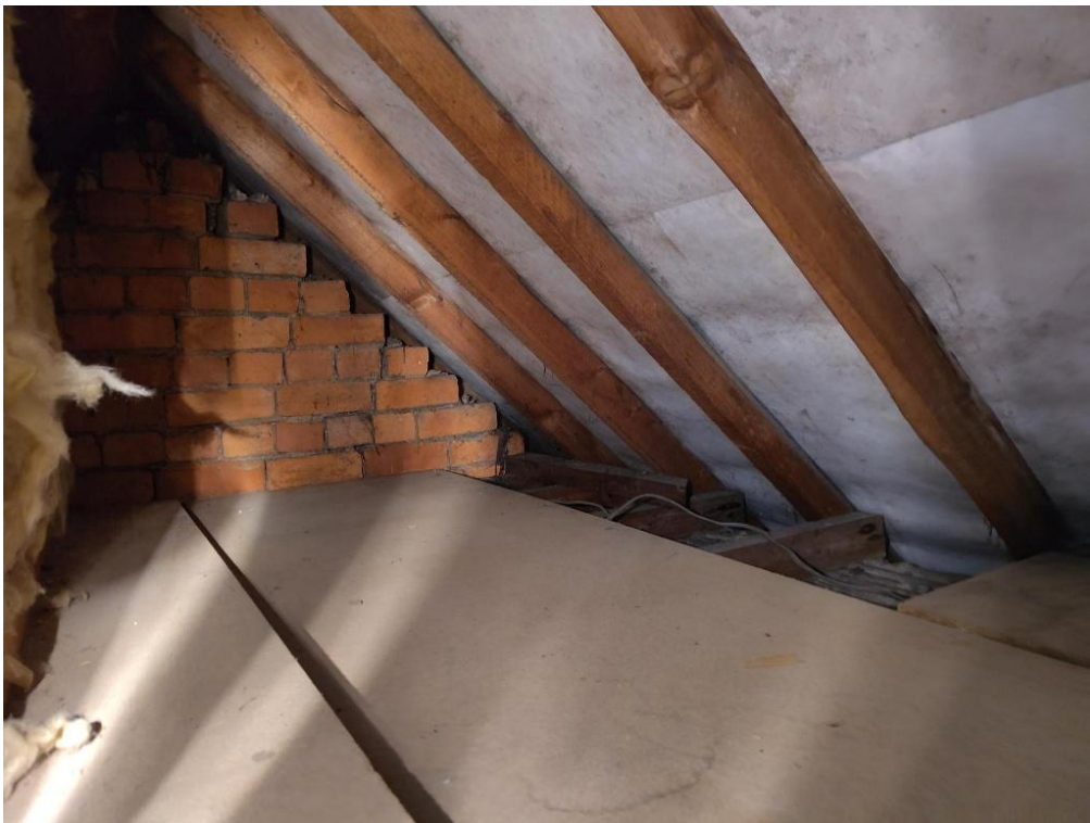
Photograph 6: Eaves at front section of property
