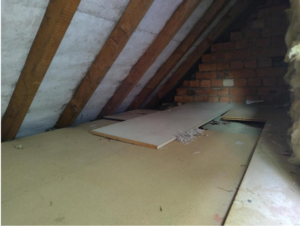
Photograph 5: Eaves at front section of property
