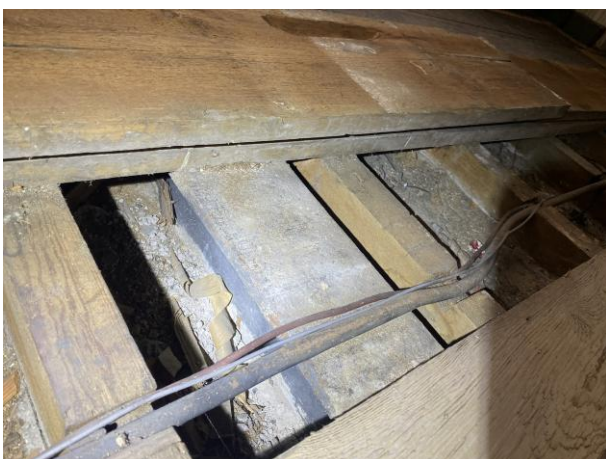
Rolled steel joist / clay & straw pugging insulation
