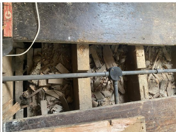
Clay & straw pugging insulation conceals dropped void
