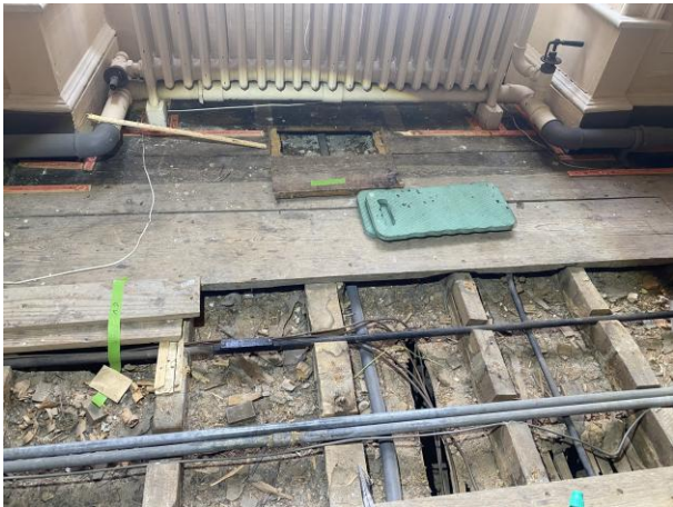
Clay & straw pugging insulation conceals dropped void
