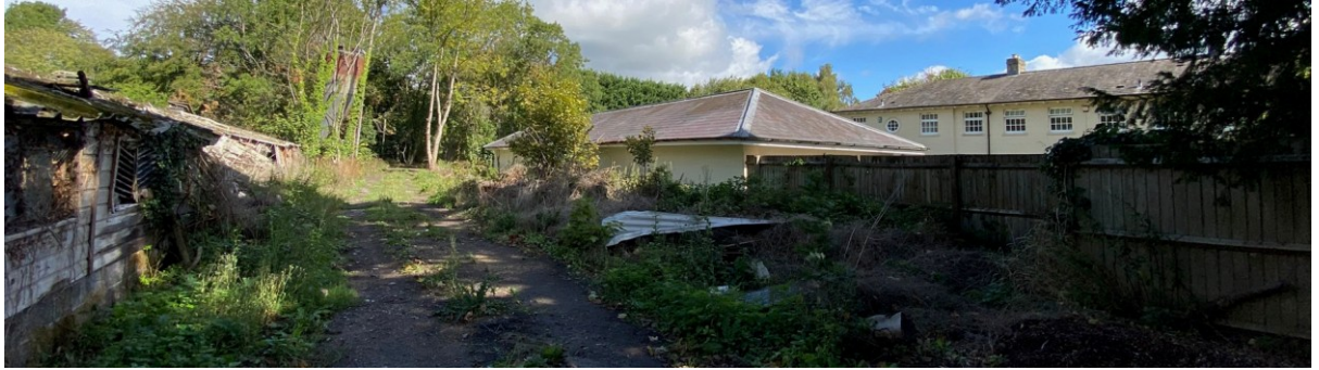
Site visit image of existing shed facing North
