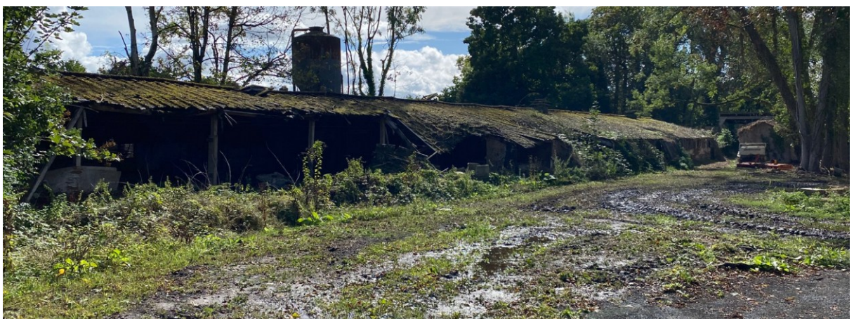
Site Visit image of existing shed facing Southeast
