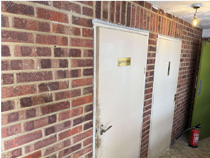
Existing wc access
