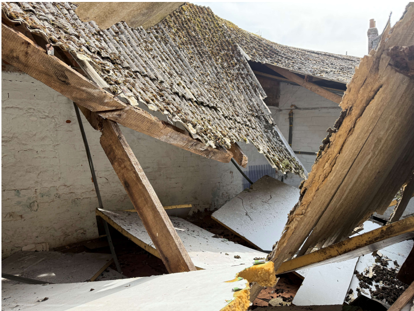
Store to be demolished
