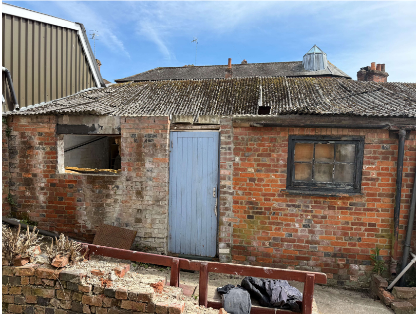
Store to be demolished
