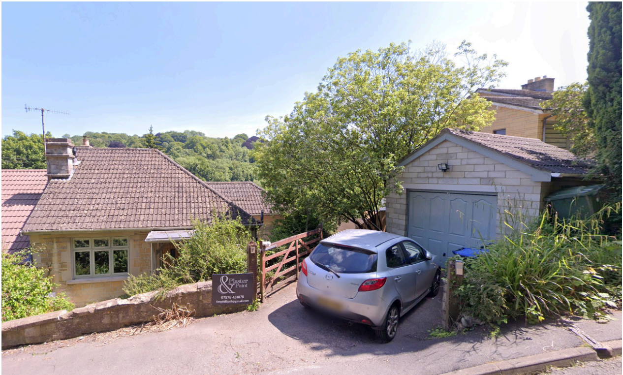
Image 3: View of the front elevation from Crowe Hill
