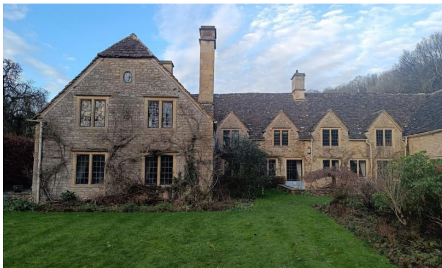
Figure 1: The Weavers House - rear elevation
