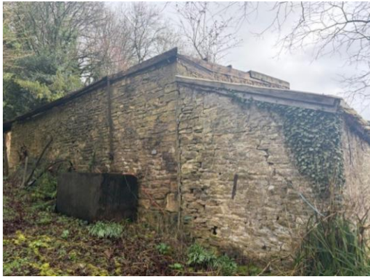
Photograph 4: West facing view
