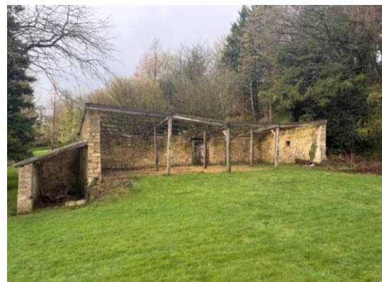
Photograph 3: East facing view
