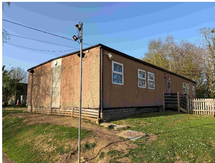
Fig 1. Pre-fab unit (to be removed).
