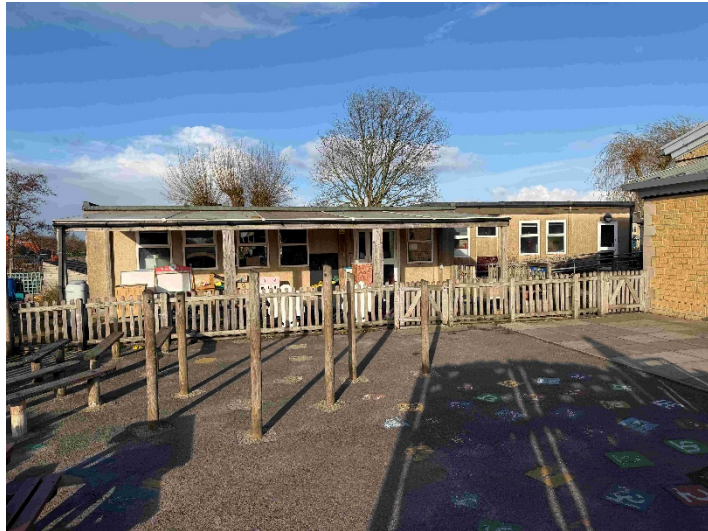
Fig 1. Pre-fab unit (to be removed).
