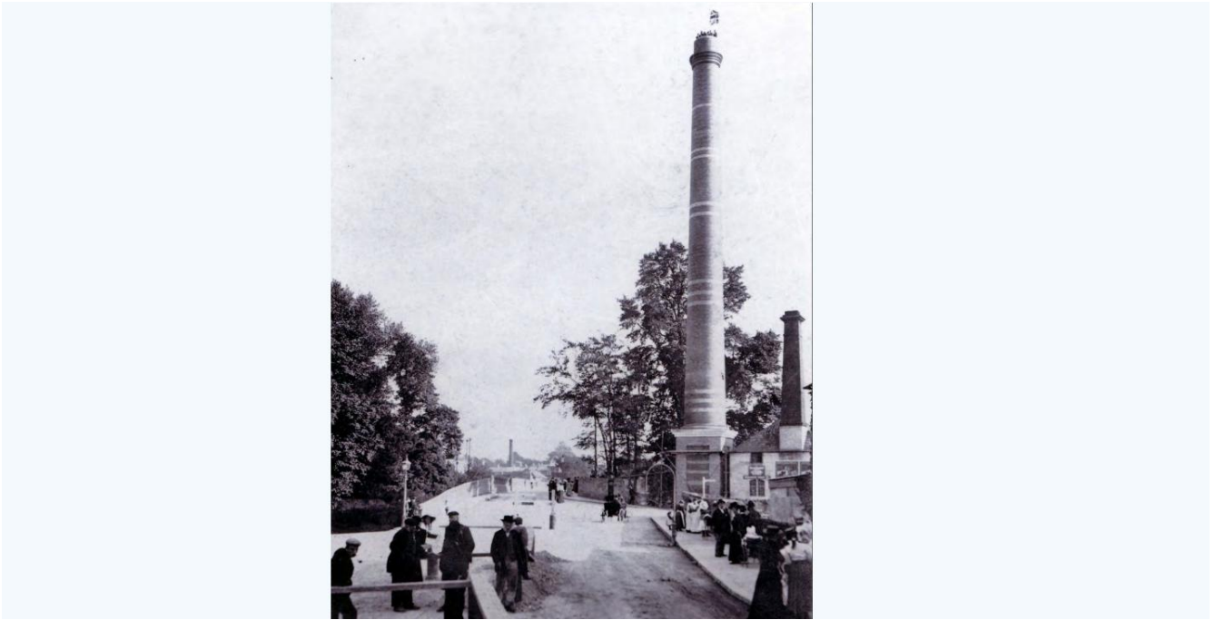
Figure 6: Image from the applicant's Design Note showing the chimney potentially from the 19 th century. The existing chimney is significantly truncated, now finishing just above the second set of triple banding from the base of the plinth.
