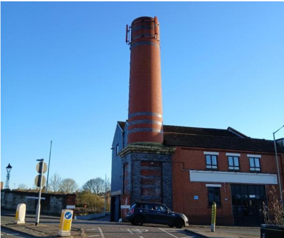
Figure 7: Image taken on a site inspection in March 2026.
