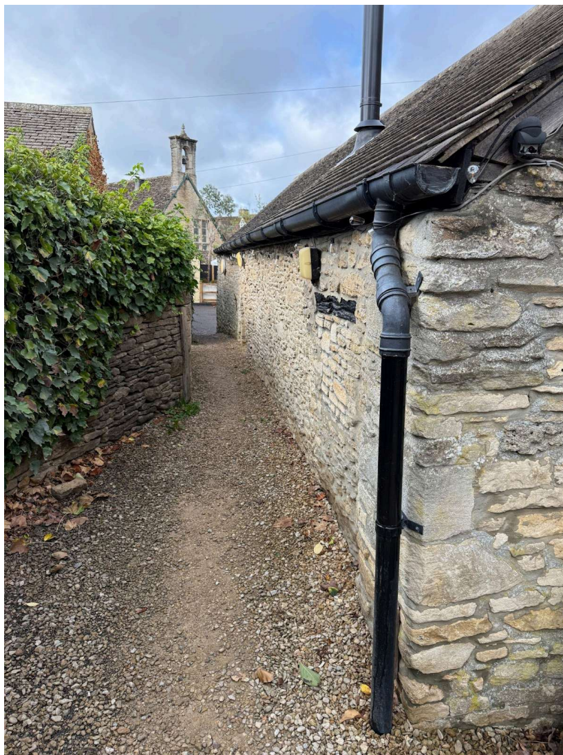
Picture 6 - North wall guttering to Dining Area
