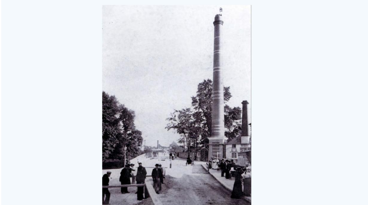
Figure 6: Image of the chimney at the site, potentially from the late 19 th century.
