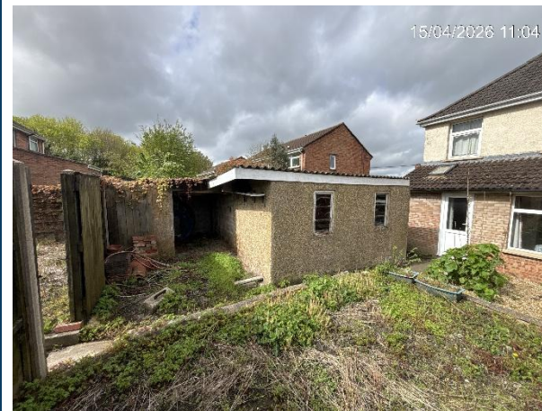
Photo 3: Eastern elevation of the garage (B1) and lean-to section.
