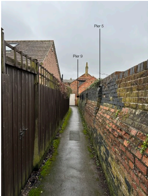
View adjacent to Pier 5
