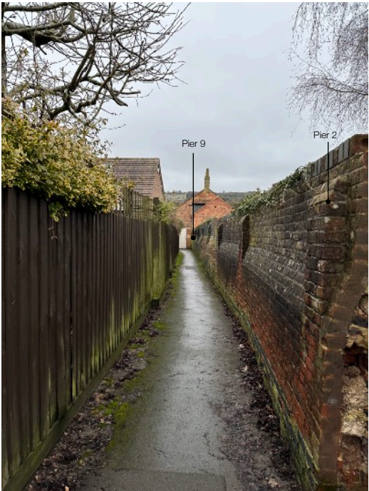
View adjacent to Pier 2
