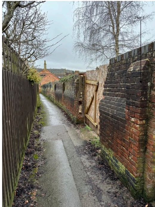
View adjacent to Pier 1
