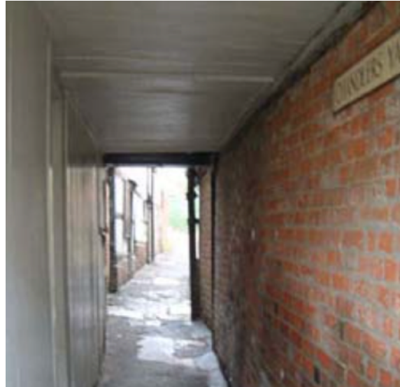
Chandlers Yard passage from High Street, extract from Marlborough Conservation Area Statement
