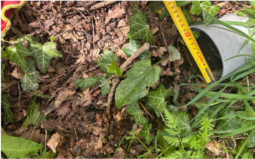
Existing Pipe Outfall to Dry Pond
