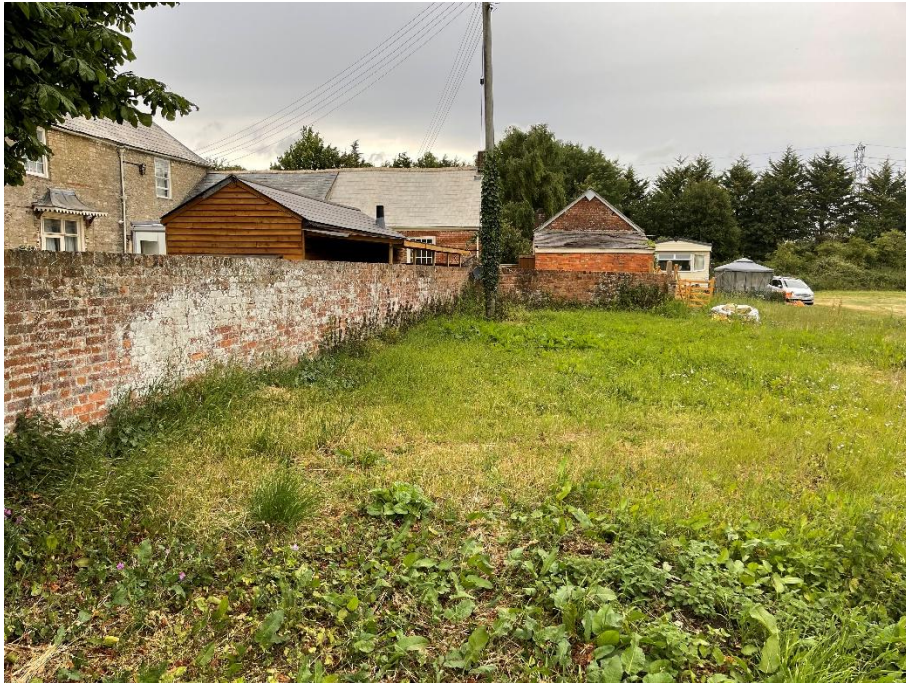
Figure 1 Site area showing continuous wall.
