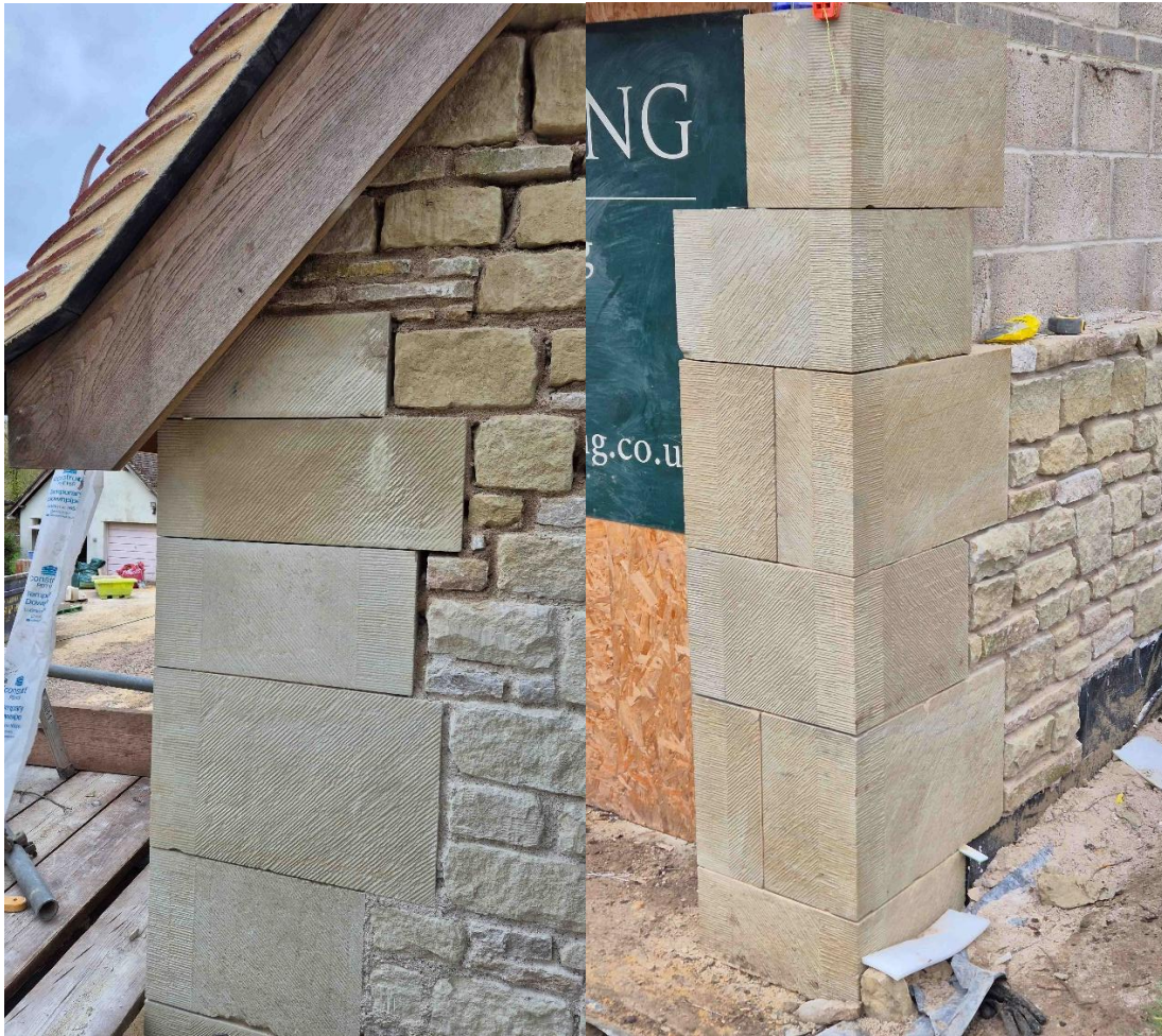
Garage Chicksgrove stone quoins and rubble wall
