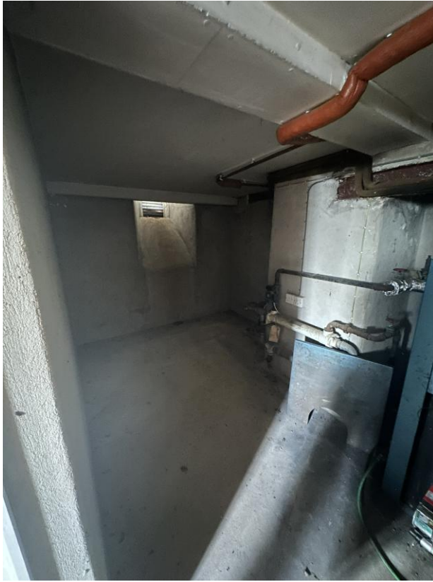
Photograph 7. Internal view of basement showing the metal vent.
