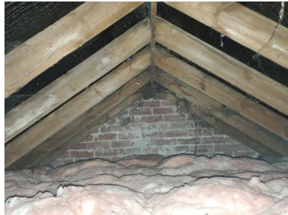
Photo 10: Internal view of northern loft void.
