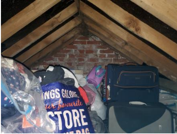
Photo 7: Internal view of southern loft void.
