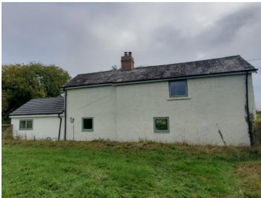
Photo 3: The west facing elevations of the residential dwelling.
