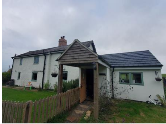
Photo 2: The east facing elevations of the residential dwelling.
