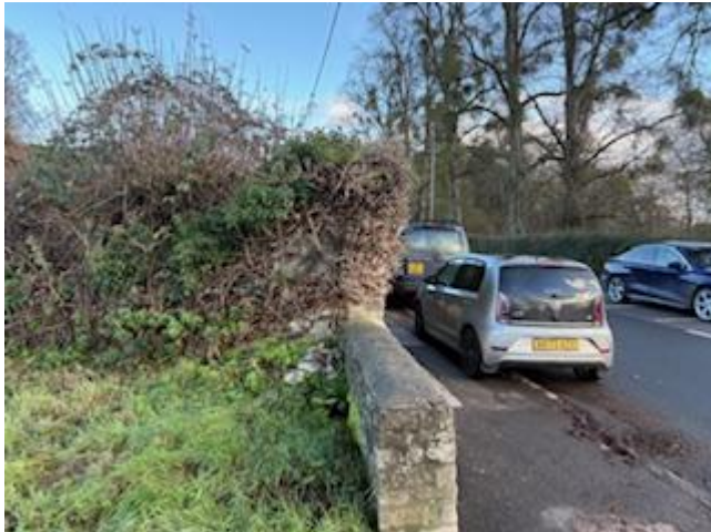
Figure 3: Existing wall in visibility splay.
