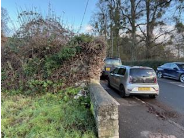
Figure 3: Existing wall in visibility splay.
