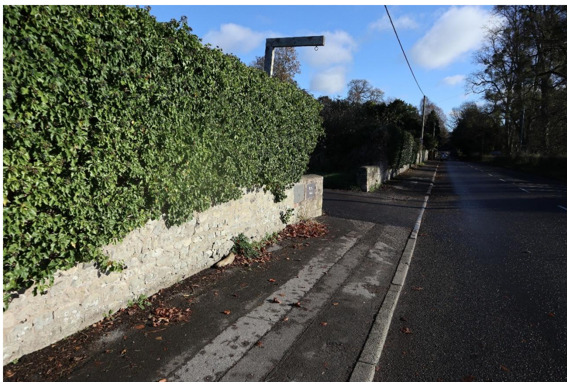
Figure 5.2 View facing west along Boreham Road, showing the section of rebuilt stone wall located at the north-western edge of the Bishopstrow Conservation Area
