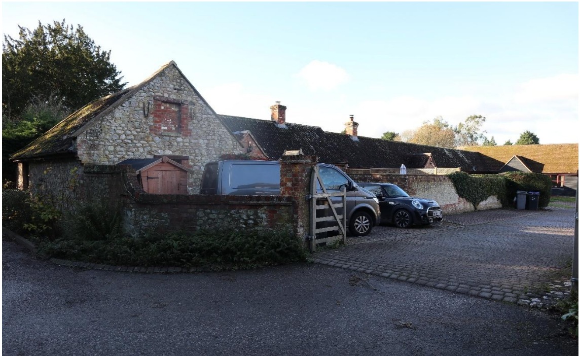
Figure 5.14 An example of some of the converted ancillary buildings at Bishopstrow Home Farm.
