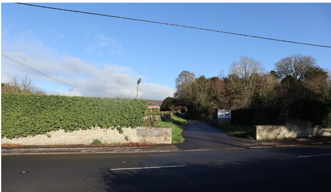
Figure 5.3 A portion of the Boreham Road boundary wall located at the access drive to Home Farm
