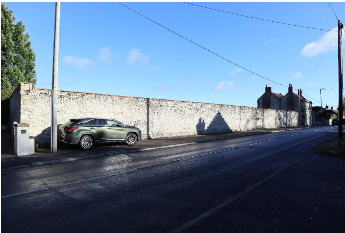
Figure 5.8 A portion of the Boreham Road boundary wall to the west of The Cotes (Grade II). Visible is the unused and boarded up historic opening at the eastern end of the wall (below).
