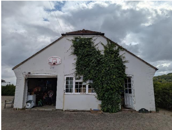
Photo 5 – external view of B2, cottage west elevation
