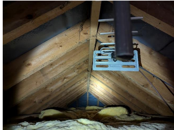
Photo 6 – Internal view of loft void in B2, cottage
