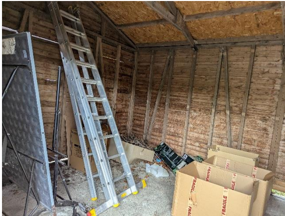
Photo 11 – internal view of B4, timber garage used for storage
