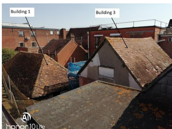
Plate 9. Southern and western elevations of Buildings 1 and 3.
