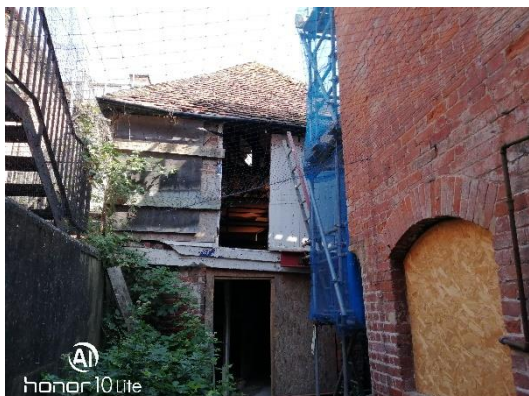
Plate 1. Southern elevation of Building 1.
