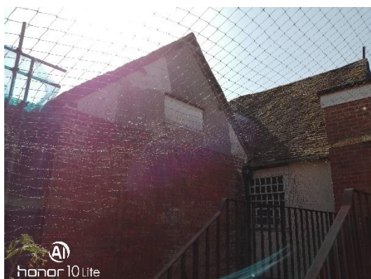
Plate 7. Western elevation of Building 3.
