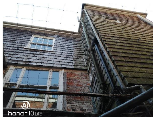
Plate 10. Western elevation of Building 5.
