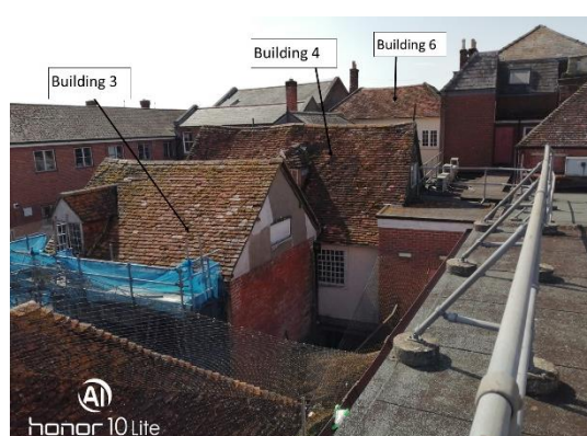
Plate 8. Northern roof faces of Building 3, Building 4 and Building 6.
