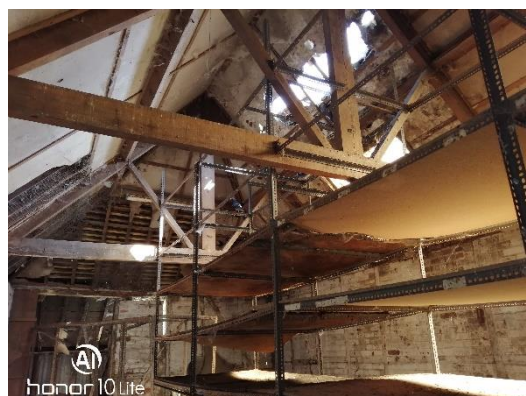
Plate 2. Internal upper floor of Building 1.
