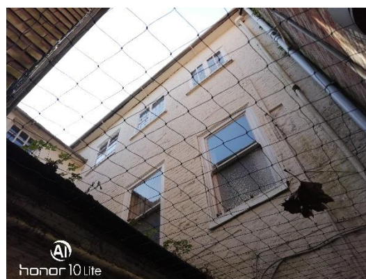
Plate 12. Northern elevation of Building 6.
