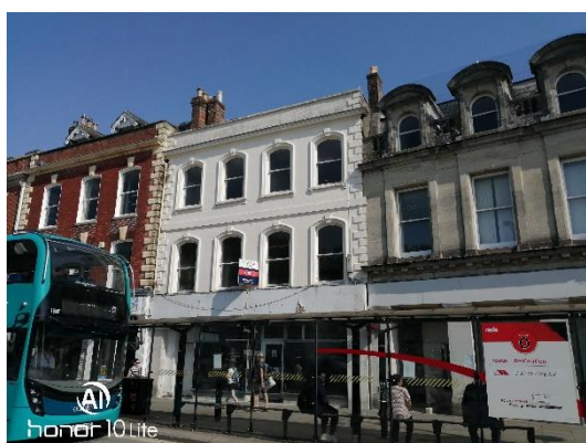
Plate 11. Southern elevation of Building 6.
