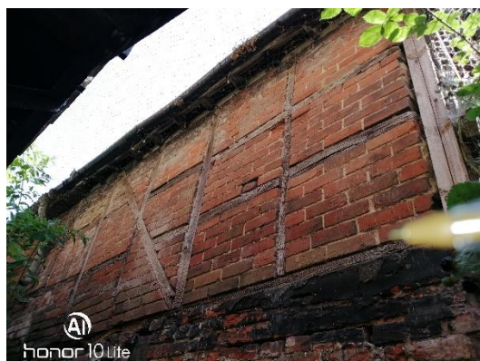
Plate 3. Western elevation of Building 1.
