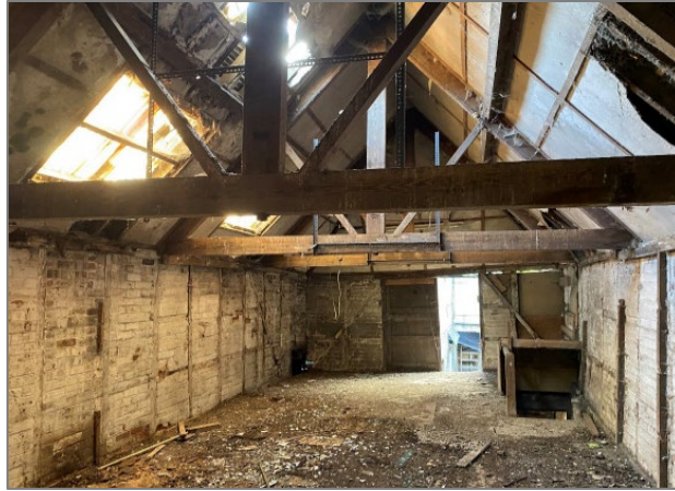
Figure 5 – Existing first floor stable building
