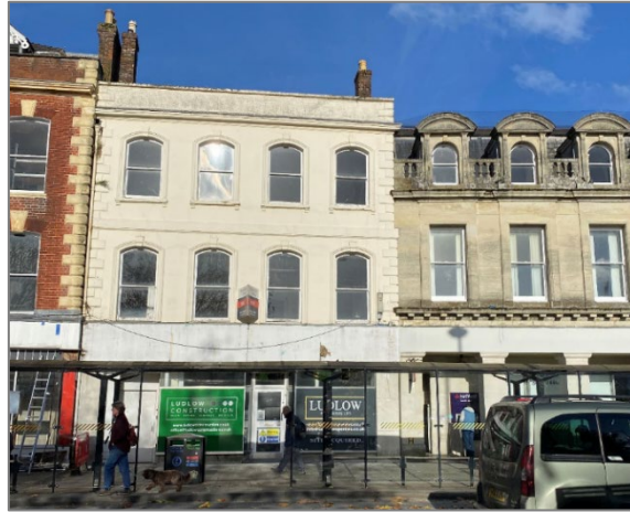
Figure 2 – Existing front façade
