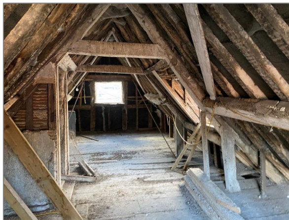
Figure 4 – Attic level in oldest core
