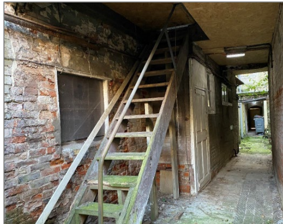
Figure 3 - Existing alleyway off Blue Boar Row
