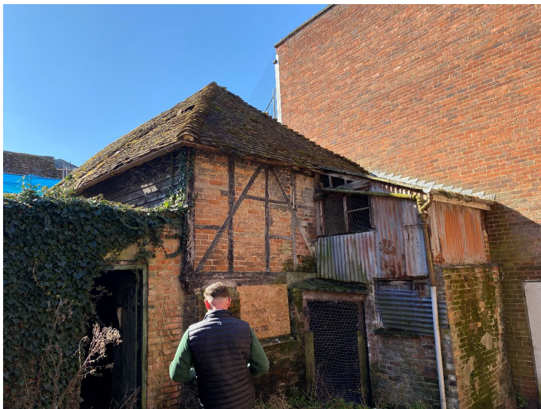
Figure 46: northern end of the structure, modern additions and modern next door structure hard against the slightly older building with its hipped roof. Timber siding visible on the long elevation.
