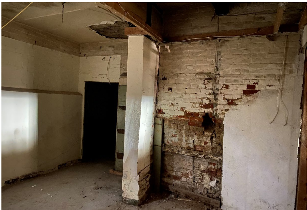
Figure 22: Central area and location of historic stair – ancient newel stair retained above this area.
