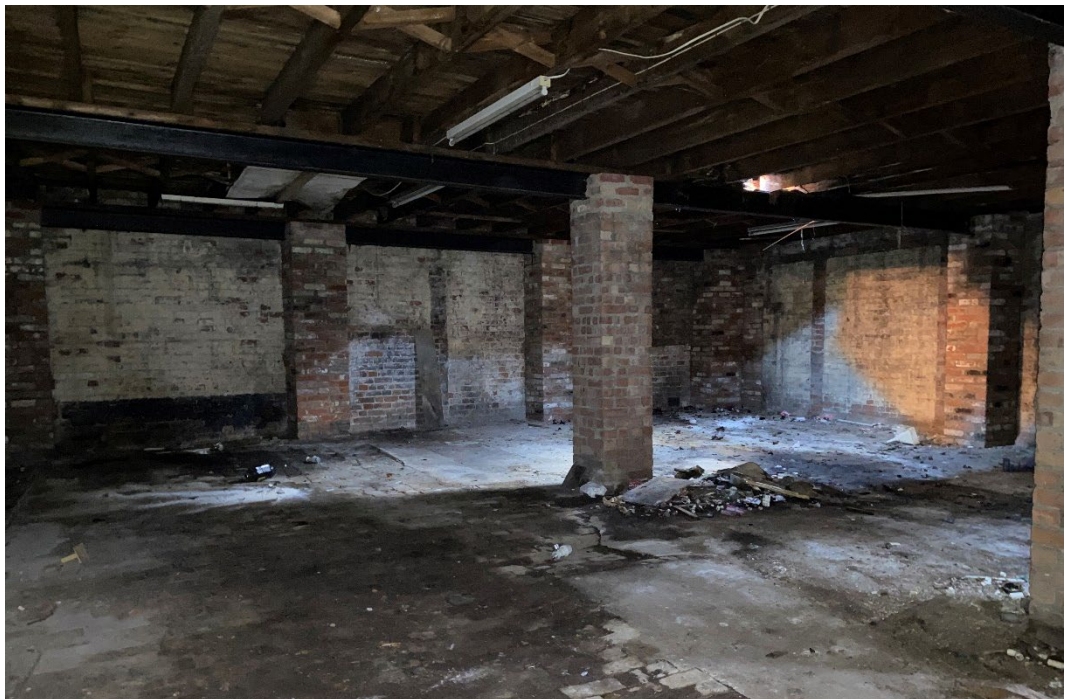
Figure 30: The north east structure, heavily altered and rebuilt with flat roof.
