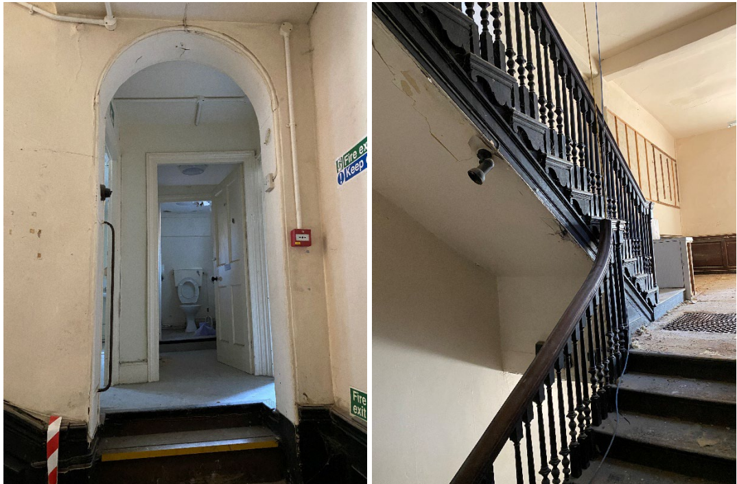
Figure 16-17: (left) view from half landing into rear portion through arched opening and (right) view of main stair balustrade at first floor level.
