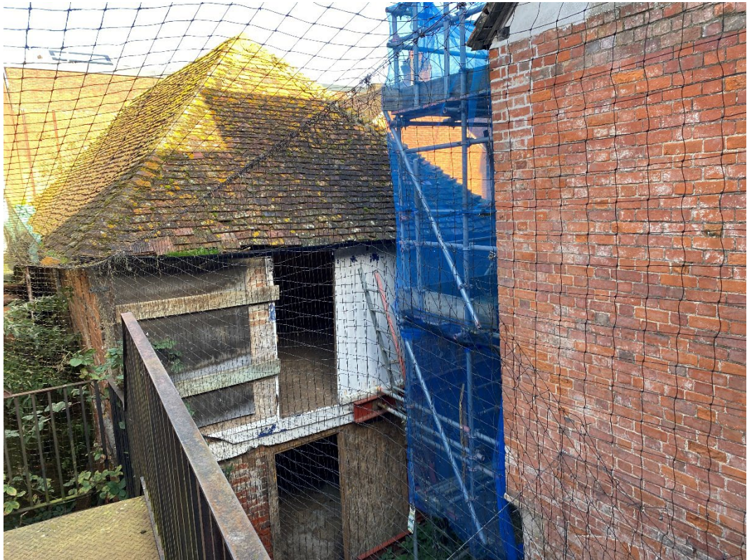
Figure 27: the late 18 th century structure to the rear, 19 th century store on the right.
