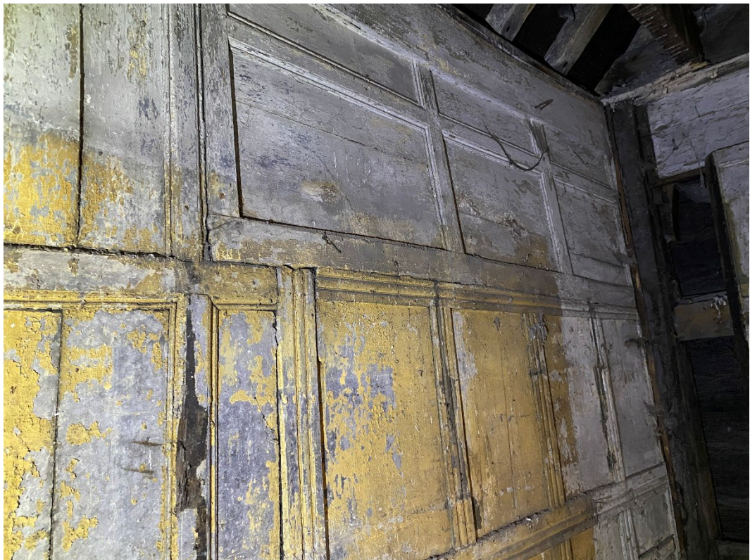
Figure 4: panelling fixed to the walls in the first floor room over the alley but showing clear adaptations in upper part.
