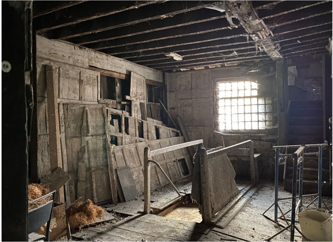
Figure 23: Room in central structure, historic panelling stacked an in situ. Early 18 th century window, modern stair down to side alley in centre.
