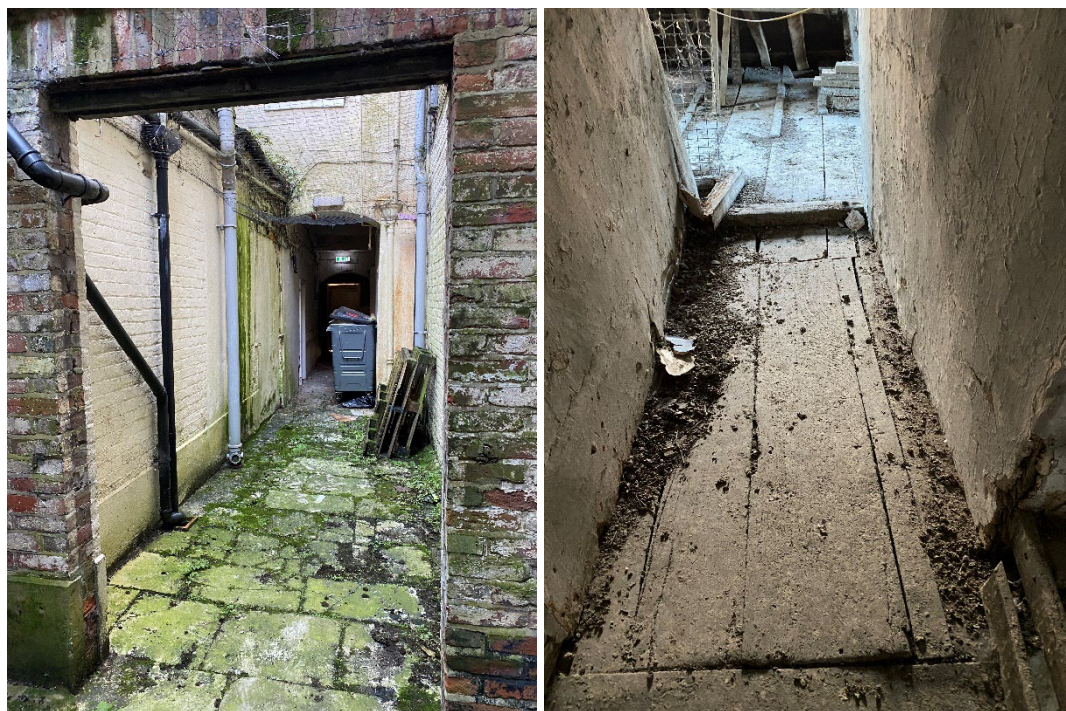
Figure 34-35: flag stones within the side passage, well squared and set; wide floor boards, perhaps oak or elm, within the central structure.
