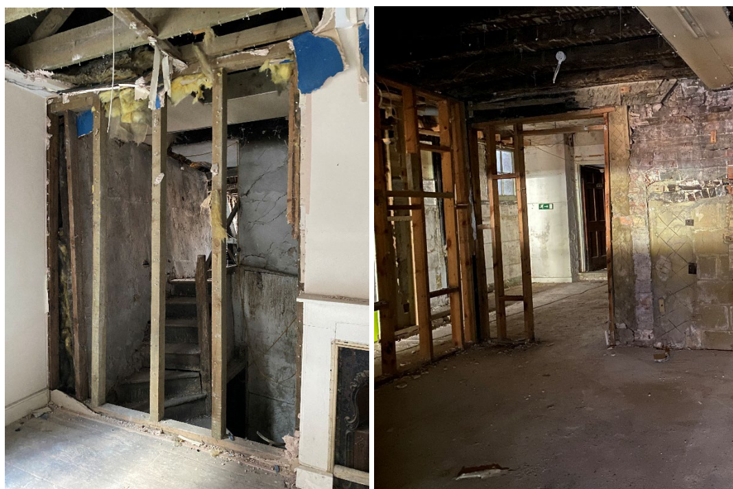
Figure 42-43: areas of extant fabric removal in modern period where fire rated partitions will be installed between units 6/7 in the front of the building and unit 2.
