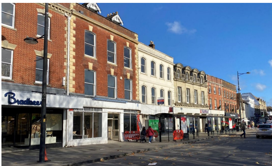
Figure 2: Blue Boar Row from the southwest, no.46/47 the white building in the centre.
