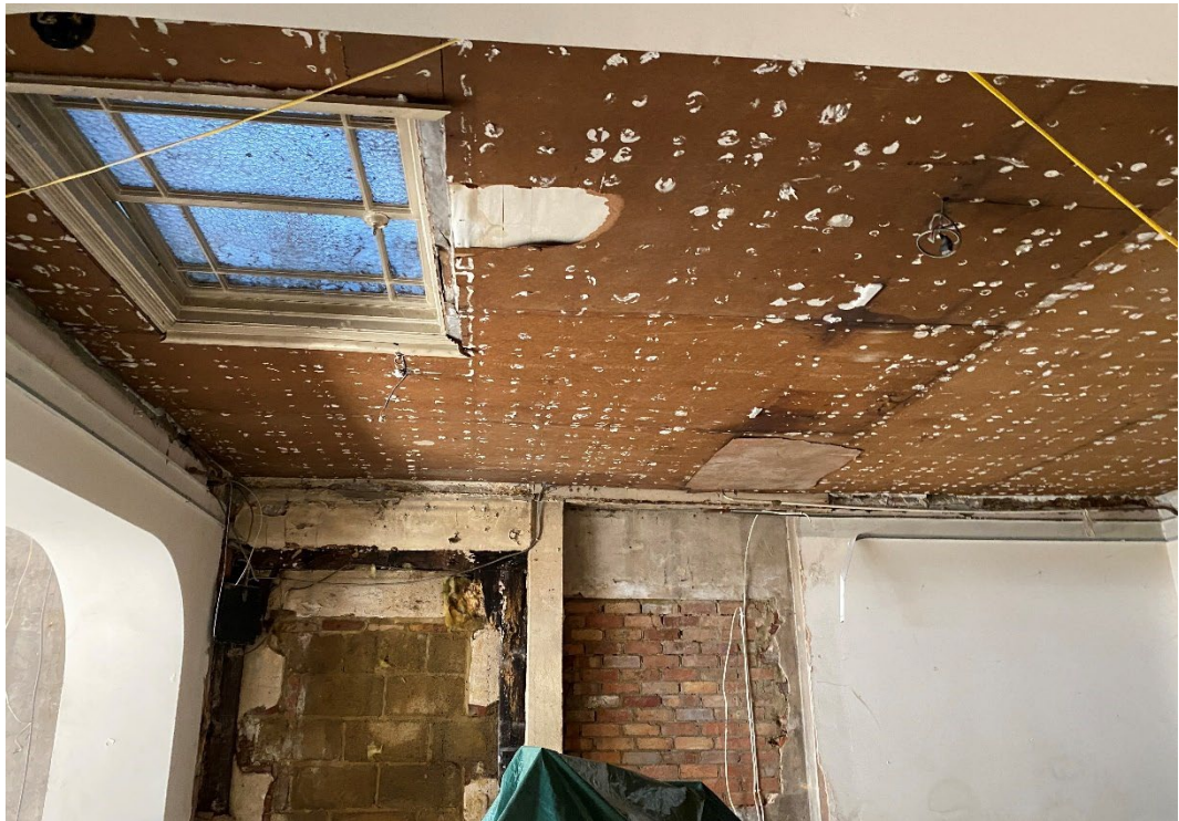
Figure 12: Ground floor central space, blocked door lower left equates to historic entry from side alley. Mid 19 th century skylight over former passage.
