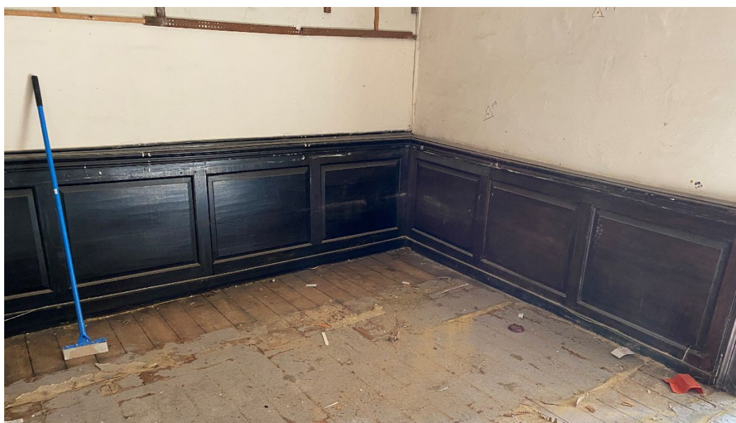
Figure 37: Dado level panelling on first floor landing, note narrower floor boards.
