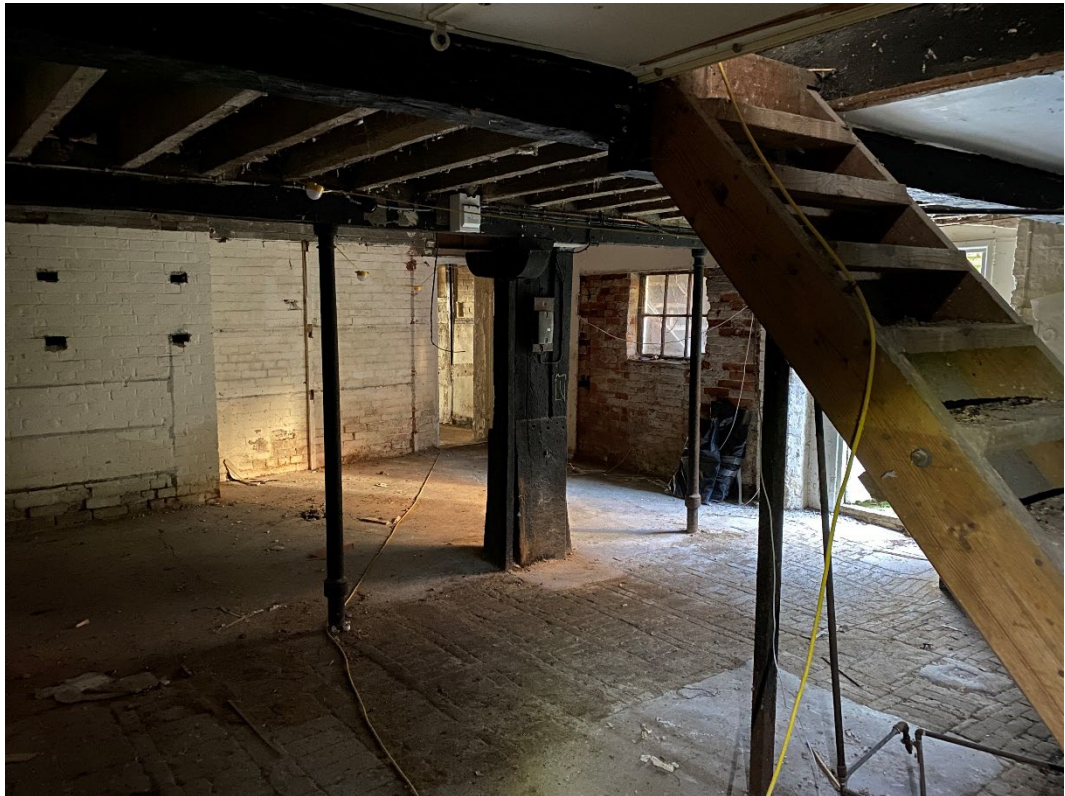
Figure 21: ground floor area under older and 19 th century structures. Some historic flooring survives but partitions and structural lines eroded.
