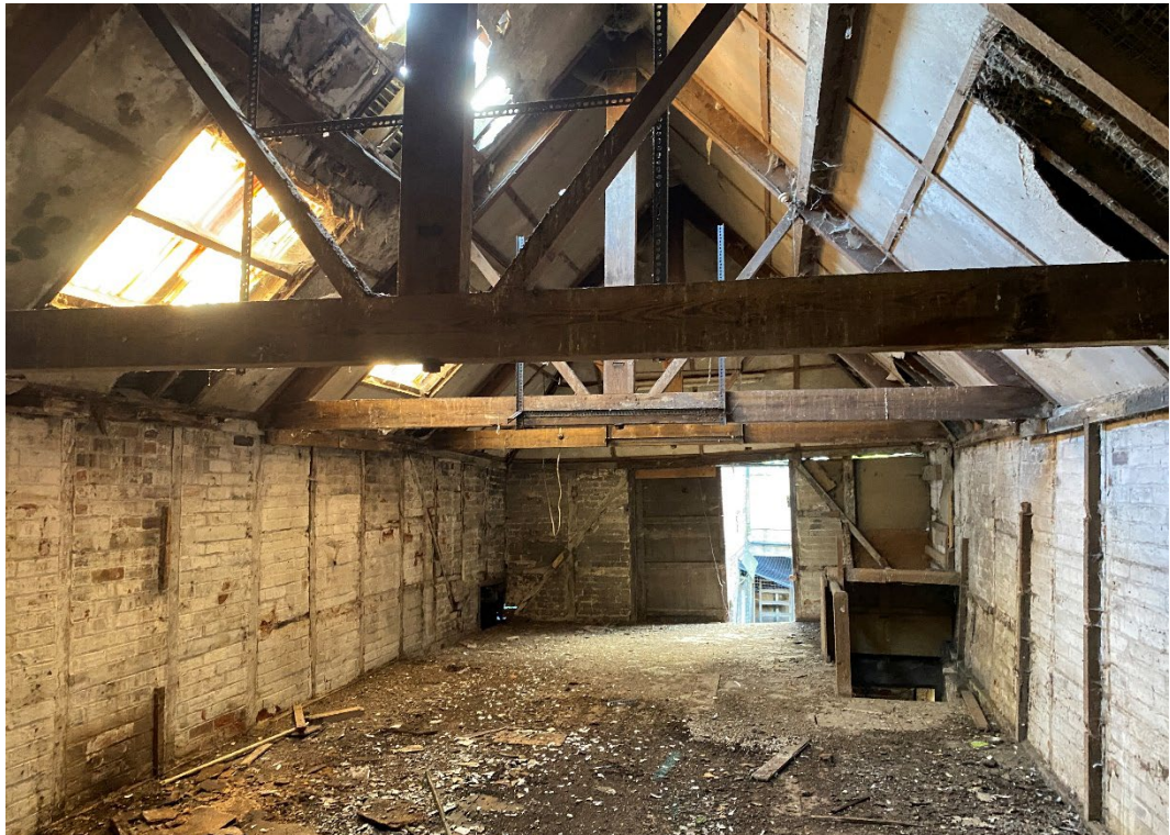
Figure 29: first floor area, a single space with 20 th century roof structure and covering, post 1916 fire.
