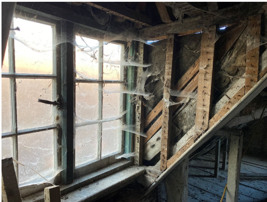
Figure 39: Dormer in attic of oldest core, dormer frame may be 19 th century but window has been replaced in the 20 th .
