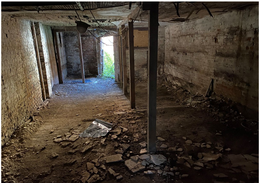
Figure 28: Ground floor space in the late 18 th early 19 th century store/stable.
