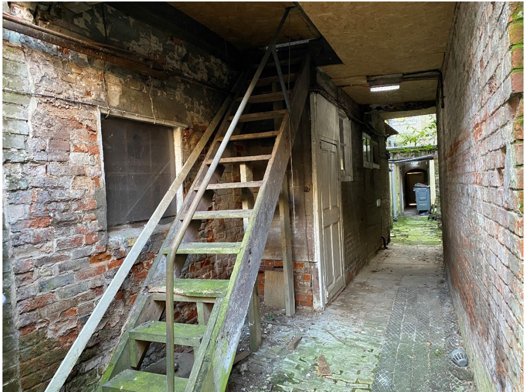
Figure 31: the side alley looking towards the market square.
