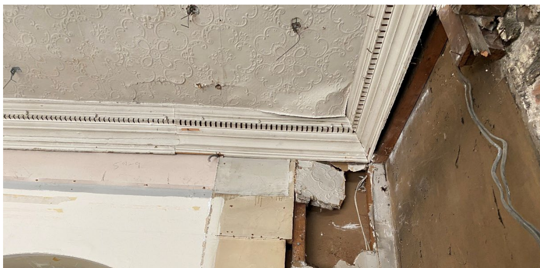
Figure 38: Embossed paper ceiling and small dentil cornice of timber profile in former retail space. Note inset alignment from brick wall on the right, and fragment of early sheet plaster board just in from the corner
