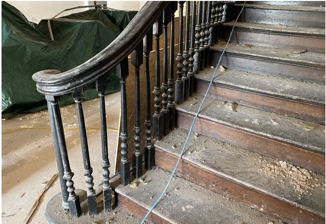
Figure 14: the main c.1740 stair with turned balusters three to a tread and curtail step.
