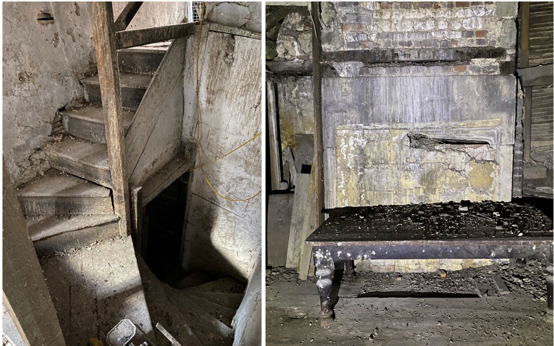
Figure 25-26: Newel stair from first to attic level; (right) stone fire surround with Tudor arched opening, blocked, in central area.
