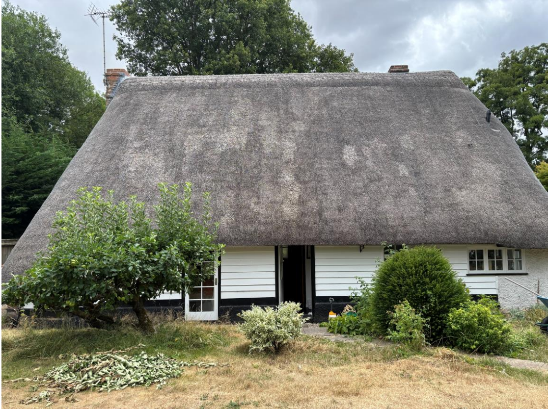
Fig.16 Rear wall of outshut – modern cladding, windows and doors
