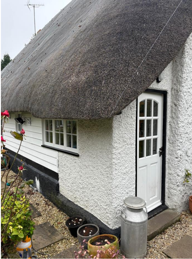
Fig.5 Modern half-glazed kitchen door on the SW gable
