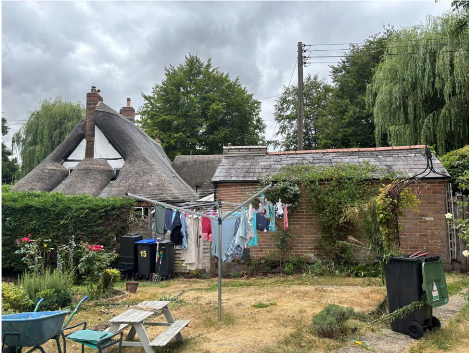
Fig.7 View looking west from the rear garden of Nine Mile Cottage to the neighbouring thatched cottage with extensions
