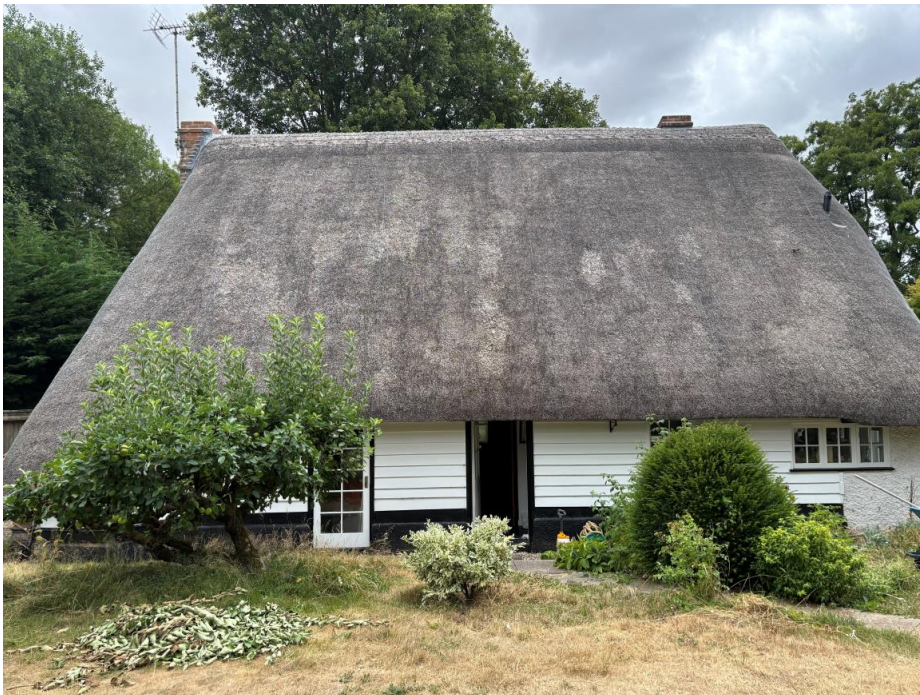
Fig.6 Rear elevation – outshut having modern weatherboard cladding and fenestration
