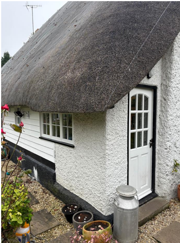
Fig.17 Modern half-glazed door on the SW elevation of the outshut proposed for removal
