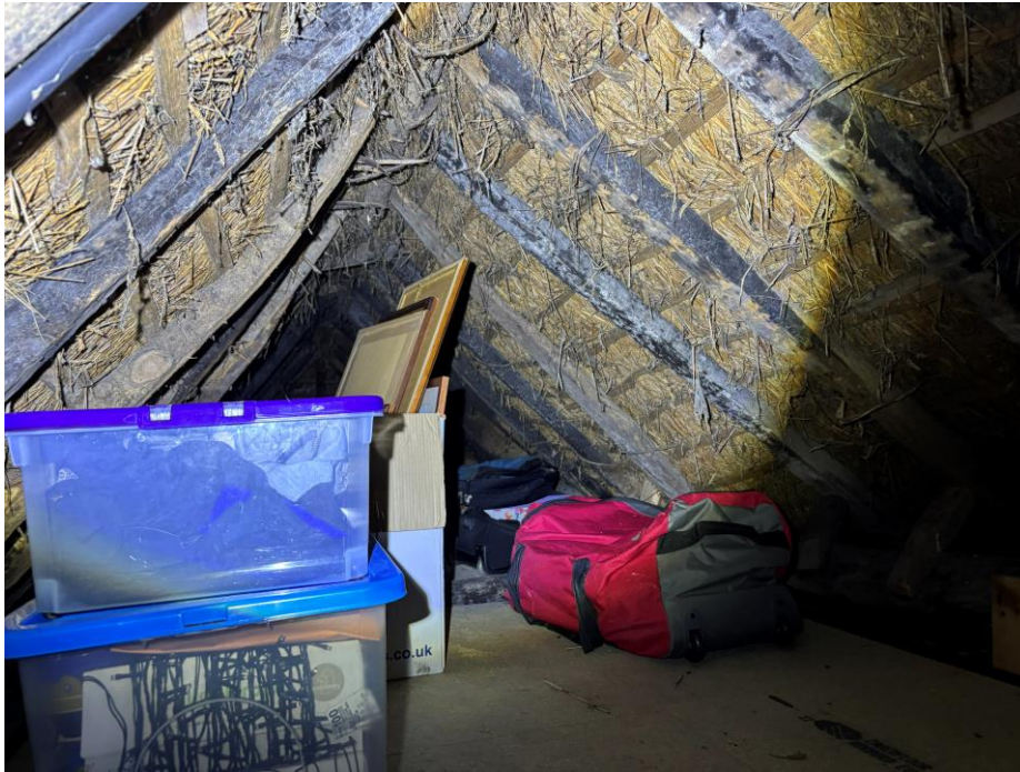
Fig.12 Loft area – historic, smoke-blackened rafters
