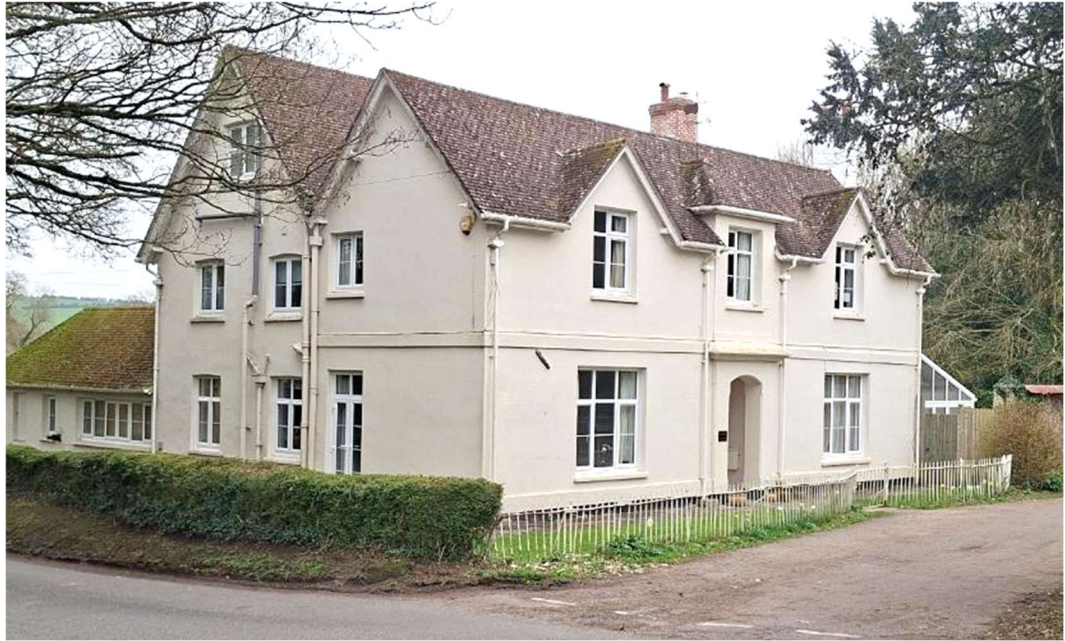
Figure 5 Ford House, front, west, and north elevations.
