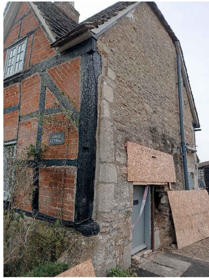
Photo 1: View of the door from the front drive (High Street)
