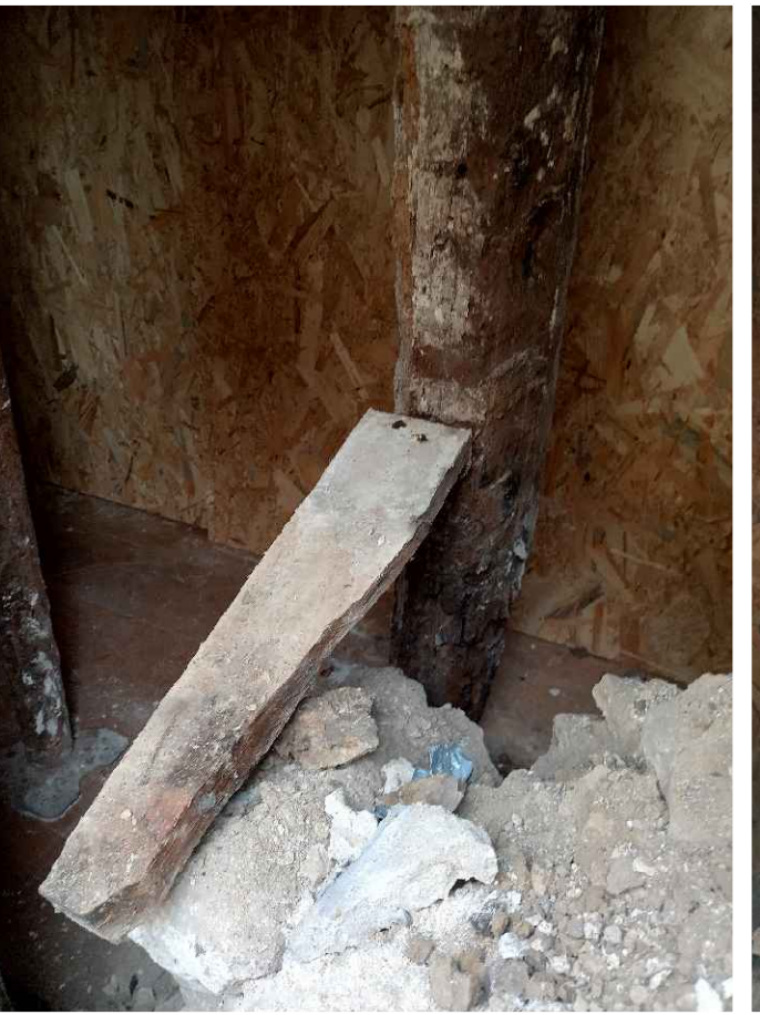
Photo 5: Photo showing timber wall ties
