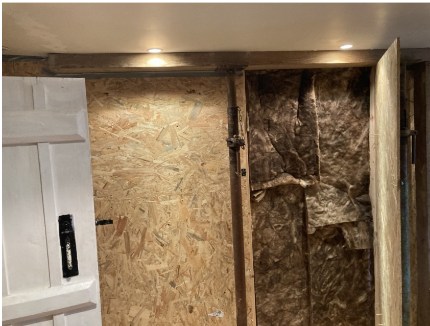
2. Temporary propping installed internally.
