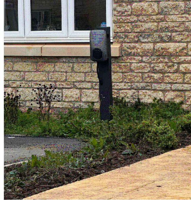
POLE MOUNTED VEHICLE CHARGING POINT
