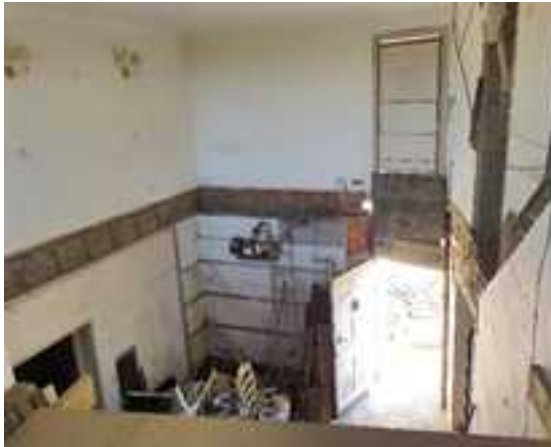
Figure 11: A view facing north from the second floor of the south-west section of the building showing the historic extension of the main building that has a flat roof
