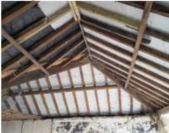
Figure 9: A view facing south of the existing dormer within the northern side of the interior roof valley along with the only extant section of ceiling under the southern roof ridge
