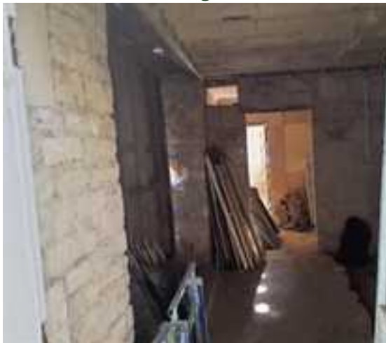
Figure 13: The interior space of the western single storey pitched roof section of the building
