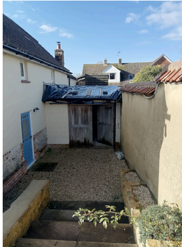
Existing front elevation of side garage
