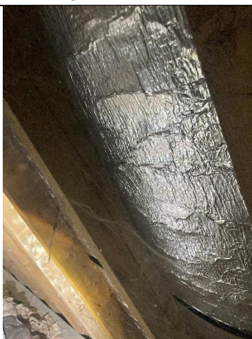
P11 Roof lining
