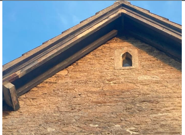
P4 Small gaps under barge boards/soffits on south-west elevation: area of works
