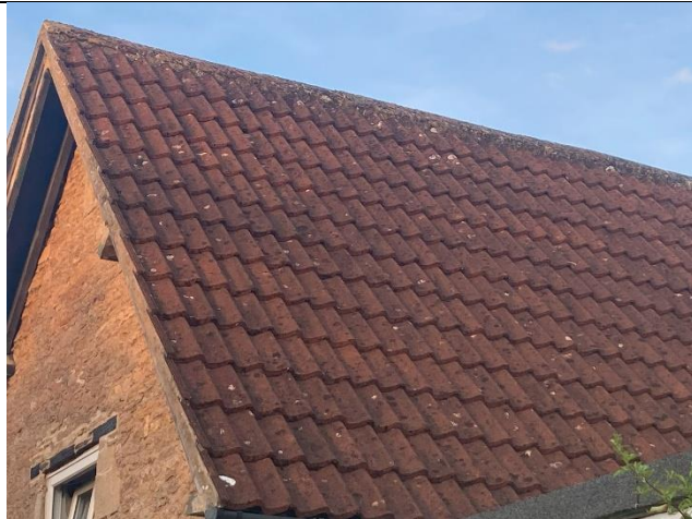
P5 Tiled roof adjacent to south-west elevation: no impacts
