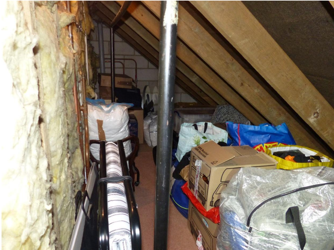
Figure 18 – First floor storage area
