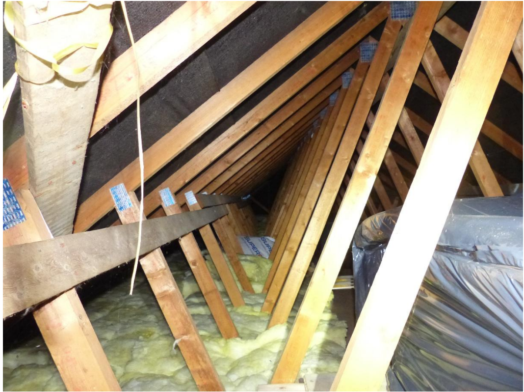
Figure 17 – Loft void viewed northwards from access hatch
