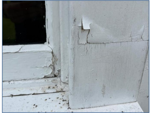
Sash box scarf repair
