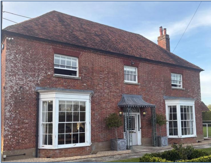
South Elevation showing bays and short sashes over
