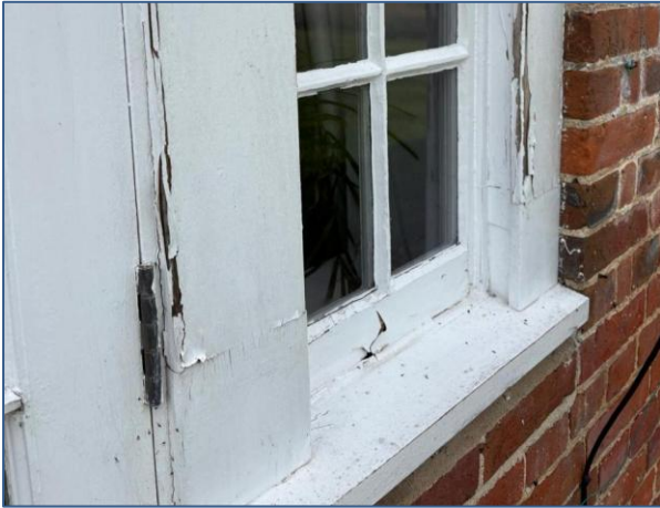
Sidelight sash repair
