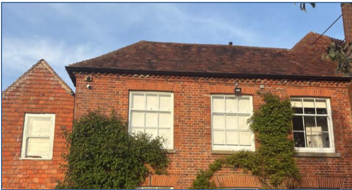
West Elevation first floor sashes in brick and tile hung elevations
