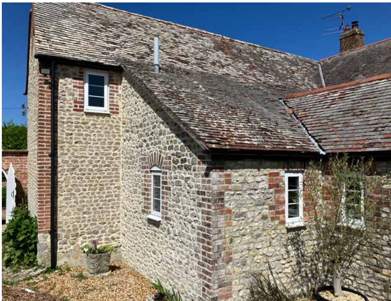
Existing The existing natural stone, brick quoins and clay plain tiles will be salvaged from this section of the building and set aside for reuse within the new extension.
