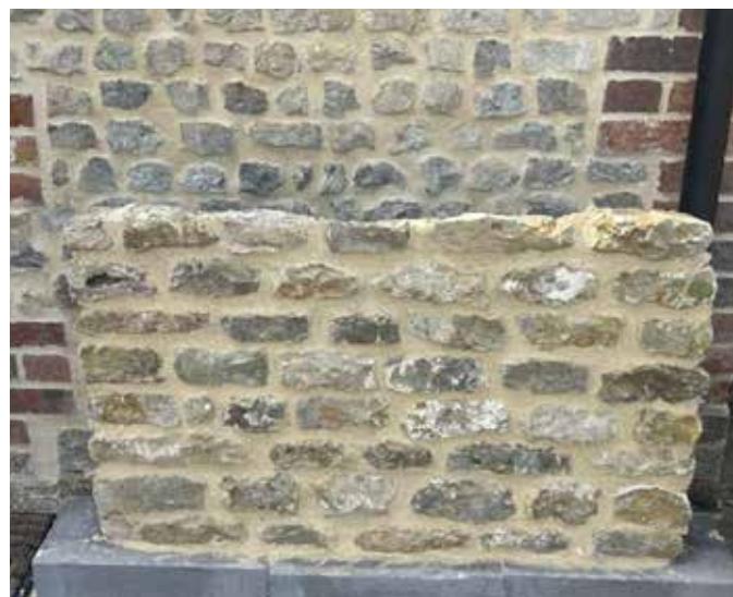
Proposed stone panel: 1 metre square panel of natural stonework to be used in the proposed extension for inspection and approval.
