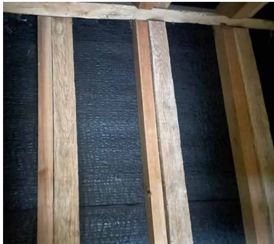
Existing The existing rear roof structure where the new roof to the first floor extension will be laid over
