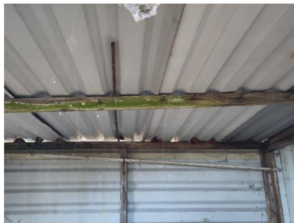
Figure 17 - Internal of building B1
