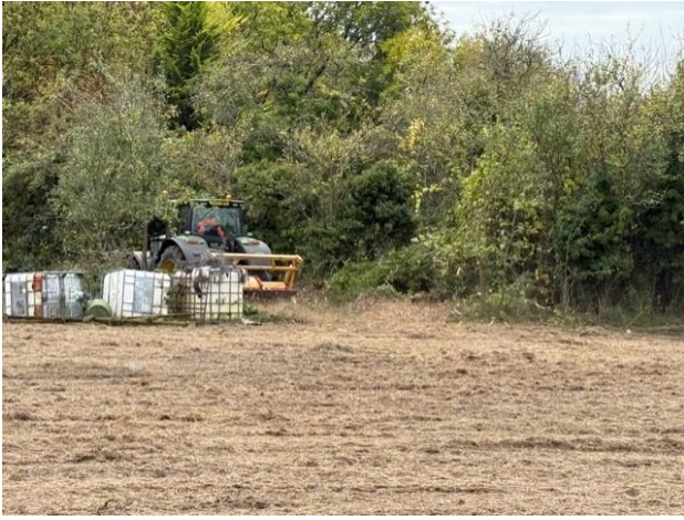
Figure 8 - cleared scrub and trees
