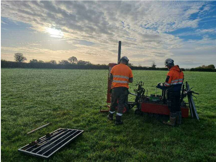
Photograph 23 – The location of borehole WS109.
