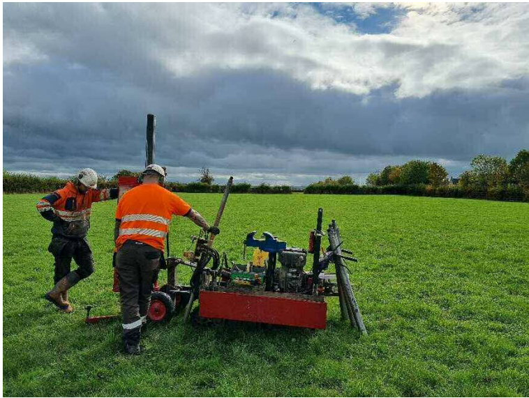
Photograph 17 – The location of borehole WS106.
