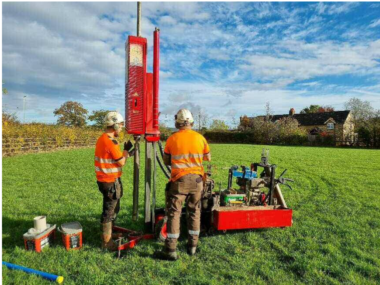
Photograph 25 – The location of borehole WS112.
