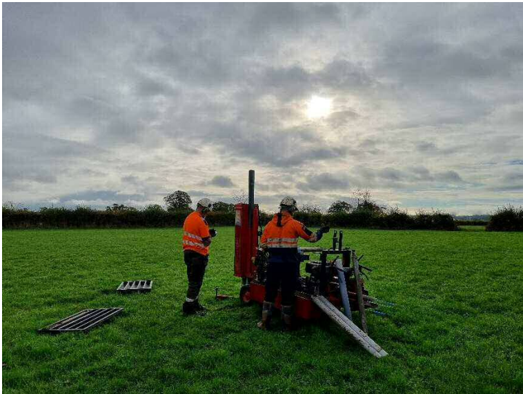
Photograph 5 – The location of borehole WS101.
