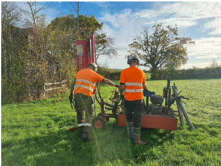
Photograph 25 – The location of borehole WS110.
