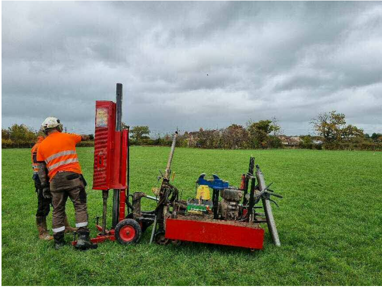
Photograph 15 – The location of borehole WS105.
