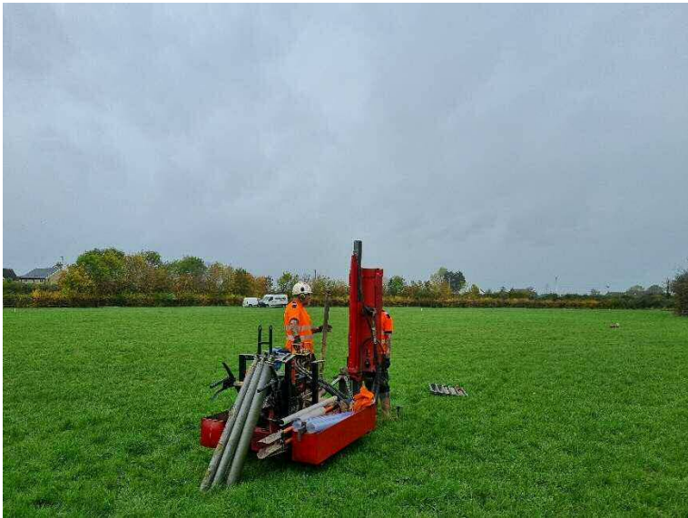
Photograph 9 – The location of borehole WS103.
