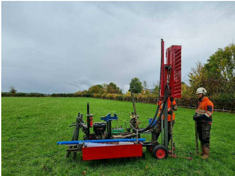
Photograph 21 – The location of borehole WS108.
