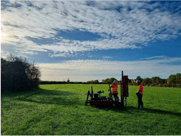
Photograph 23 – The location of borehole WS111.
