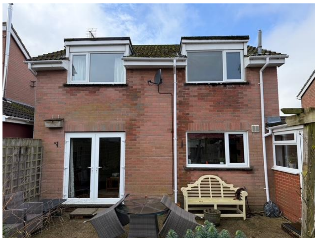
Figure 4 - Rear Elevation of no. 41
