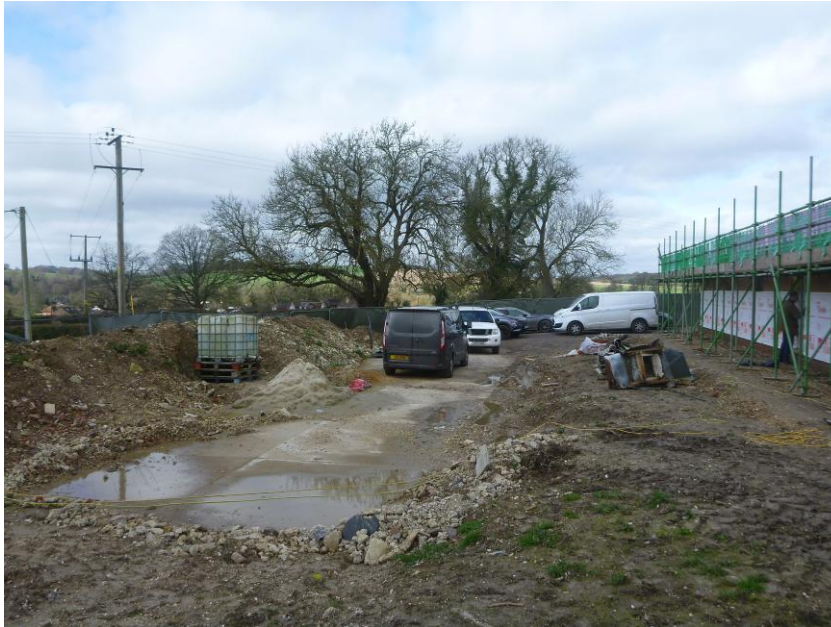
Fig 2: Within the site are two former chicken sheds, one which is being converted and the other has been demolished.
